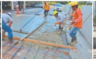
PARKING DECK & PT CABLE REPAIRS
