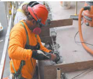
HIGH-RISE SPALL REPAIR
