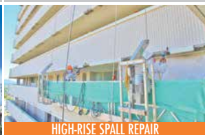
HIGH-RISE SPALL REPAIR
