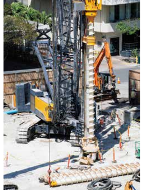
Kelikai's MC-128 at work on Hilton's new tower PHOTO COURTESY KELIKAI INC.
