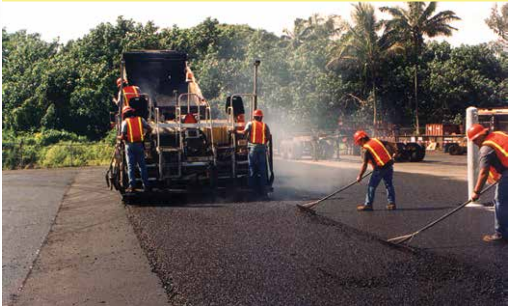
Laying asphalt
