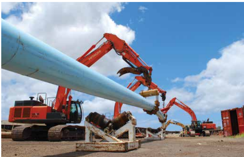
On Pearl Harbor's waterline project, Healy Tibbitts installed 24-inch fusible PVC below the channel bottom. PHOTO COURTESY HEALY TIBBITTS BUILDERS INC.
