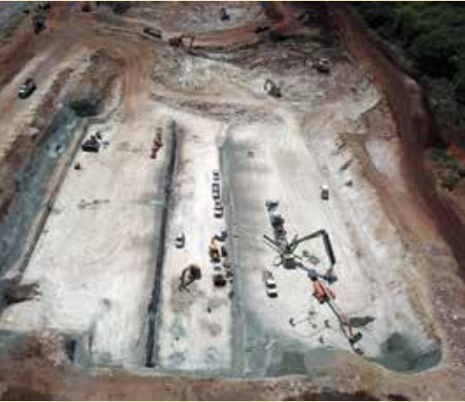
Mass excavation at Nan Inc.'s Honouliuli Wastewater Treatment Phase 1B project. PHOTO COURTESY NAN INC.
