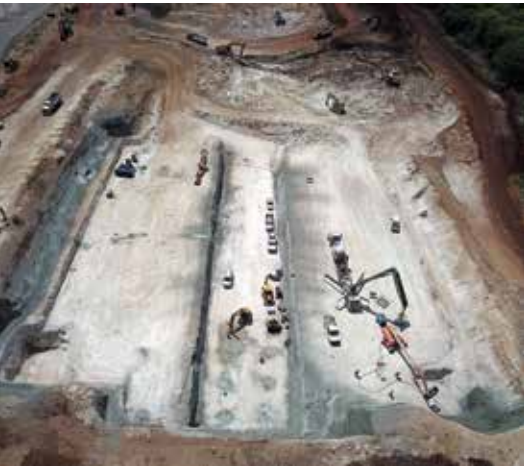
Mass excavation at Nan Inc.'s Honouliuli Wastewater Treatment Phase 1B project. PHOTO COURTESY NAN INC.
