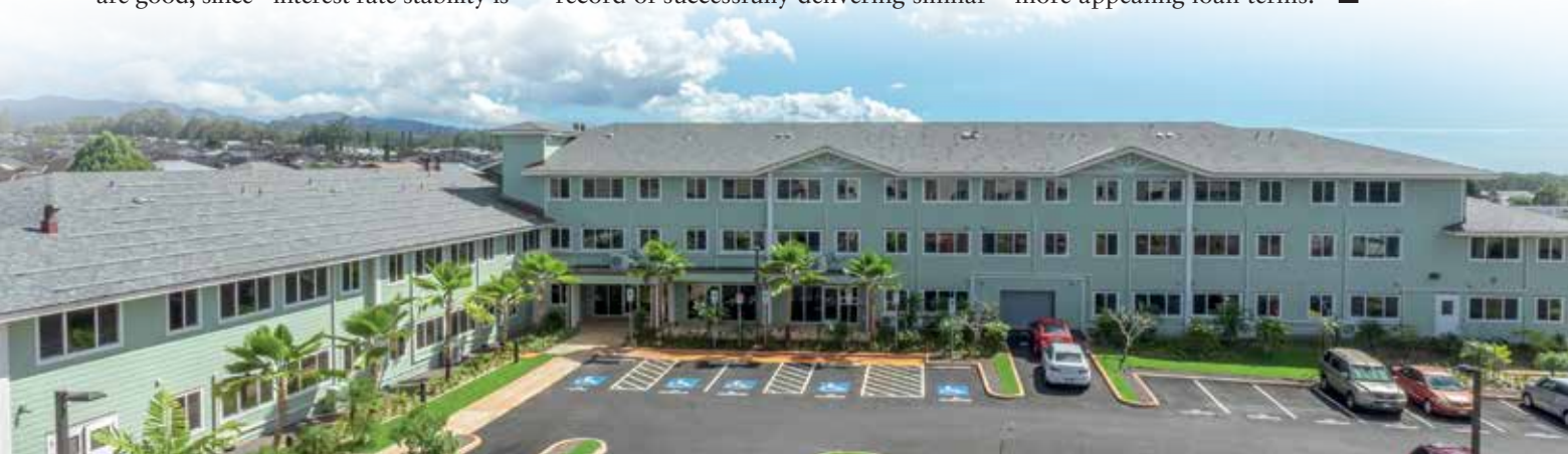
Meheula Vista (Phase III), a master-planned, low-income senior affordable rental housing development financed by Bank of Hawaii.
