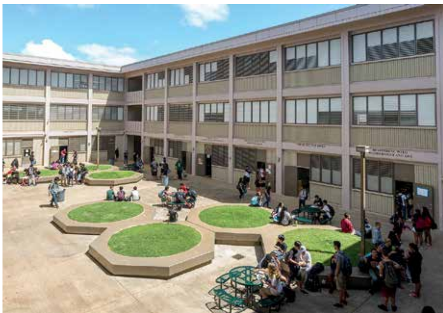
Swinerton is constructing five new classroom buildings at Campbell High School. PHOTO COURTESY SWINERTON BUILDERS
