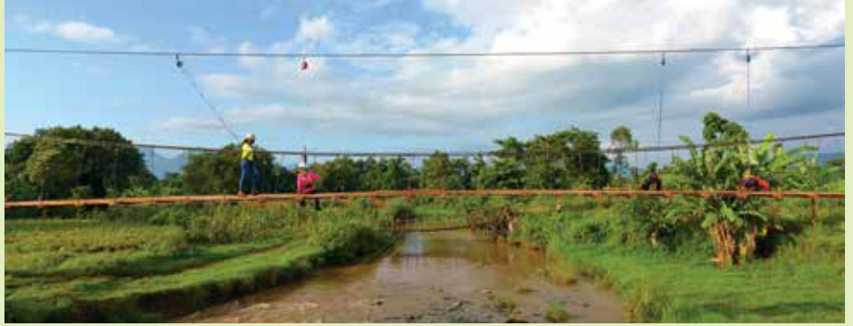
Nordic PCL's Women's Build team members on the 210-foot suspension bridge over the Sironko River. PHOTO COURTESY BRIDGES TO PROSPERITY
