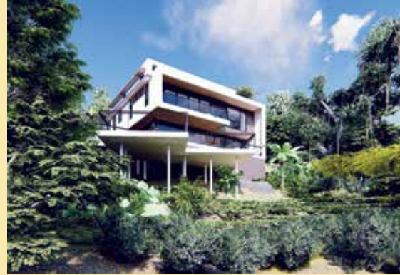
This luxury home is being built on a 70-foot drop. RENDERING COURTESY ROLI POLI STUDIOS LLC
