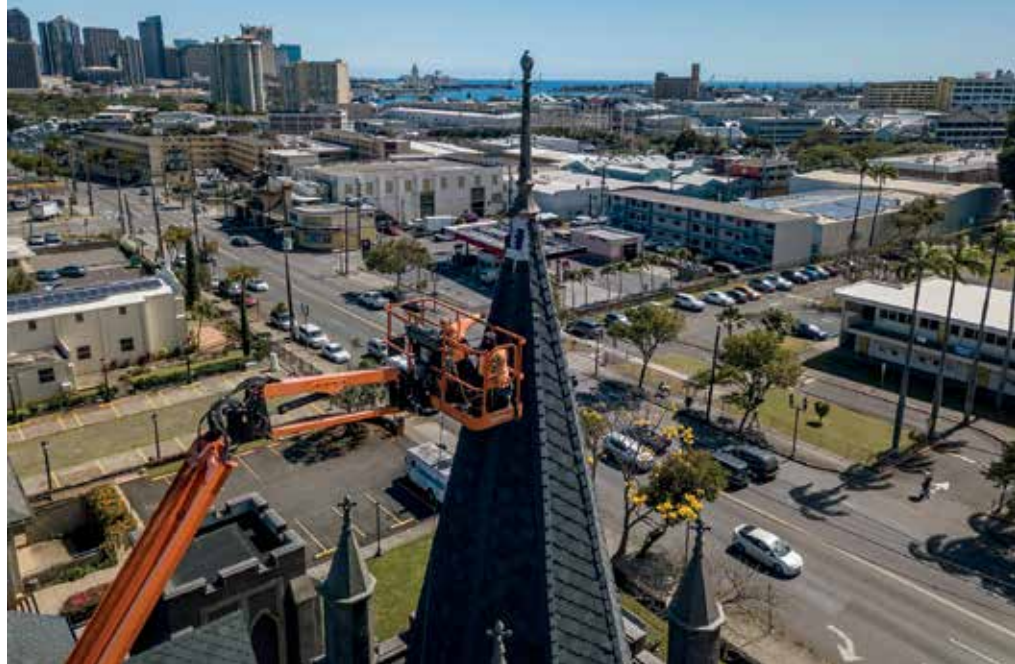
High winds were part of a steeple re-roof with GAF shingles by Surface Shield.
