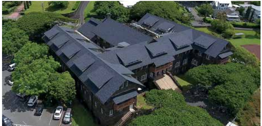
Mid-Pacific Institute, roofed with Malarkey’s Legacy 50-year modified shingle with Scotchgard Algae Block PHOTO COURTESY MALARKEY ROOFING PRODUCTS
