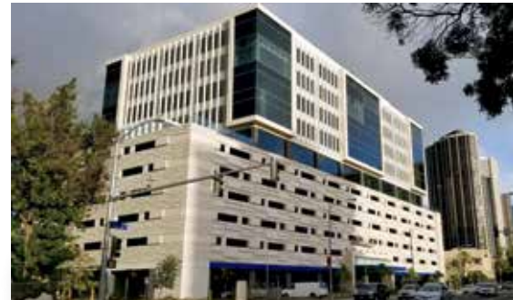
A-1 A-LECTRICIAN projects last year included the American Savings Bank campus.
