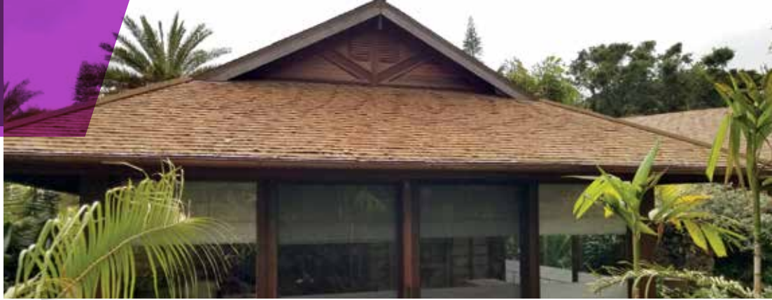
Beachside installed the roof for the Koele Lodge expansion project.
