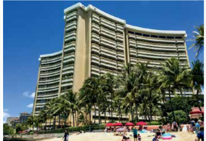
Zelinsky Company is currently painting the exterior of the Sheraton Waikiki.
