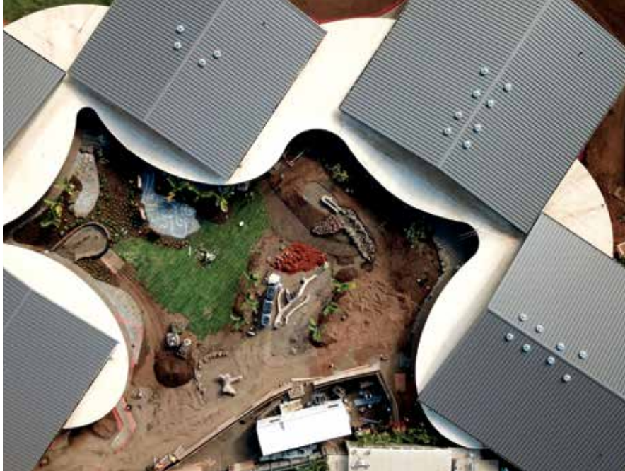
Beachside used Computer Assisted Design (CAD) to spec the single ply TPO roofing pre-ordered from Firestone. PHOTO COURTESY BEACHSIDE ROOFING LLC
