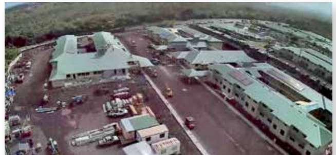
Coastal Construction's workload includes Mohouli Senior Living in Hilo.
