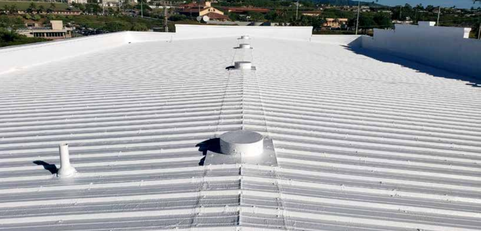
At the Maui News building, National Coatings restored multiple substrates including metal roofing, modified bitumen vertical walls and gutters. PHOTO COURTESY NATIONAL COATINGS CORP.
