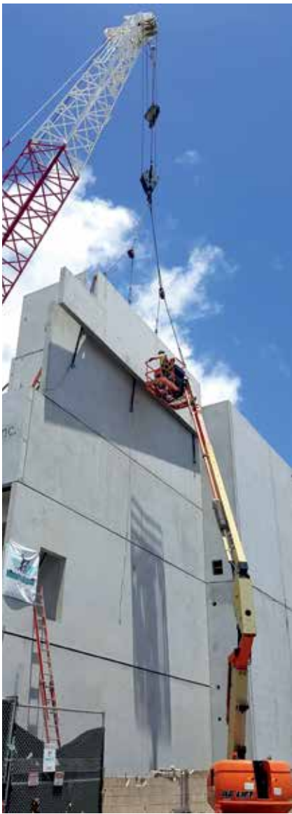
Commercial Plumbing's new three-story pre-cast office building and warehouse
