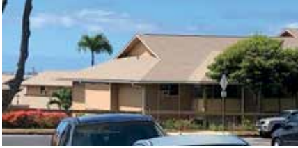
Tropical Roofing and Raingutters installed more than 200,000 square feet of Malarkey's NEX Highlander shingles in Energy Star-rated Golden Amber at Waiau Garden.
