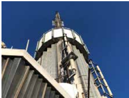
A temporary structural “cocoon” kept workers and the public safe during construction. | PHOTO COURTESY SKANSKA USA
