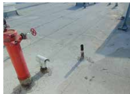
Built-up roof bubbling and deterioration
