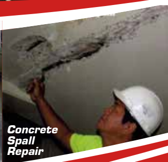
Concrete Spall Excavation
