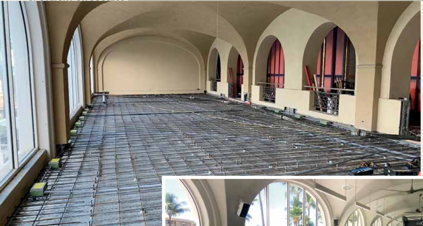
The fitness center's floor is readied for pouring concrete.
