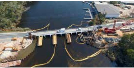
Halls River Road bridge PHOTO COURTESY FDOT
