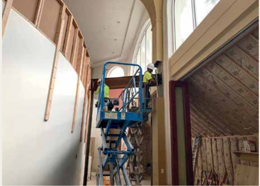
Workers secure the steel beams.
