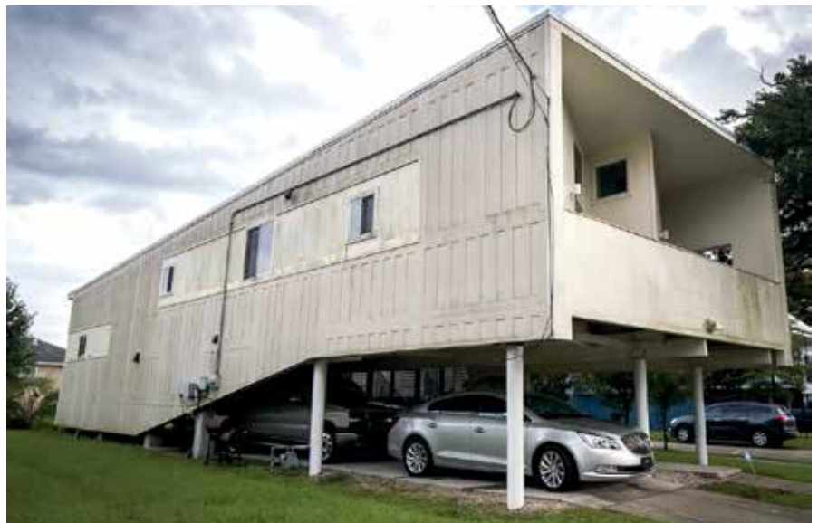
Mold covers the side of a Make It Right Foundation home in the Lower 9th Ward neighborhood in New Orleans.
