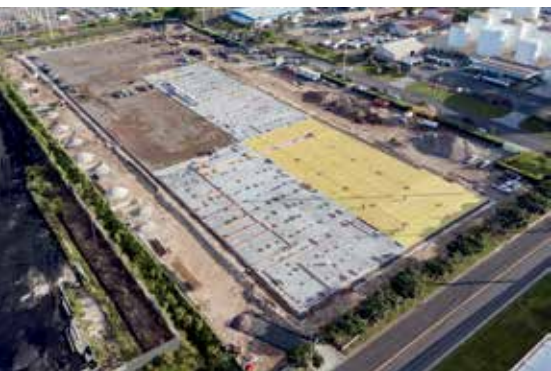
View of Honolulu Builders' Hanua Logistics Center jobsite, zones 1 through 4 with panel wall forms PHOTO COURTESY HDC PROPERTIES LLC
