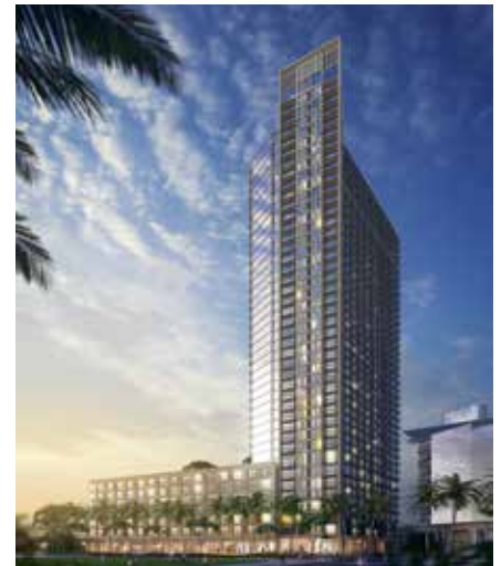
A’ali’i, a mixed-use/residential tower currently underway by Albert C. Kobayashi Inc. in Ward Village RENDERING COURTESY THE HOWARD HUGHES CORPORATION
