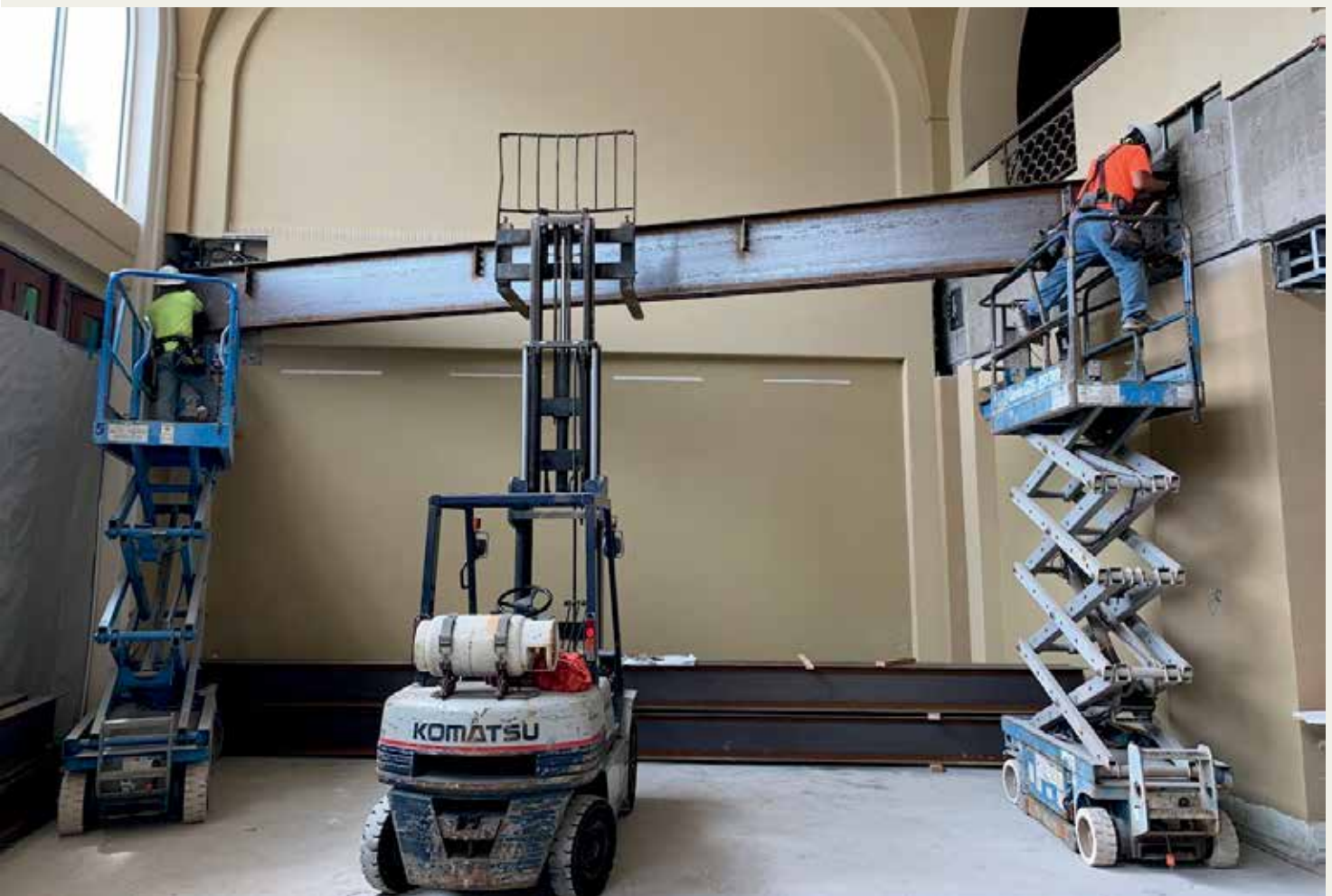
Workers install steel beams to support the floor of the fitness center at Fairmont Kea Lani.
