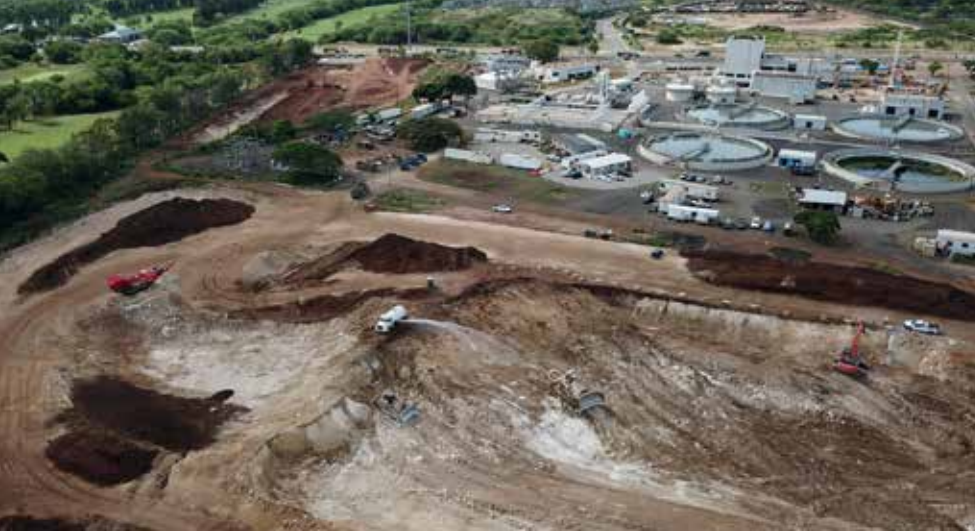
Nan Inc. is using GPS to work off of reference points in real time at the 24-acre Honouliuli Wastewater Treatment Plant project. PHOTO COURTESY NAN INC.
