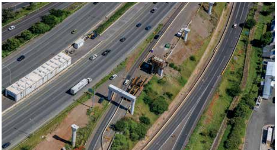
HART's guideway takes shape along eastbound H-1 near Airport Exit 16.
