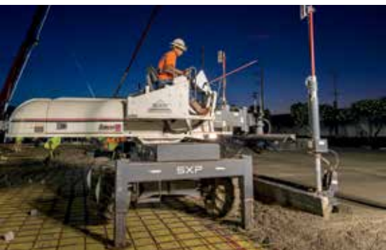
Laser screed by Honolulu Builders at the Hanua Logistics Center warehouse PHOTO COURTESY HDC PROPERTIES LLC
