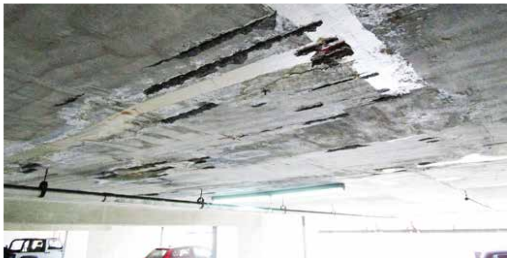
Water stains, efflorescence, corroded steel reinforcing, spalled concrete and previous repair attempts visible at the ceiling of a parking garage located below a recreation deck
