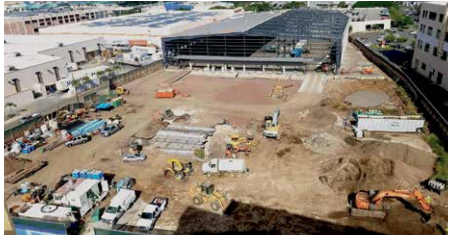
DHX's new storage facility PHOTO COURTESY DHX
