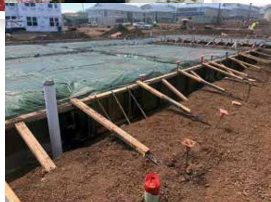
Koa'e Workforce Housing, a current Shioi project, will provide 134 units, 23 buildings and a community center. PHOTO COURTESY SHIOI CONSTRUCTION INC.
