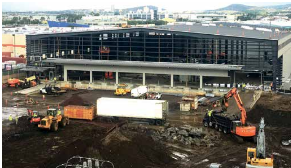
... the crew frames the warehouse.
