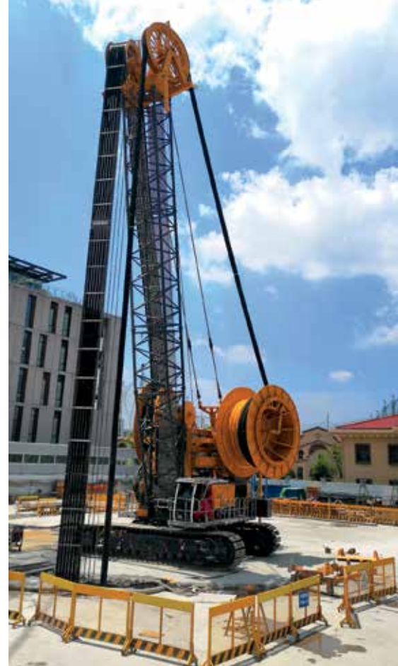
Bauer's 158-foot MC-128 crane weighs approximately 172 tons.
