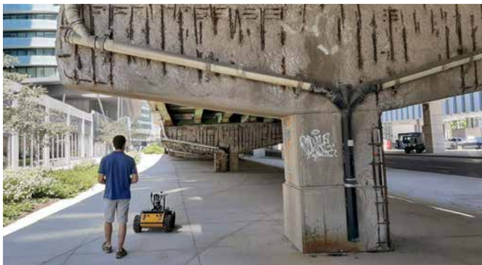
A University of Waterloo robot inspects the Gardiner Expressway in Toronto in July. PHOTO COURTESY CLEARPATH ROBOTIC
