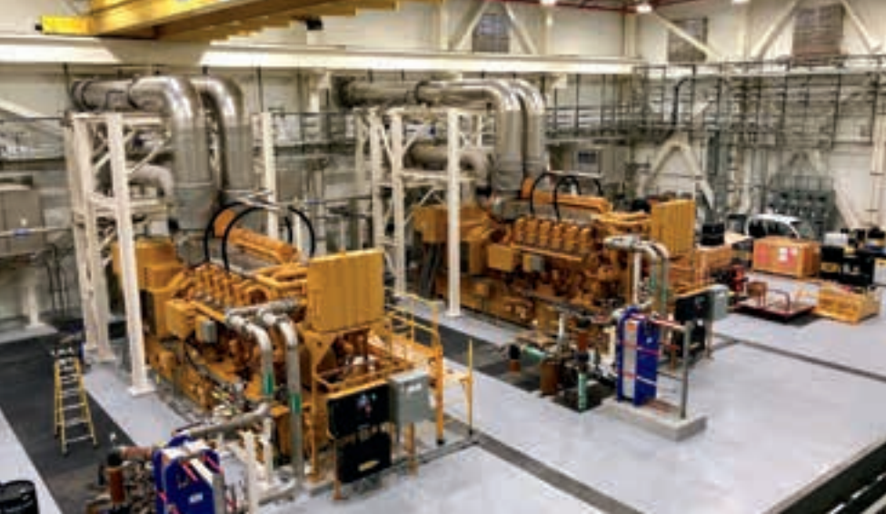
Nan Inc. will overhaul a generator (left) at the Power Plant Annex on Kwajalein, RMI. PHOTO COURTESY NAN INC.
