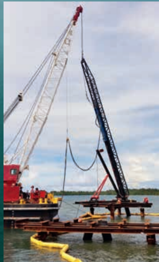
Installing piling at the wharf
