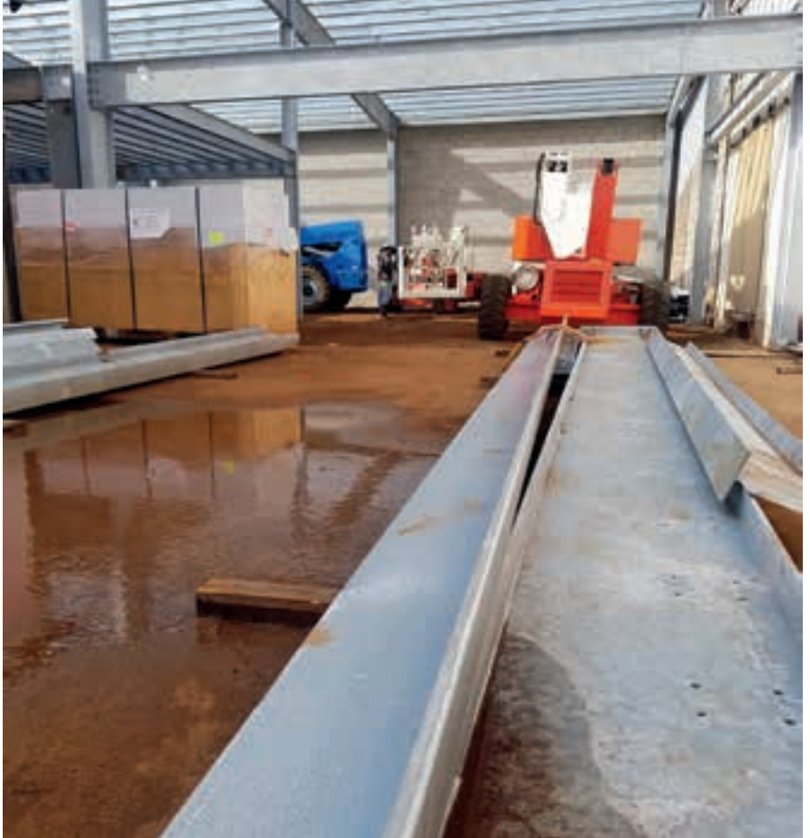
Schurch Construction is expanding the Kauai Beer Company in Lihue. PHOTO COURTESY SCHURCH CONSTRUCTION CORP.
