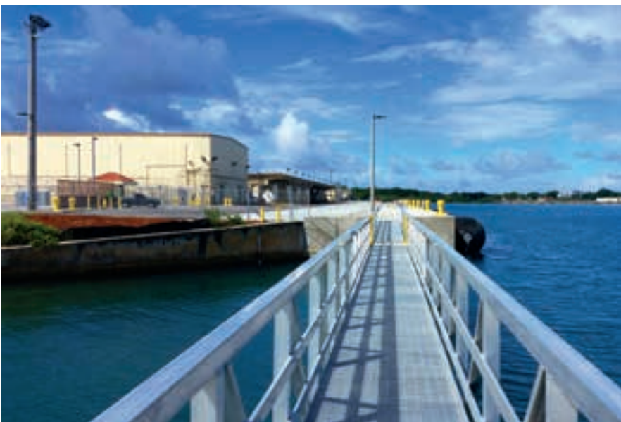
The multimillion X-Ray Wharf upgrade project at Apra Harbor on Naval Base Guam was named one of the most substantial contracts of 2018 by the Associated General Contractors of America. PHOTO COURTESY AGC
