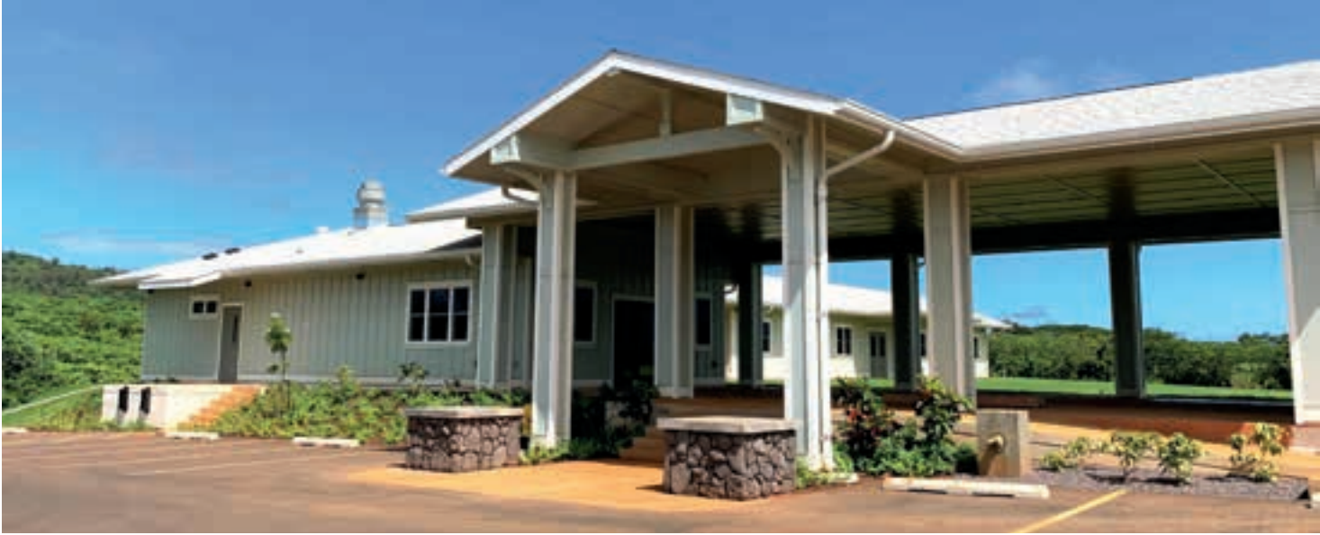
Layton Construction is wrapping up work on the Adolescent Treatment and Healing Center in Lihue. PHOTO COURTESY LAYTON CONSTRUCTION CO. LLC
