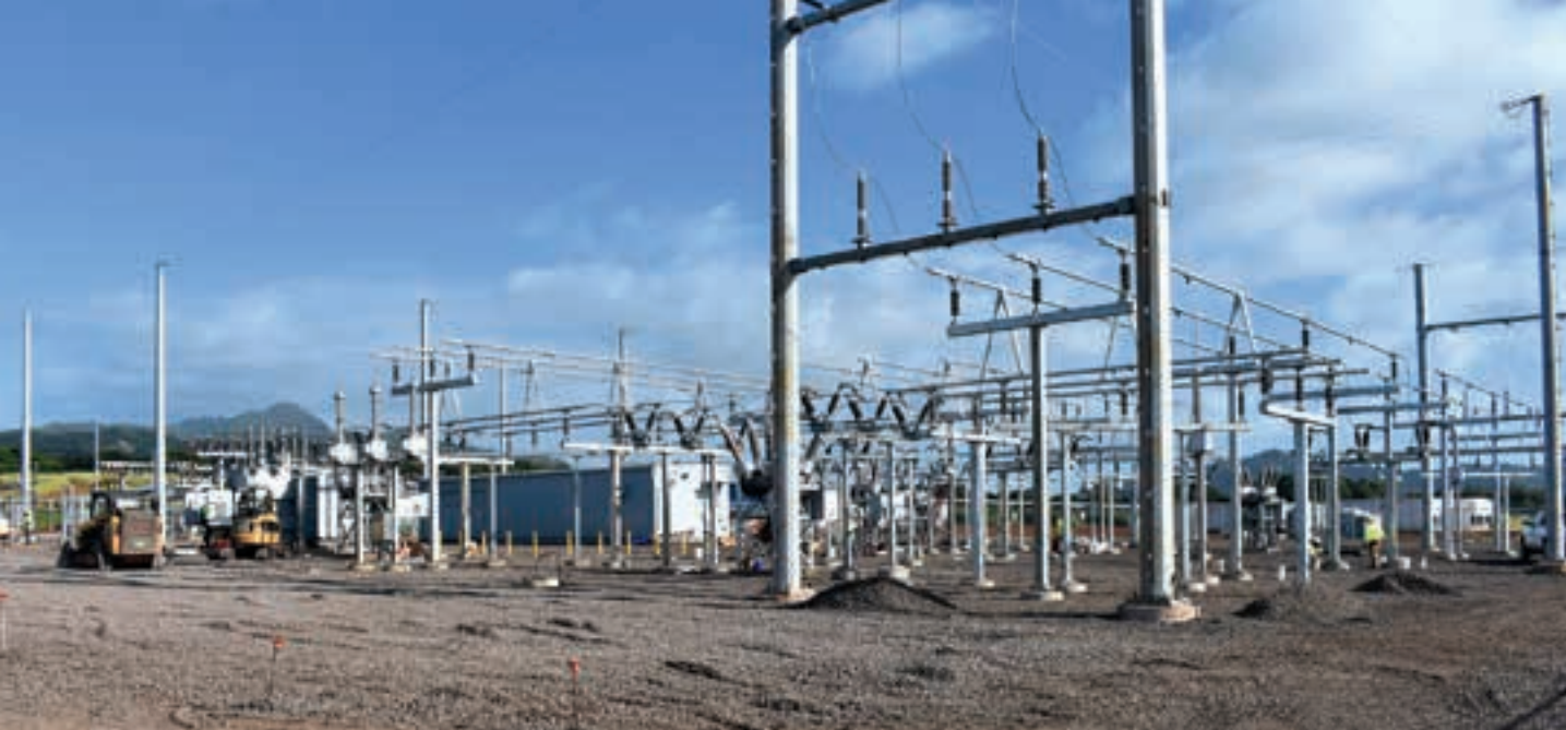
Tomco Corp. has built two substations in Lawai to help integrate power from the solar facilities into the grid. PHOTO COURTESY TOMCO CORP.
