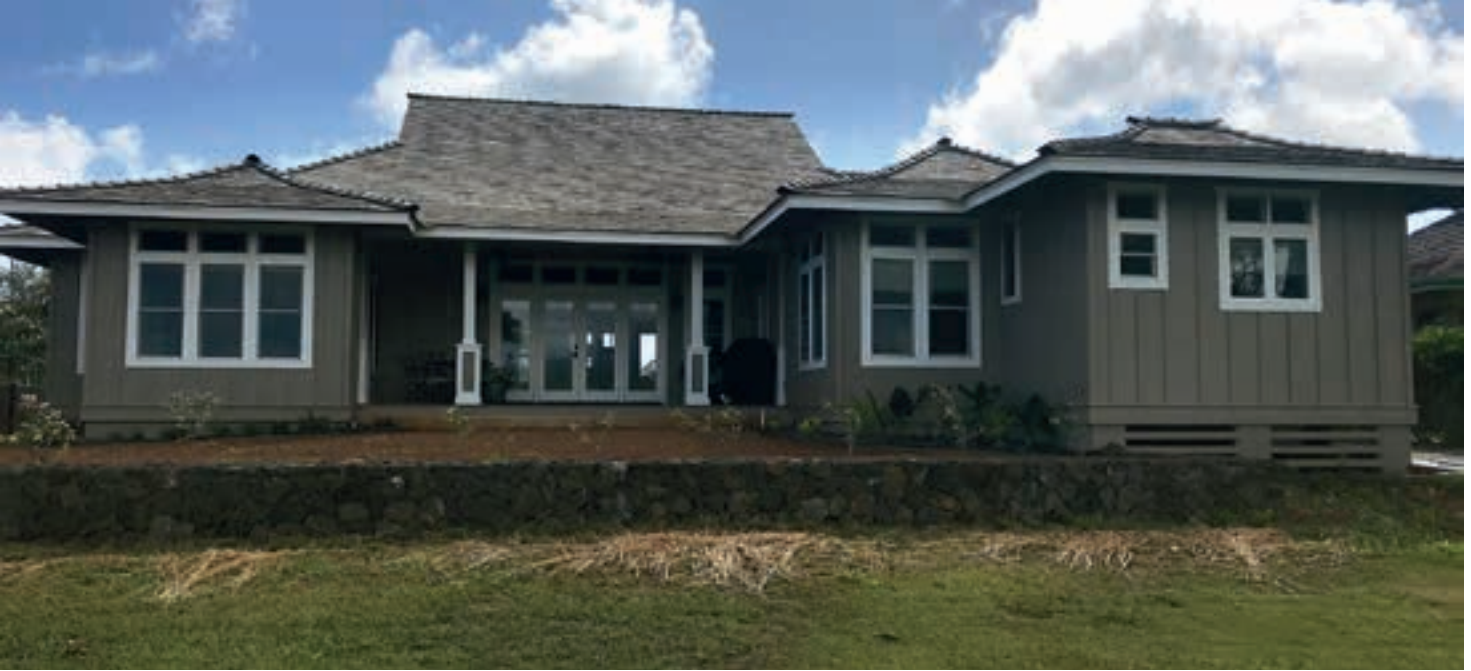
Appleby Construction puts the finishing touches on a residence in Poipu. PHOTO COURTESY APPLEBY CONSTRUCTION
