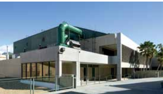
Layton's renovation of the University of Hawaii at Manoa gym won a GCA of Hawaii 2019 Build Hawaii Award of Excellence.
