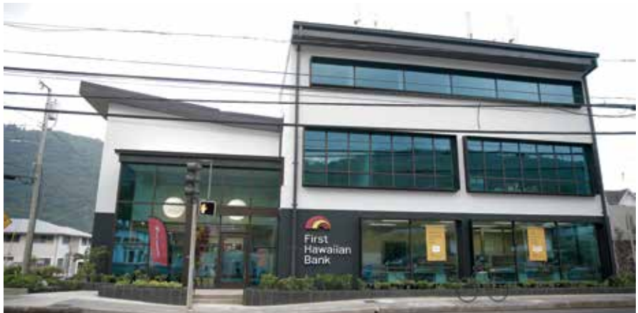
Ralph S. Inouye Co. Ltd. completed work on First Hawaiian Bank's Manoa branch.
