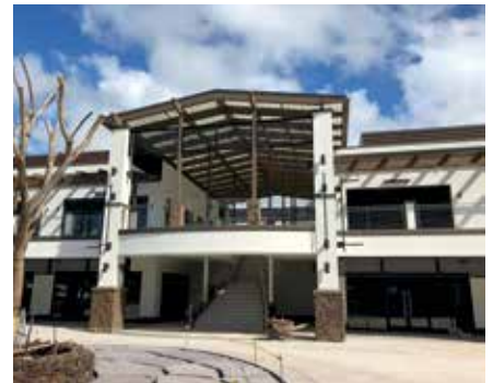
Maryl Group completed work last year on the 22,000-square-foot Wailea Village Center.
