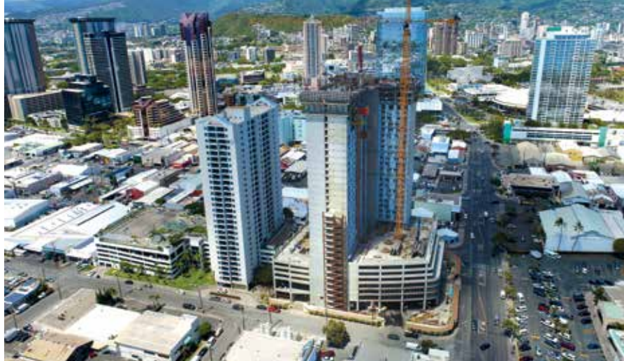
Ke Kilohana wrapped one month ahead of schedule. PHOTO COURTESY NORDIC PCL CONSTRUCTION INC.
