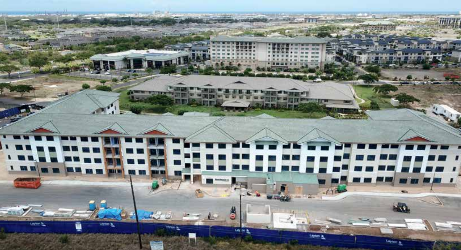
Marriott Residence Inn Kapolei construction site PHOTO COURTESY LAYTON CONSTRUCTION CO. LLC
