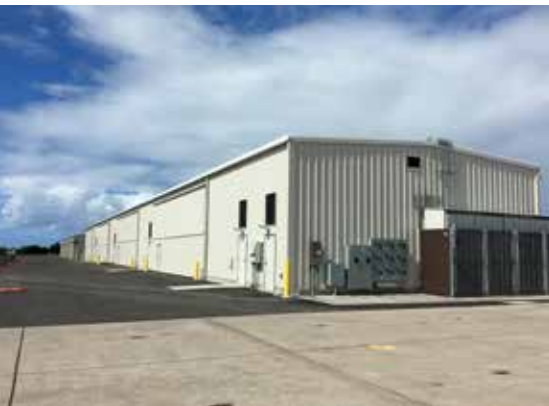
Elite Pacific jobs last year include the new T-hangar and infrastructure improvements Phase I at Kalaeloa Airport
