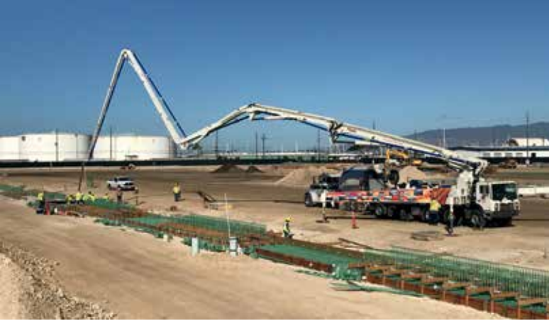
Kiewit works on Phase I of the Kapalama Container Terminal PHOTO COURTESY KIEWIT INFRASTRUCTURE WEST CO.
