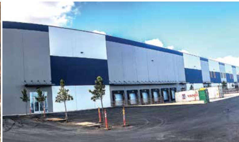
NEW WAREHOUSE SHELL BUILDING, LOT 20
