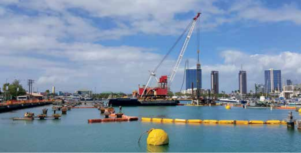
Healy Tibbitts installs concrete mooring piles designed to expand the harbor by 45 additional slips. PHOTO COURTESY HEALY TIBBITTS BUILDERS INC.
