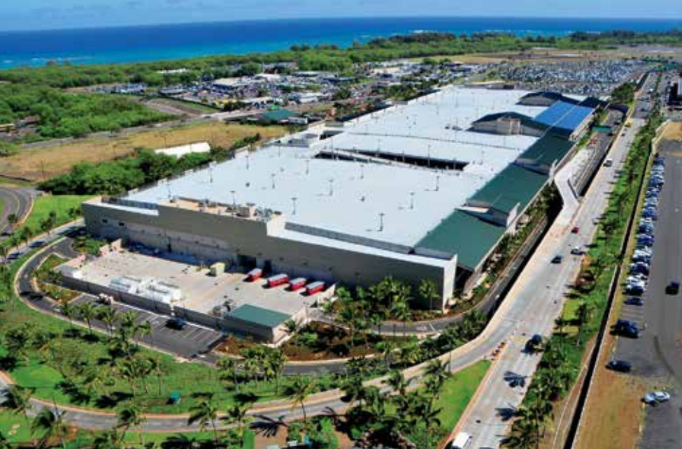
Aerial view of the new Consolidated Rent-A-Car facility at the Kahului Airport PHOTO COURTESY DOT
