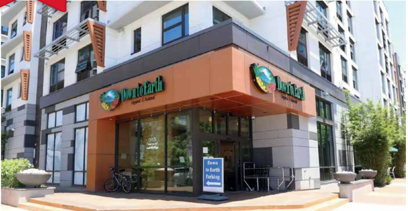
Honolulu Builders is working on its third Down To Earth store, like this one in Kakaako.
