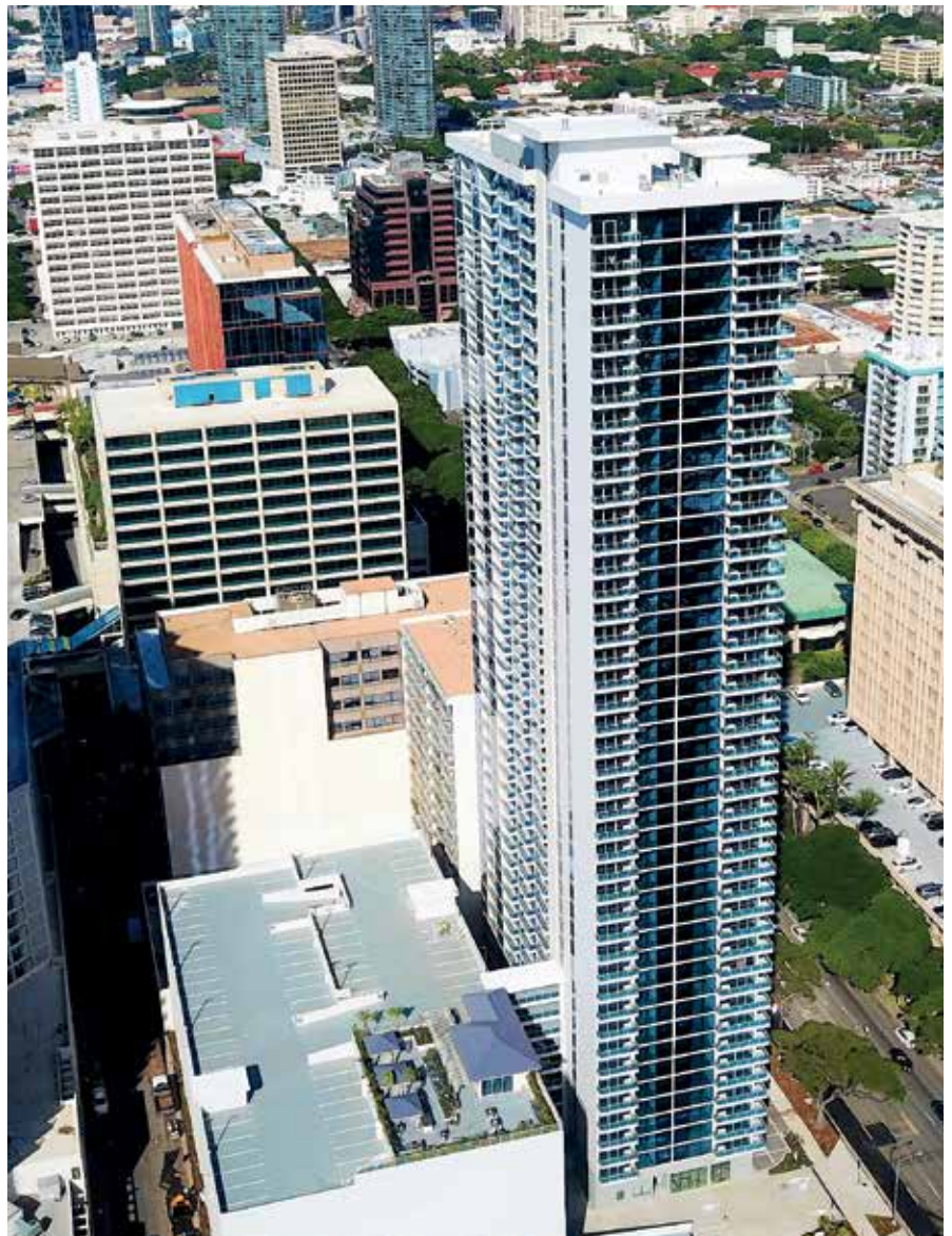
Hawaiian Dredging completed work on the Kapiolani Residence in 2018.
