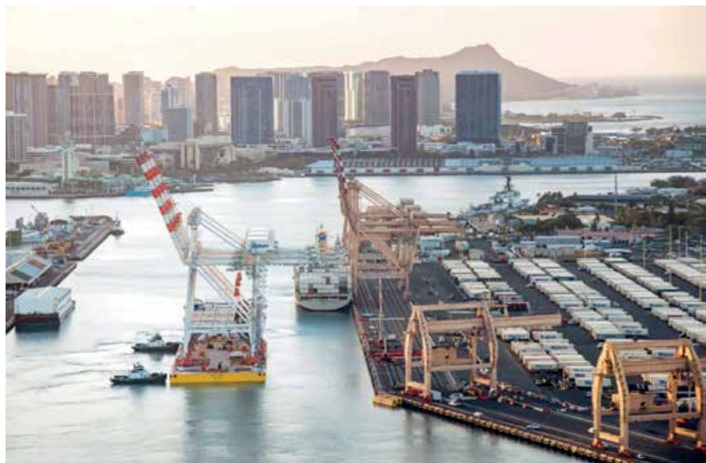
Matson’s gantry cranes and deployment of four ships by 2020 is part of a multi-year $60 million Sand Island Terminal expansion and modernization project. PHOTO COURTESY MATSON INC.
