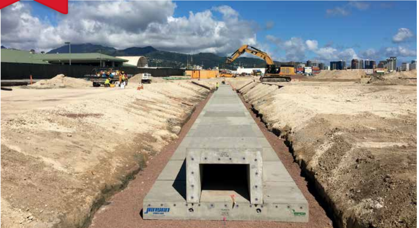
Kiewit is the general contractor on the new Kapalama Container Terminal cargo yard project at Honolulu Harbor.
