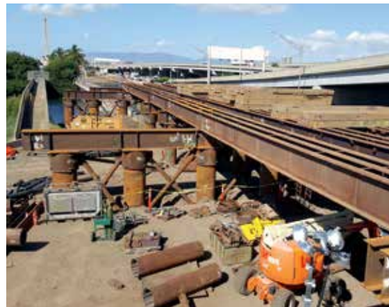
Pilings for the HART trestle project, located next to Nimitz Highway, are within a few feet of a gas line and an active sewer force main.
