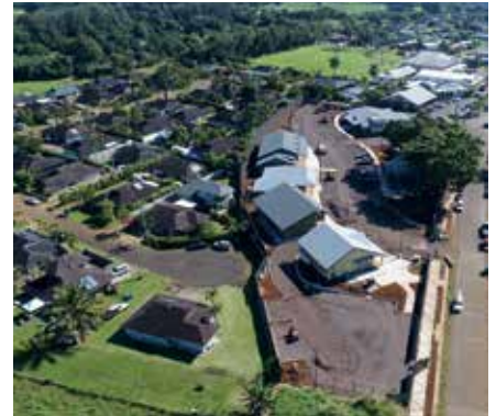
Shioi Construction has completed its work on the Kilauea Lighthouse Village project.
