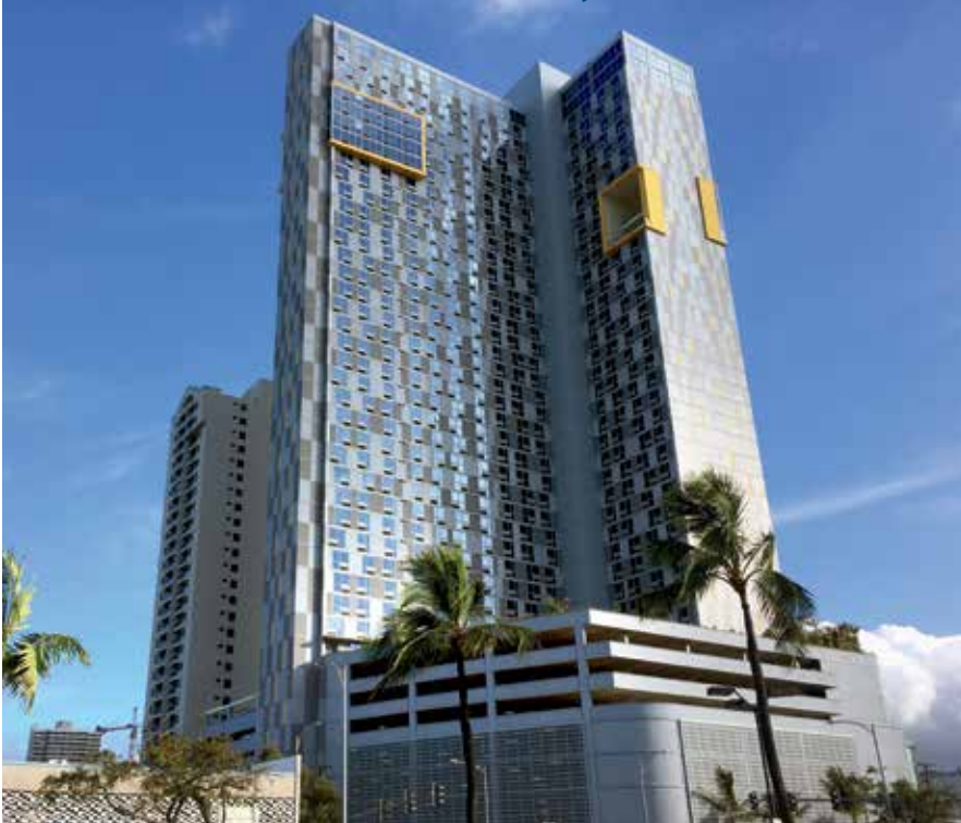
Most amenities are on Ke Kilohana's landscaped eighth floor. PHOTO COURTESY NORDIC PCL CONSTRUCTION INC.
