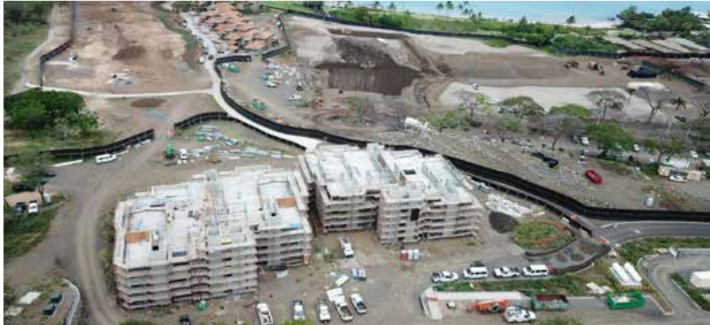
DDL is mechanical contractor on the redevelopment of Makena Kula Villas, which has an estimated value of $354.5 million.
