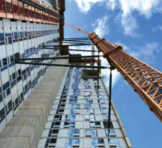
Nordic PCL completed one floor of 13,000-square-foot post-tension slab each week. PHOTO COURTESY NORDIC PCL CONSTRUCTION INC.
