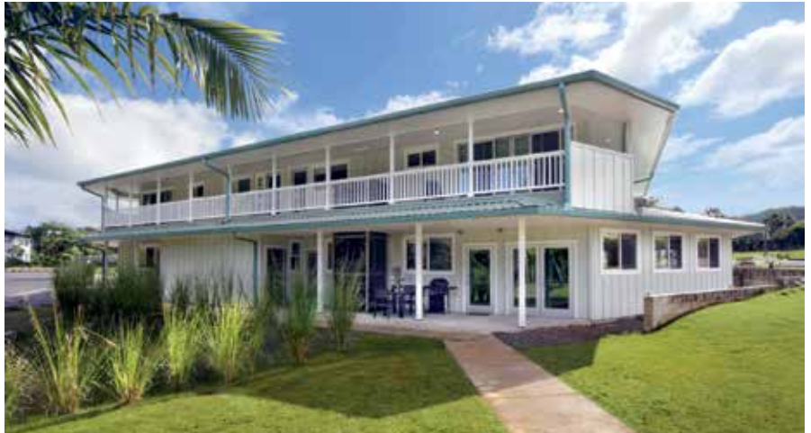
Layton finished the Makana North Shore Urgent Care Center one month ahead of schedule.
