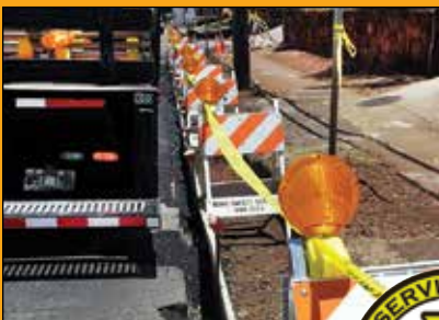
Temporary Traffic Control
