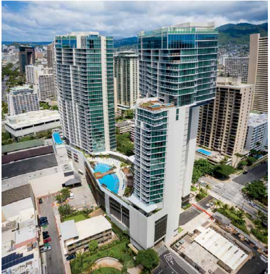
Albert C. Kobayashi Inc. garnered awards for its work at The Ritz-Carlton Residences, Waikiki Beach.
