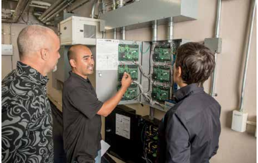
Installation of access control system at a major Hawaii data center
