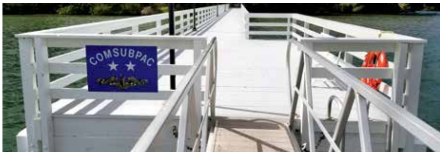
Among Alan Shintani Inc.'s projects last year was the boat landing at Joint Base Pearl Harbor-Hickam.
