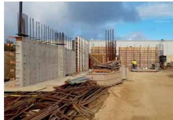
Hawaiian Dredging is currently installing CMU block, CIP walls and utilities at the MCBH communications/electronics facility.
