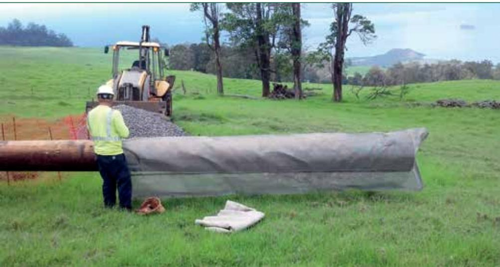
A utility pole is being prepared to go into the ground wearing a Polesock.
