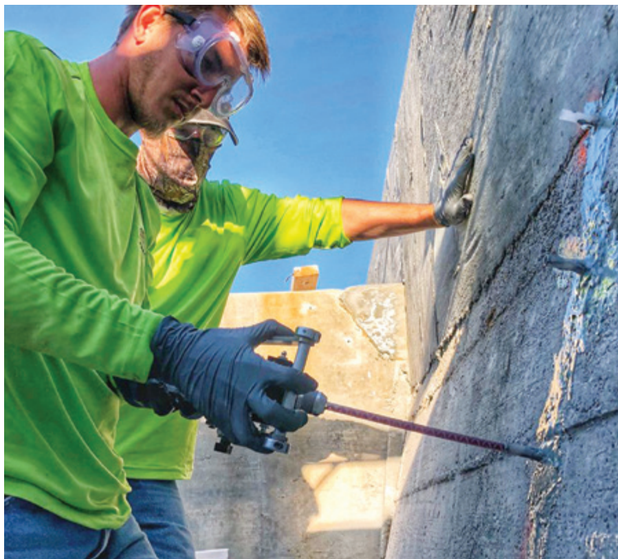
Repairing a seawall or bulkhead with polyurethane grouts will fill voids, stabilize loose soil and seal leaks at a fraction of the cost of wall replacement
