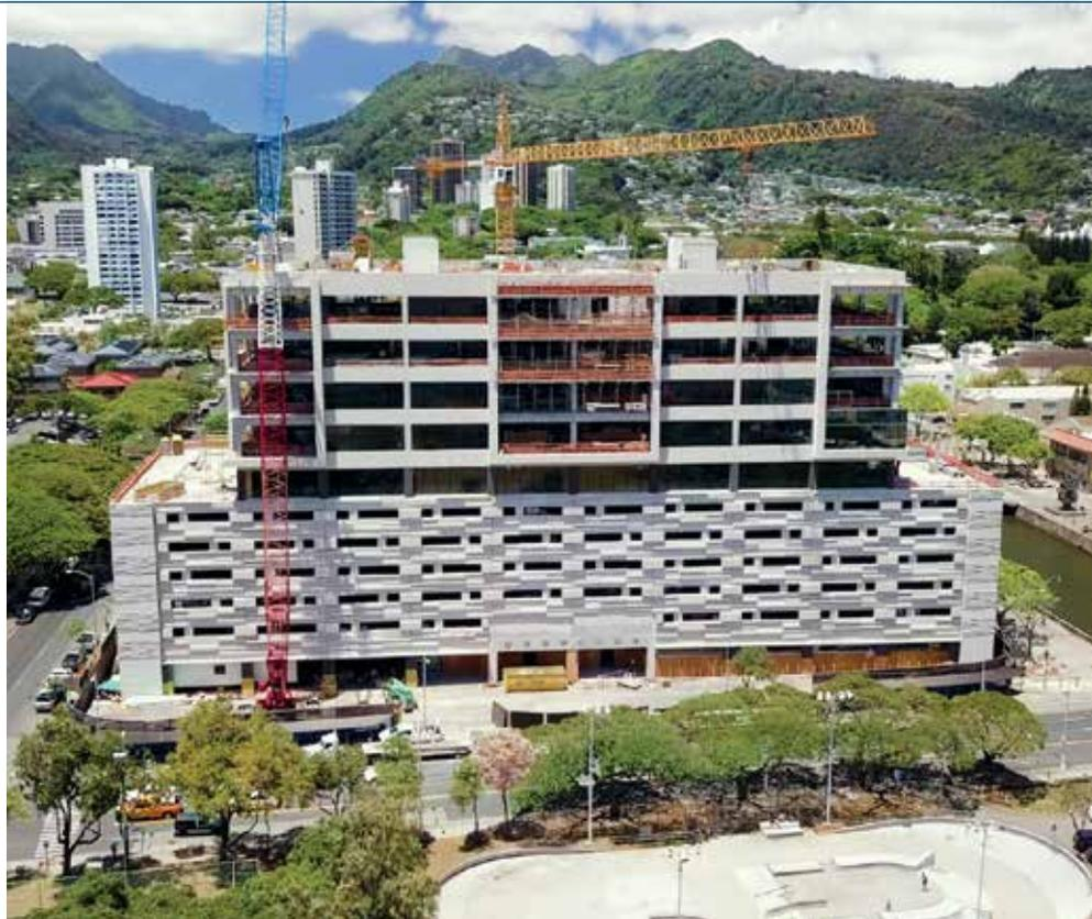
Cranes lift precast concrete into place on the American Savings Bank building.
