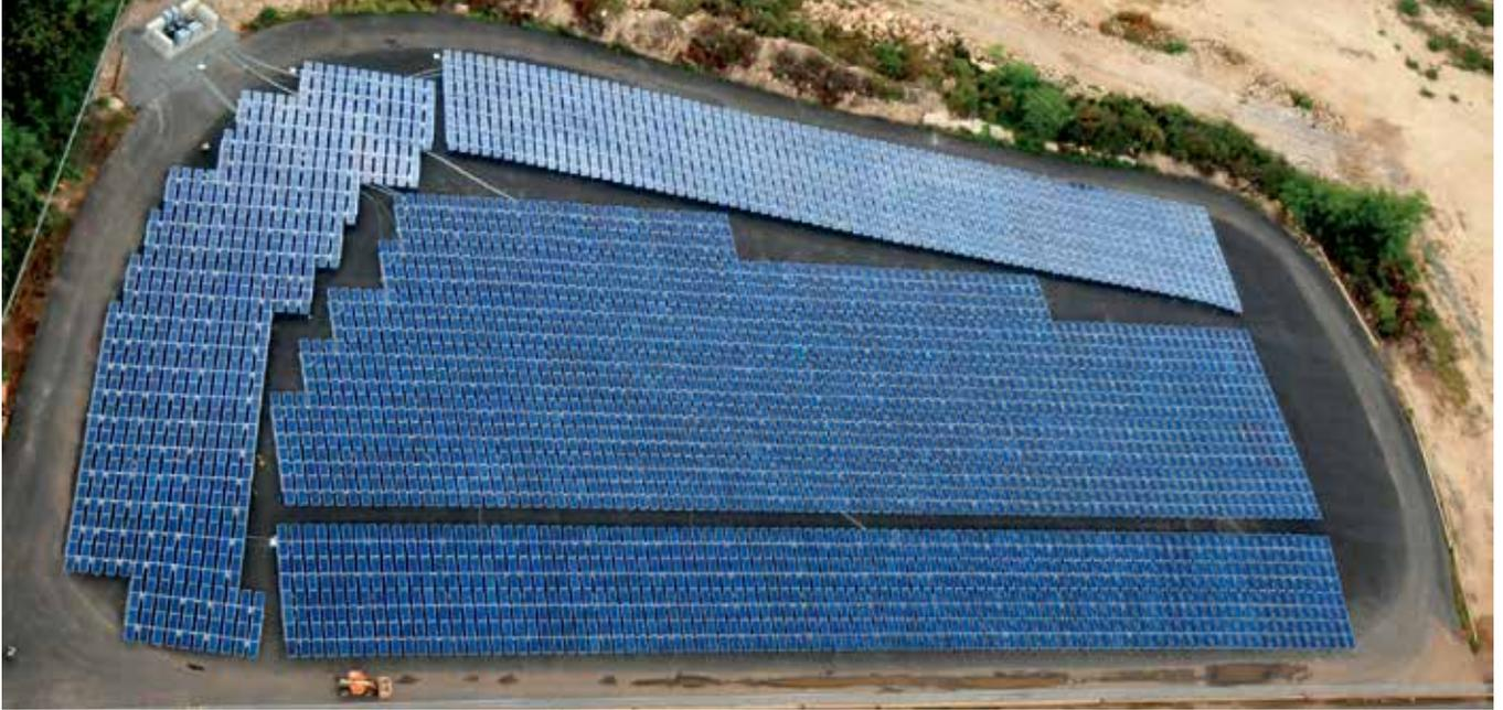
Kapolei Sustainable Energy Park was built over a remediated and capped waste pile formerly used to dispose of steel byproduct.
