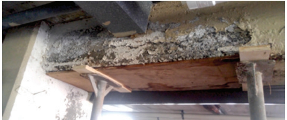
View of deteriorated concrete beam below a recreation deck.
