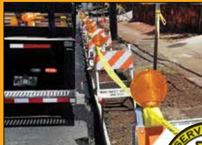
Temporary Traffic Control
