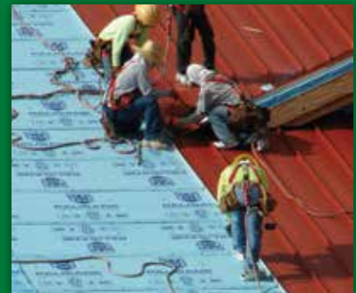
CUSTOM METAL ROOFING
