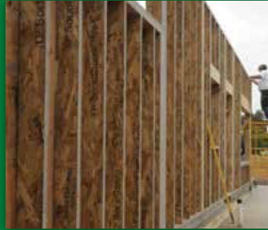
LSL WALL PANELS @ HOSPICE, KAMUELA
