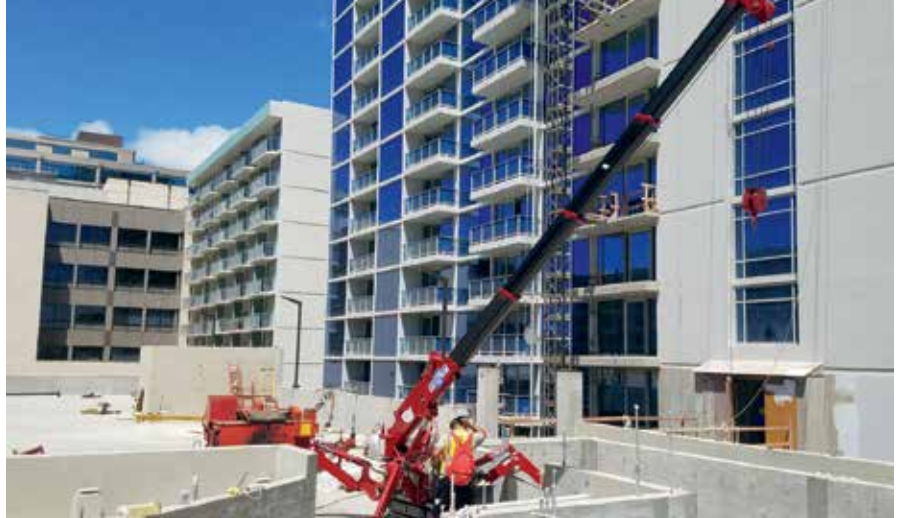
Hawaiian Dredging & Construction Co. Inc. used a new UNIC Spydercrane on the 100-foot parking deck to take delivery of materials over the side of the building from the ground.
