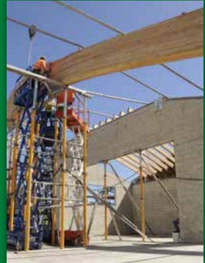
GLULAMS @ KEAUKAHA ELEMENTARY SCHOOL
