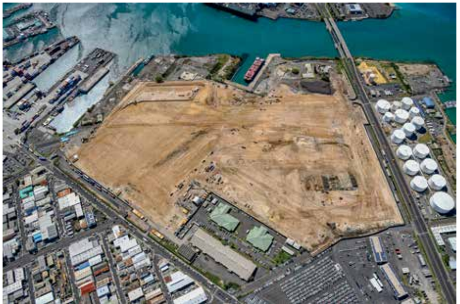
HDOT’s Kapalama Container Terminal Phase I, currently underway by Kiewit Infrastructure West PHOTO COURTESY HAWAII DEPARTMENT OF TRANSPORTATION
