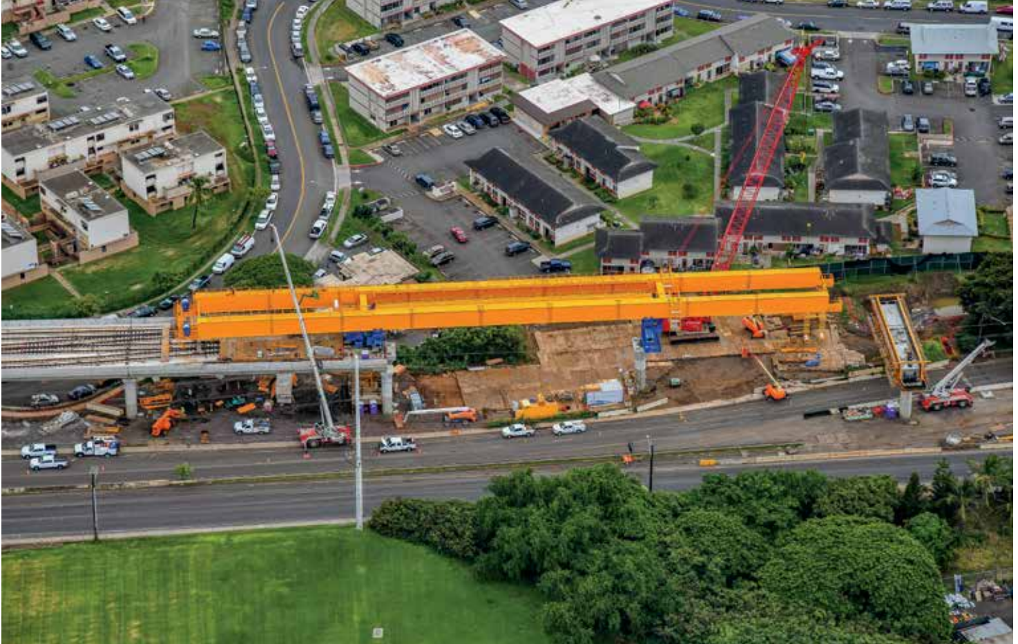
A gantry installs sections of HART's guideway between columns PHOTO COURTESY HART
