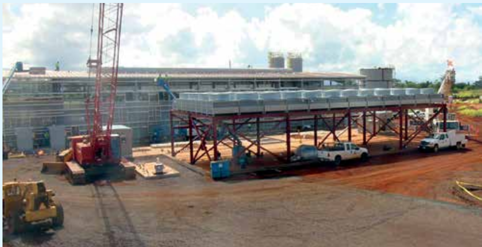
Hawaiian Electric delivers six 159-ton generators to the 50-megawatt power plant being constructed on eight acres of land on Schofield Barracks.
