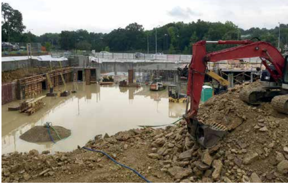
Flooded worksite after a storm
