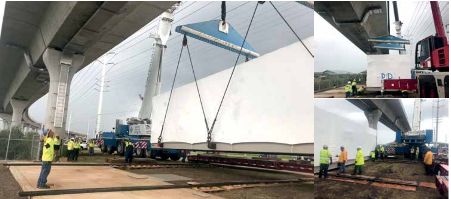
Hawaiian Crane recently designed and implemented a sliding system that helped them move a 120,000-pound HART Rail Control House 100 feet horizontally. PHOTO COURTESY HAWAIIAN CRANE & RIGGING
