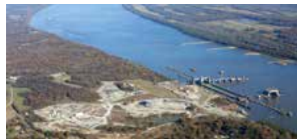
The Olmsted Locks and Dam
