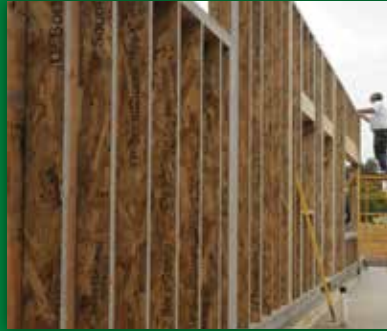
LSL WALL PANELS @ HOSPICE, KAMUELA
