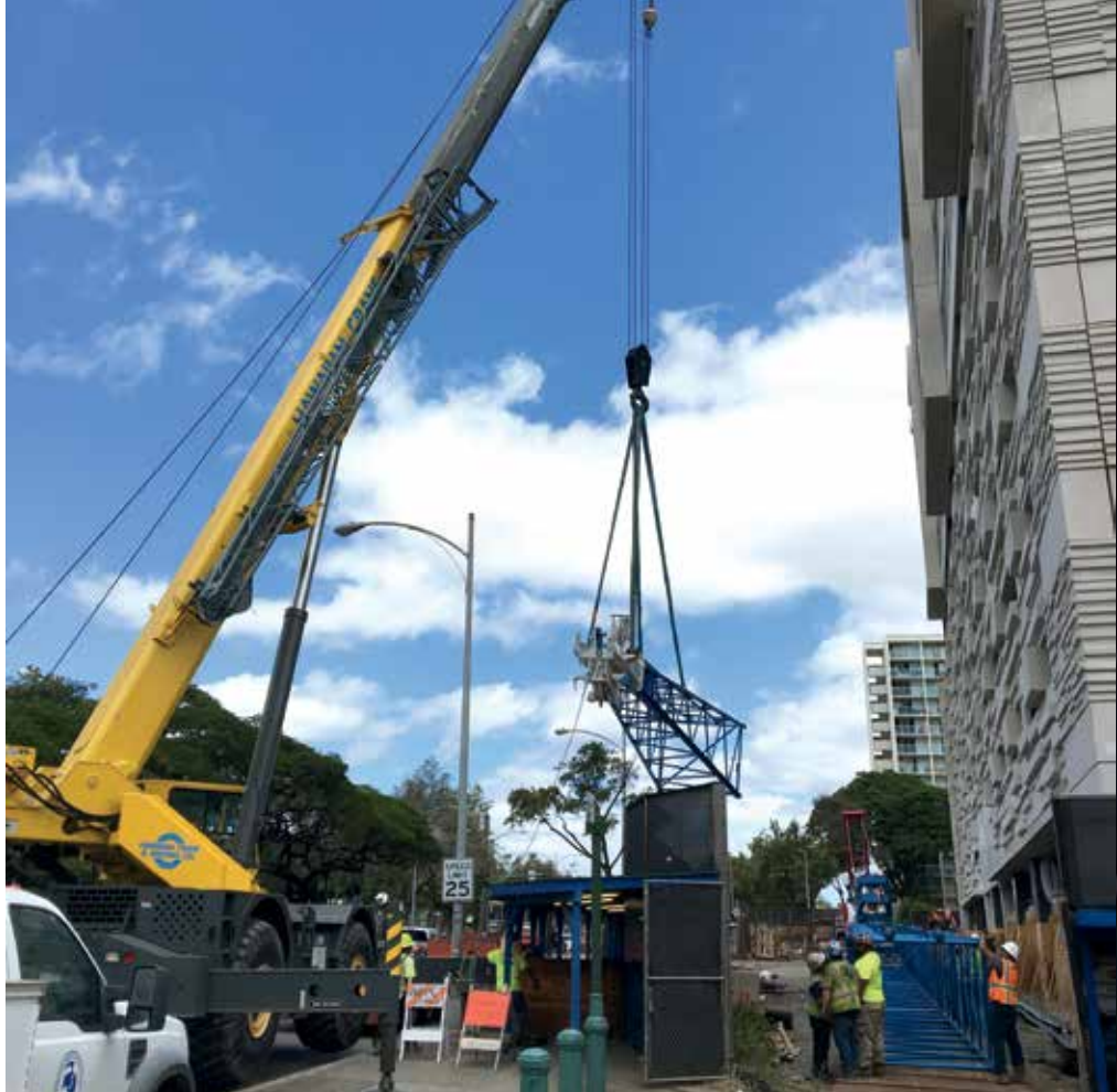
Crews from Hawaiian Crane & Rigging using their Grove RT875 crane to disassemble a Manitowoc 999 crane.
