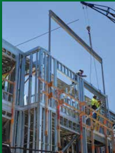
STEEL FRAMING @ KA MALANAI, KAILUA
