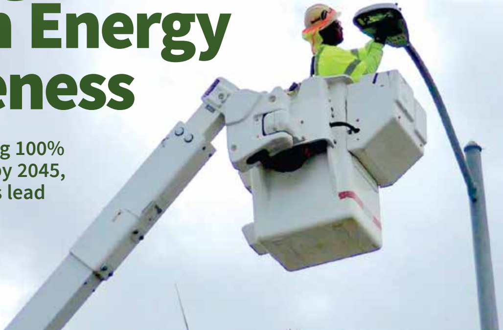
The City and County of Honolulu is installing LED light bulbs in street lights throughout the island. PHOTO COURTESY OF HAWAII ENERGY
