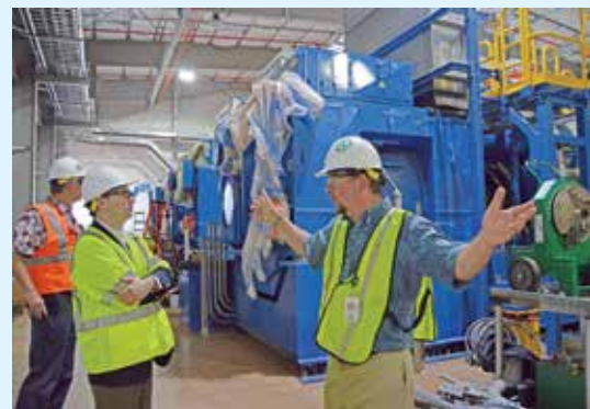
Acting Assistant Secretary of the Army for Installations, Energy and the Environment Jordan Gillis listens to Hawaiian Electric’s manager of generation project development Jack Shriver during a tour of the Schofield Barracks Generating Station.
