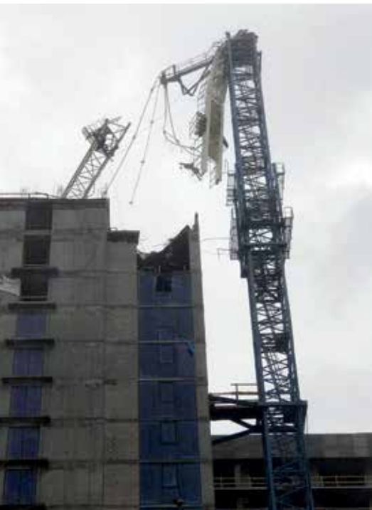
Crane collapse during a storm
