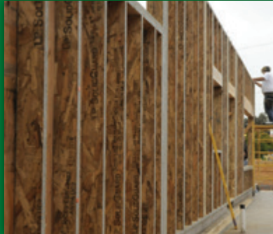
LSL WALL PANELS @ HOSPICE, KAMUELA
