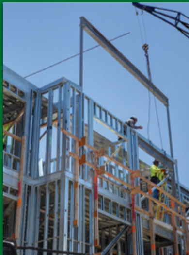
STEEL FRAMING @ KA MALANAI, KAILUA
