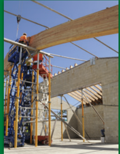
GLULAMS @ KEAUKAHA ELEMENTARY SCHOOL
