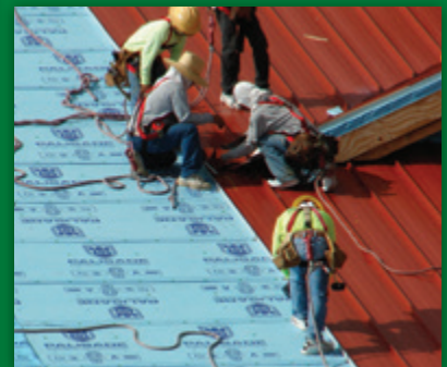
CUSTOM METAL ROOFING
