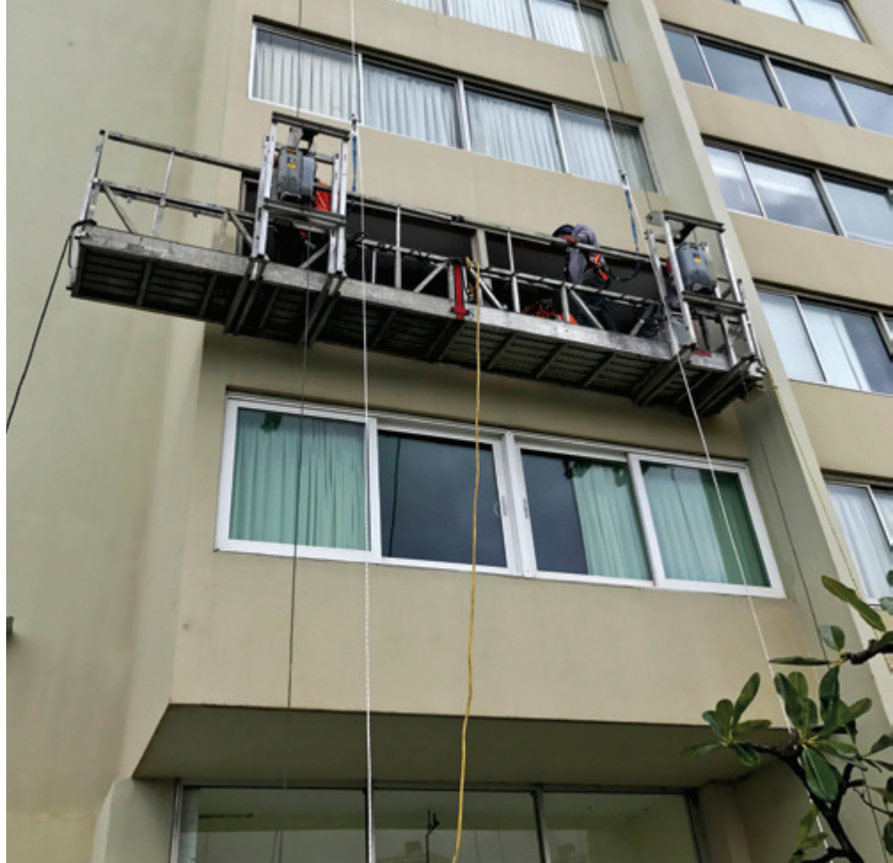
Coastal Windows installing high-rise windows
