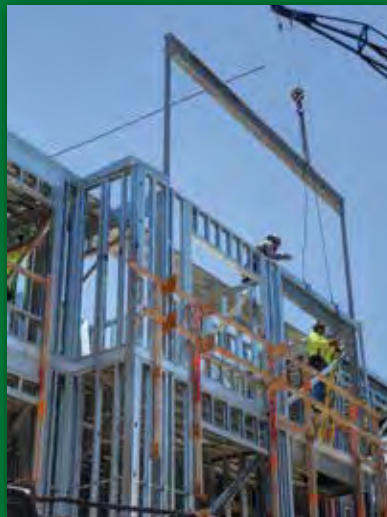
STEEL FRAMING @ KA MALANAI, KAILUA
