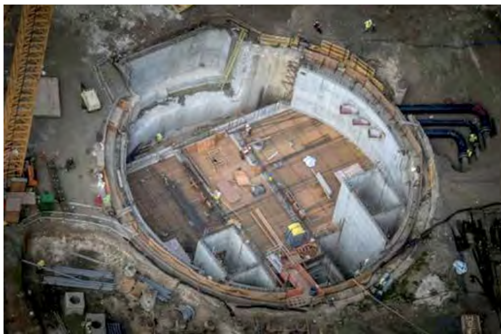
A view of Hensel Phelps’ 90-foot deep TIPS Pump Station, when it was approximately 60 percent complete. The completed Mini KIPS Pump Station protrudes from the TIPS Pump Station, which was shored during construction with ground-freezing technology.
