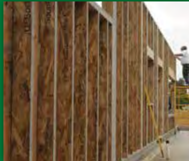
LSL WALL PANELS @ HOSPICE, KAMUELA
