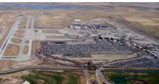
Site of the redevelopment of the Salt Lake City International Airport.
