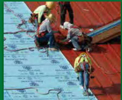
CUSTOM METAL ROOFING
