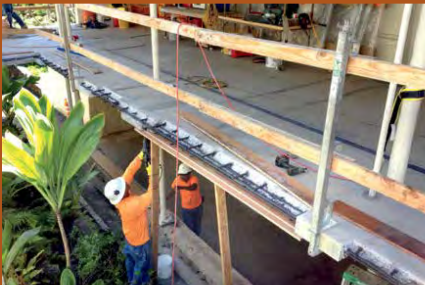
A recent deck repair by Structural Systems PHOTO COURTESY STRUCTURAL SYSTEMS INC.
