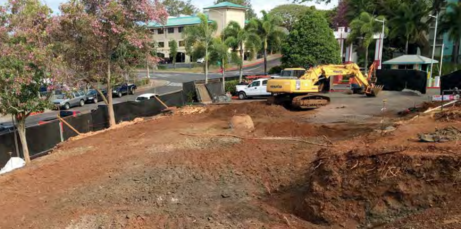
One of Unlimited Construction's ongoing projects is Moanalua Hillside Apartments. PHOTO COURTESY UNLIMITED CONSTRUCTION SERVICES INC.
