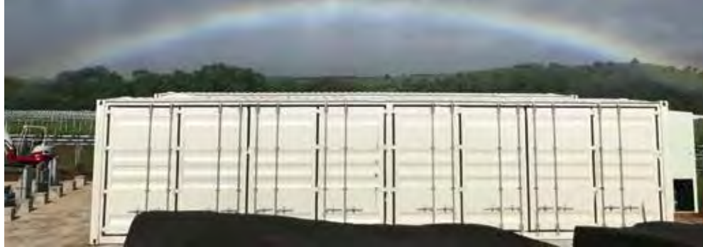
Energy storage container at the Lawai Solar and Energy Storage Project PHOTO COURTESY AES DISTRIBUTED ENERGY
