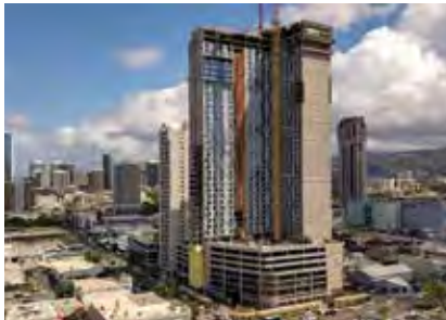
The final steel beam is lifted into place at HHC's Ke Kilohana tower. PHOTO COURTESY THE HOWARD HUGHES CORPORATION
