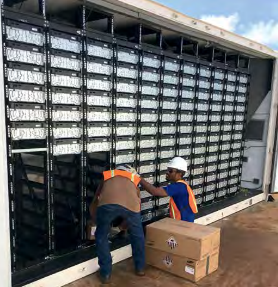
Ongoing construction at the Lawai Solar and Energy Storage Project PHOTO COURTESY AES DISTRIBUTED ENERGY
