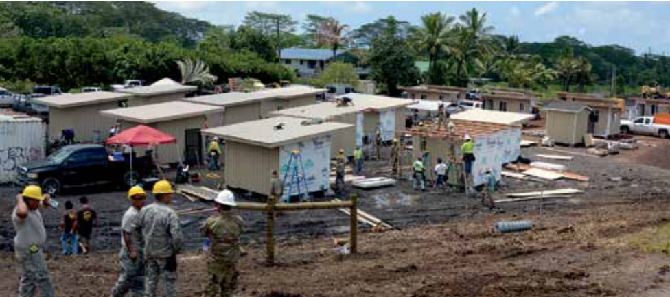
Soldiers from the 230th Vertical Engineer Company, Hawaii National Guard, construct 20 micro-shelters in Pahoia for residents displaced by the Kilauea eruptions.
