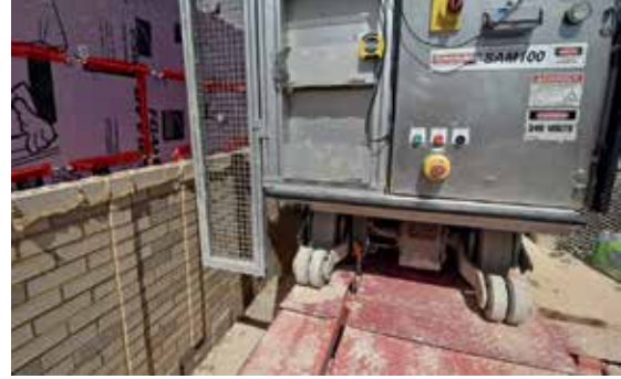
Construction Robotics' SAM100 lays bricks at the Jay and Susie Gogue Performing Arts Center at Auburn University in Alabama.
