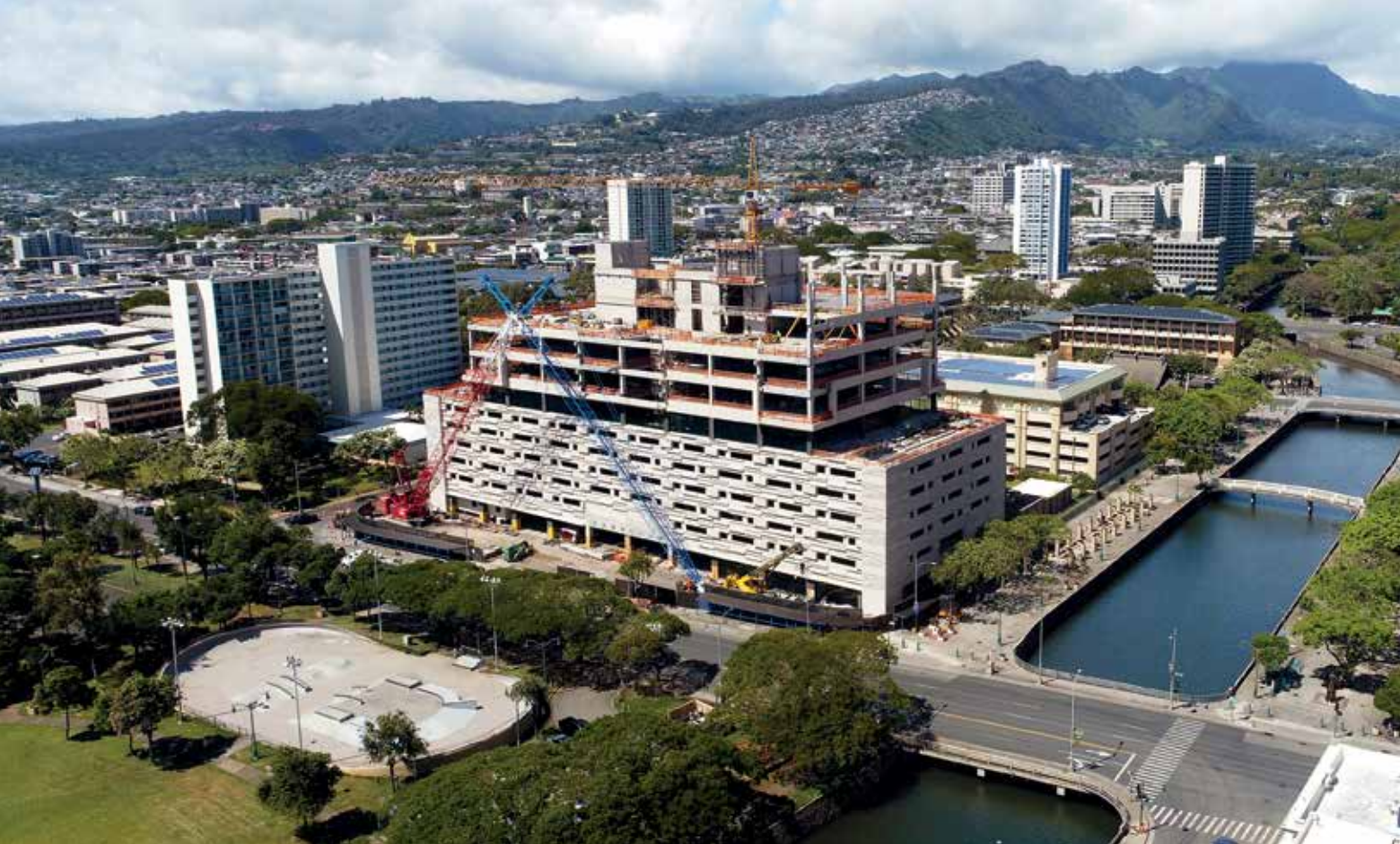
The American Savings Bank Tower is expected to wrap later this year. PHOTO COURTESY NORDIC PCL CONSTRUCTION INC.
