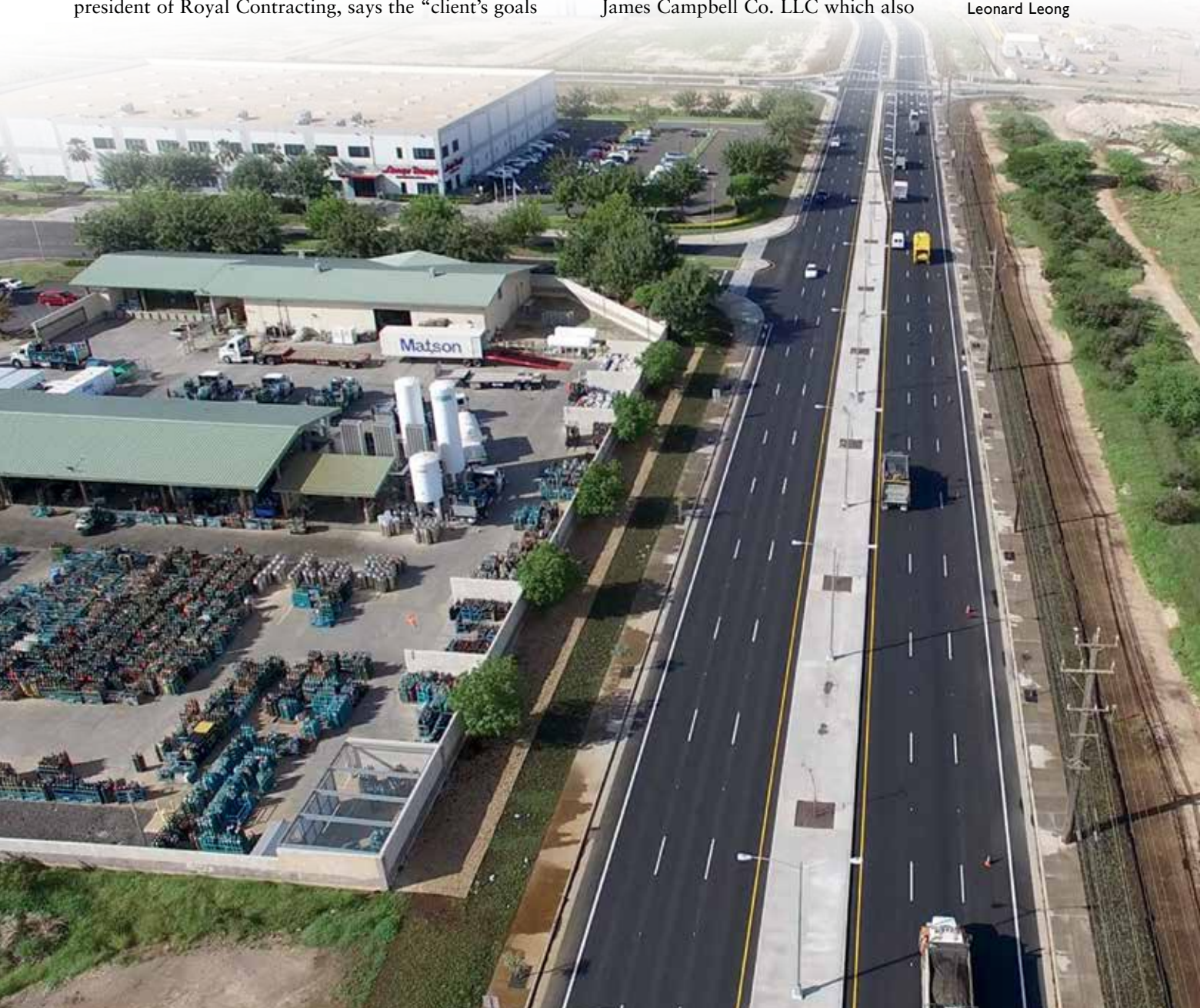
Royal Contracting's work on Kalaeloa Boulevard included widening the road from four lanes to six lanes.
