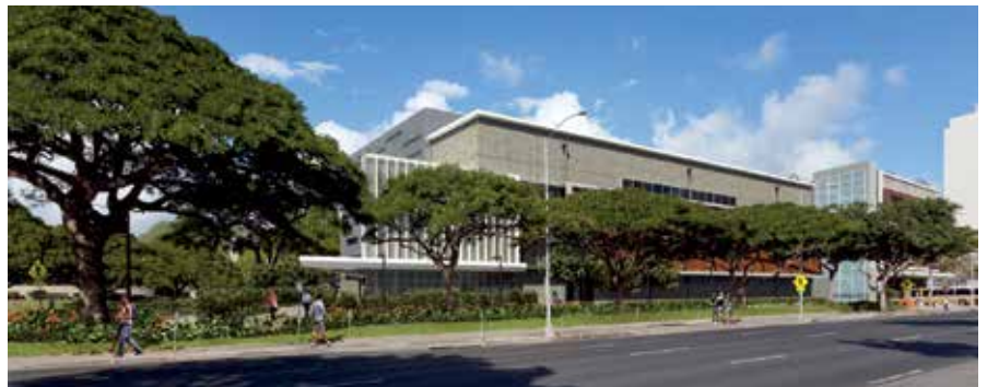
The Joint Traffic Management Center broke ground in April 2015.
