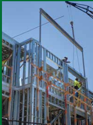
STEEL FRAMING @ KA MALANAI, KAILUA
