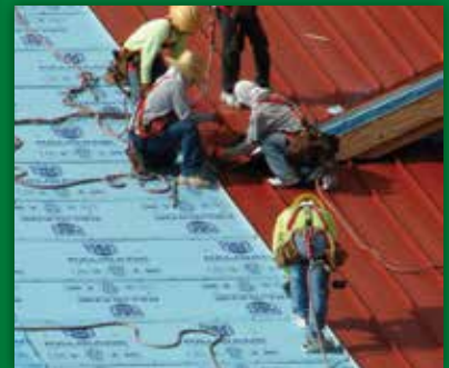
CUSTOM METAL ROOFING
