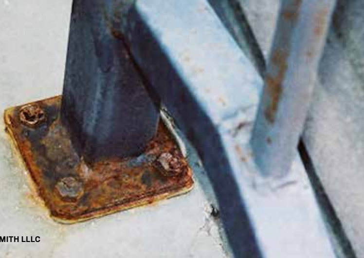
Corrosion of a railing stanchion
