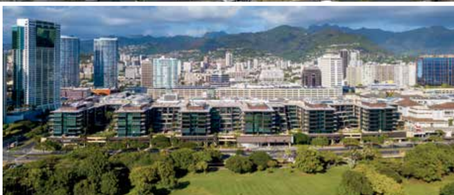
Park Lane after project completion
