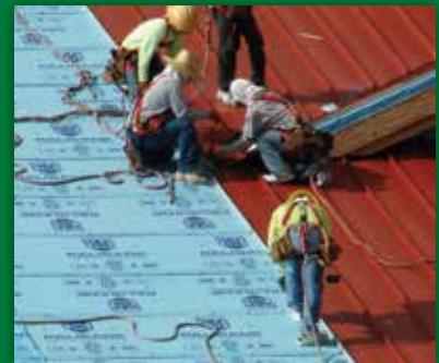
CUSTOM METAL ROOFING
