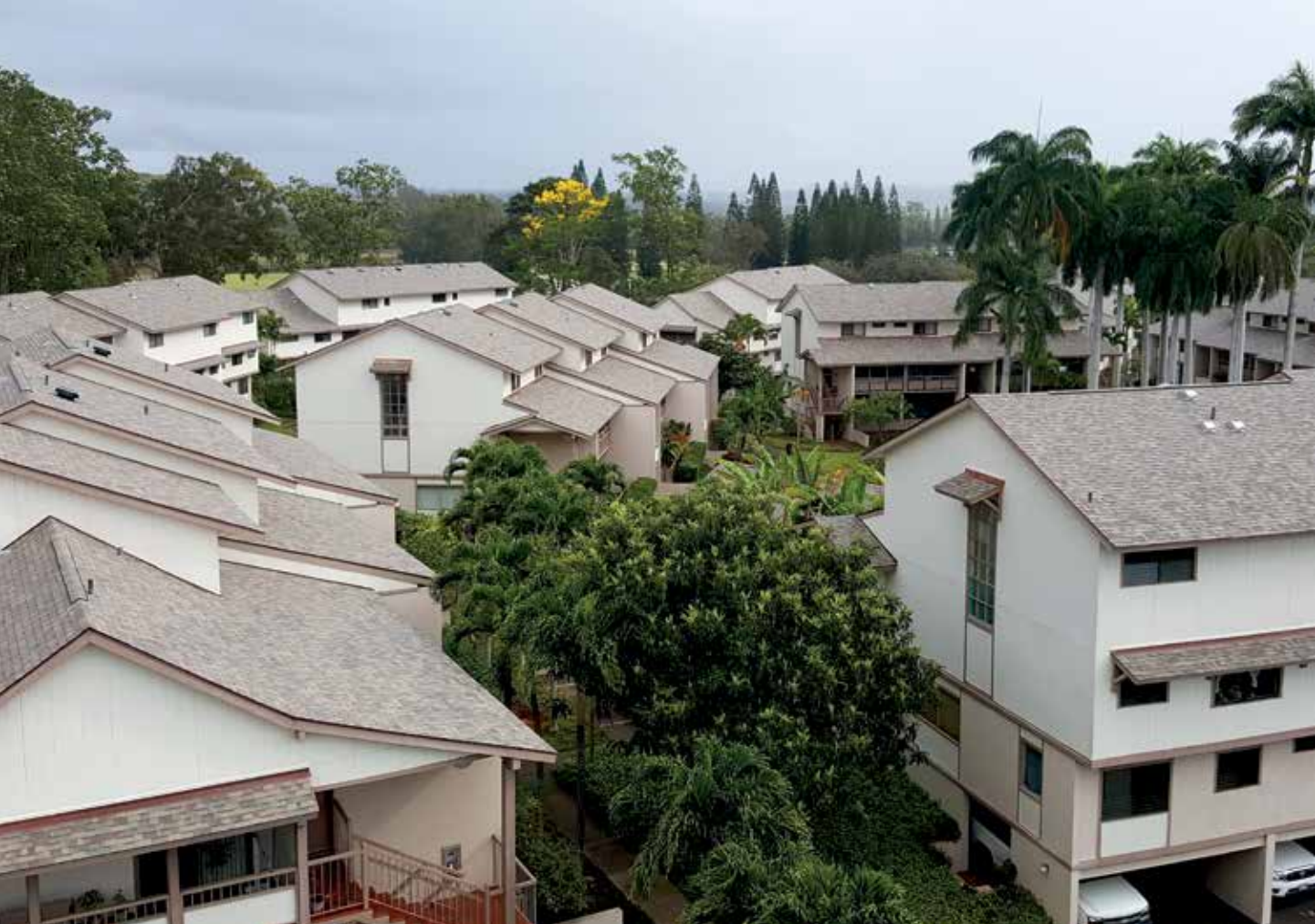
For AOA Kuahelani, CRV met and exceeded new energy code requirements with EnergyStar-compliant roofing, radiant barrier, ridge vents and solar fans. PHOTO COURTESY COMMERCIAL ROOFING & WATERPROOFING HAWAII INC.
