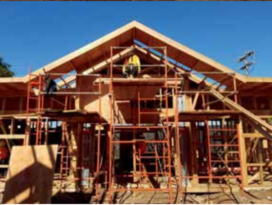
*Photo courtesy of Ku'uilei Ka'anoi, Allied Builders Systems
