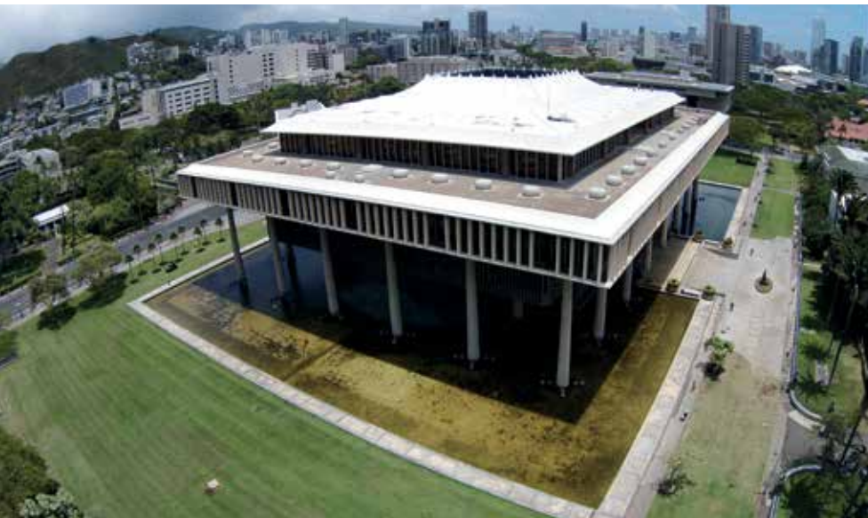
Tory's Roofing & Waterproofing reroofed the state Capitol Building in Downtown Honolulu last year.
