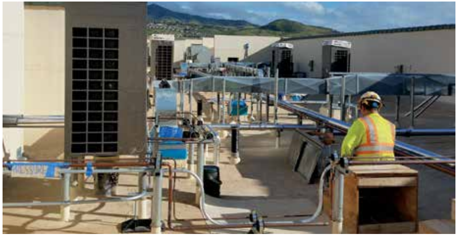
CRW worked with 850 pipe penetrations on the rooftop of the Embassy Suites in Kapolei.
