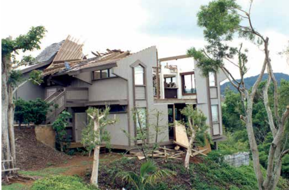
Hurricane Iniki resulted in more than $3 billion of damage.
