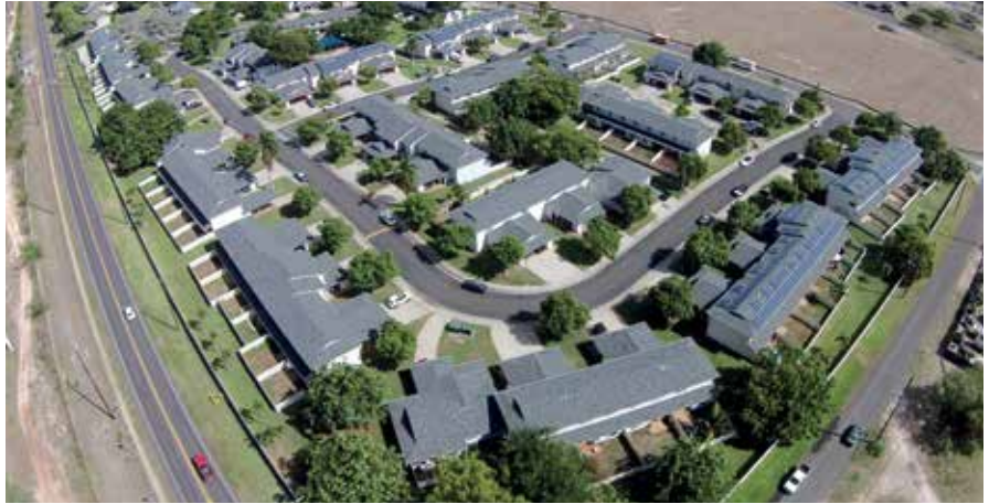
Tory's Roofing & Waterproofing began work on the Kalaeloa Kaimana project in 2017.
