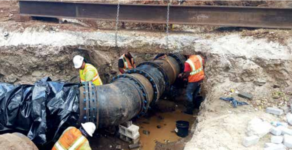
Nan Inc. recently completed work on the Airport Section utilities relocation. PHOTO COURTESY HART
