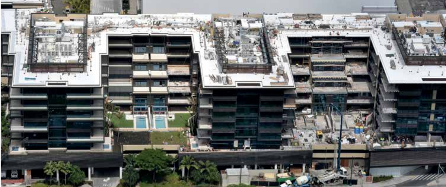
The Park Lane project involved the construction of eight buildings and two floors of parking.
