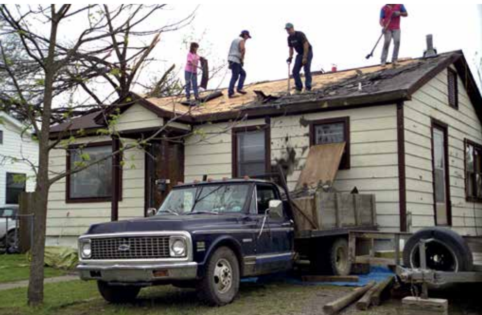
Floridians work on a roof damaged by Hurricane Andrew. PHOTO COURTESY FEDERAL EMERGENCY MANAGEMENT AGENCY
