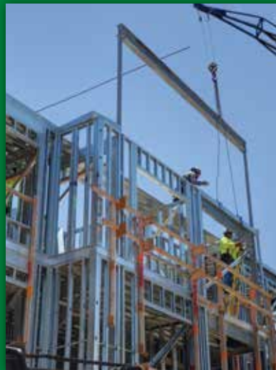
STEEL FRAMING @ KA MALANAI, KAILUA
