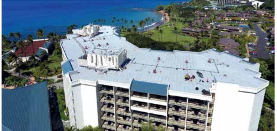
One of Cool Roof's projects last year was the Marriott Wailea's Haleakala Tower.
