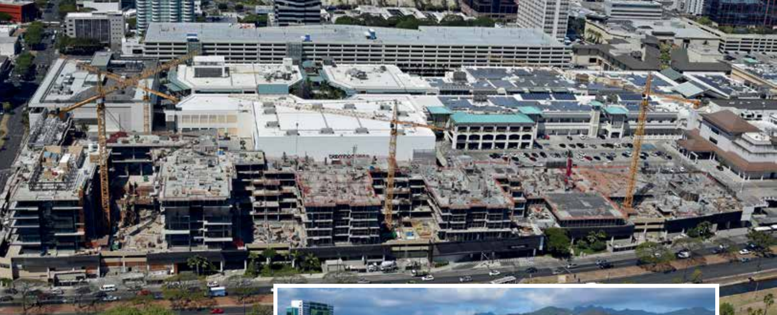
Four cranes in operation at the Park Lane construction site
