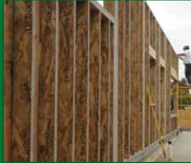
LSL WALL PANELS @ HOSPICE, KAMUELA
