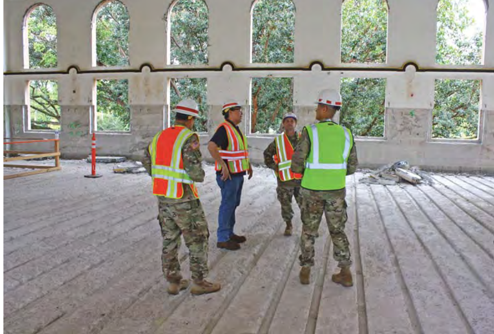
A USACE area engineer reports on renovations to Schofield Barracks' historic Quad D, Building 449, featured in the 1953 film, "From Here to Eternity." PHOTO COURTESY DINO W. BUCHANAN, USCAE-HONOLULU DISTRICT
