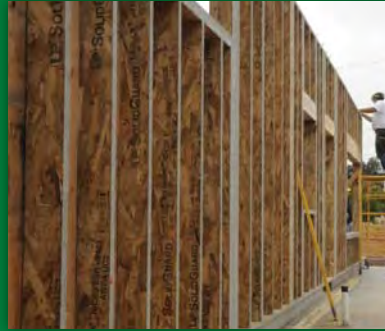
LSL WALL PANELS @ HOSPICE, KAMUELA
