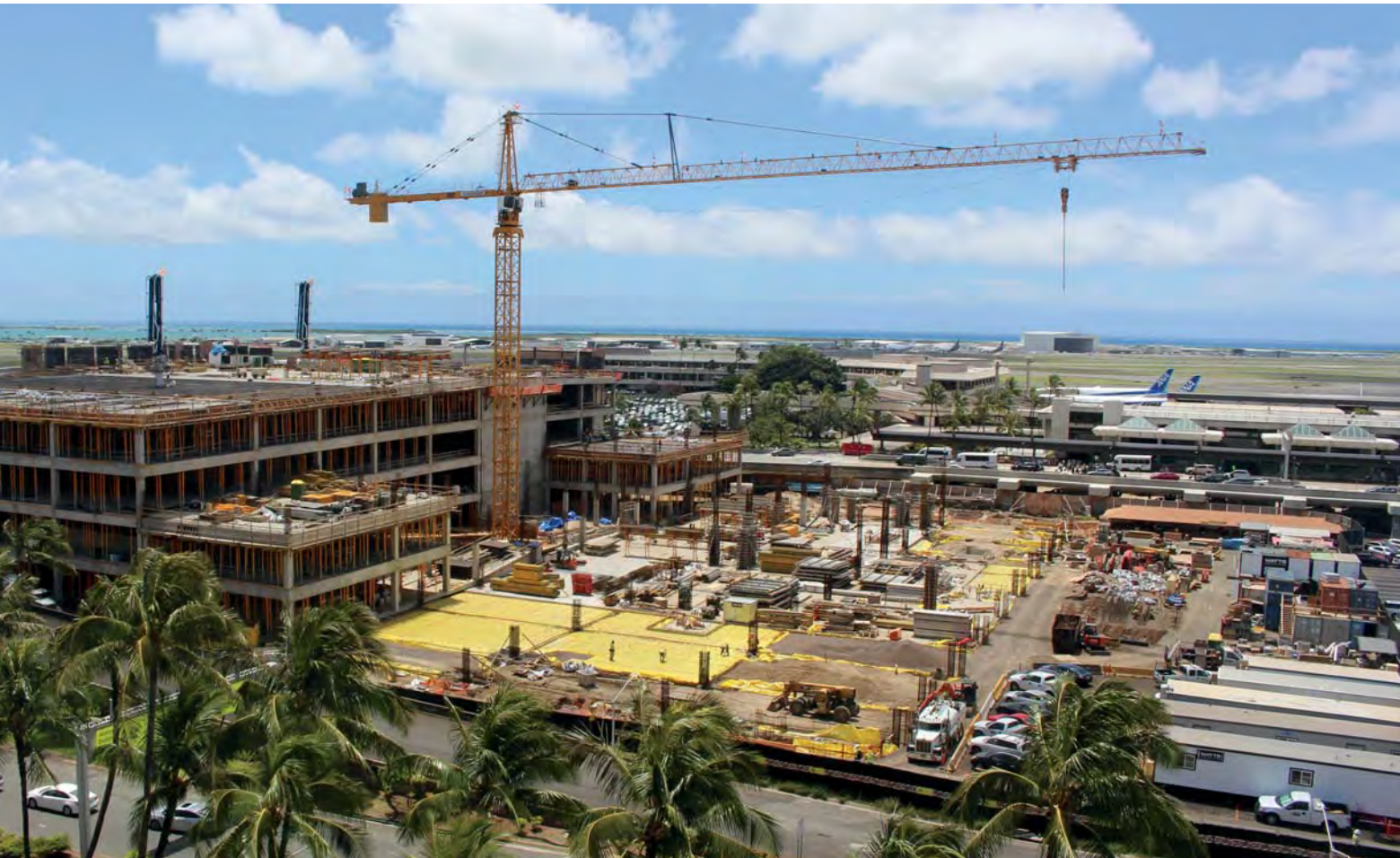
Honolulu’s new Daniel K. Inouye International Airport CONRAC is nearly 2 million square feet—most of it concrete. PHOTO COURTESY WATTS CONSTRUCTORS LLC
