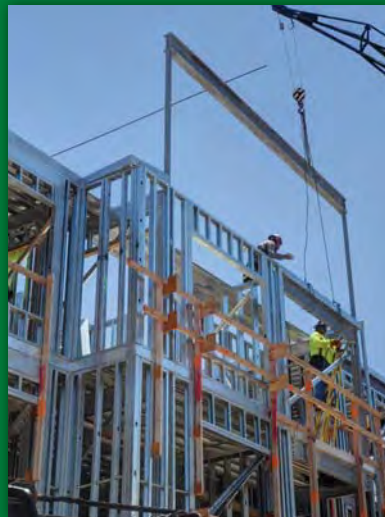
STEEL FRAMING @ KA MALANAI, KAILUA
