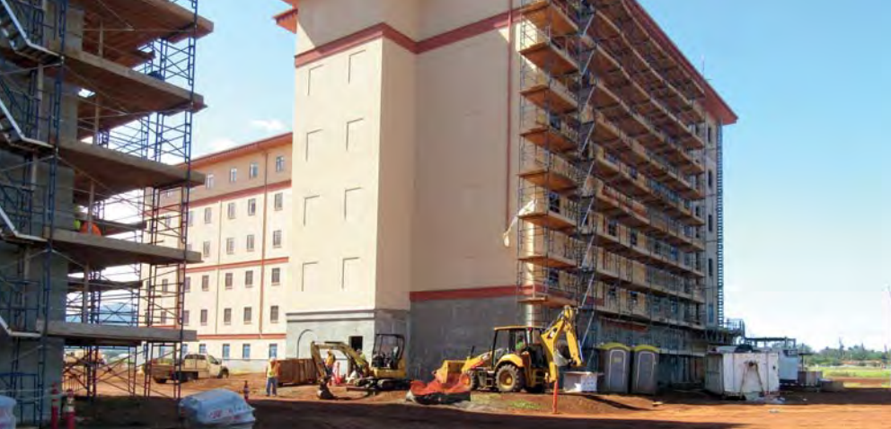
Wheeler Army Airfield's $69.7 million Combat Aviation Brigade Phase 2 project, completed by Nan Inc. PHOTO COURTESY DINO W. BUCHANAN, USCAE-HONOLULU DISTRICT
