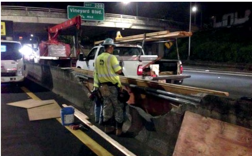
Hawaii Department of Transportation crews repair a barrier on H-1. PHOTO COURTESY HAWAII DEPARTMENT OF TRANSPORTATION
