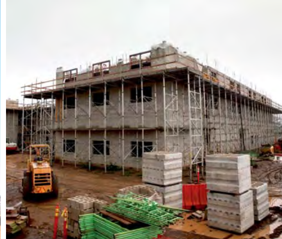
New MCBH MV-22 barracks under construction PHOTO COURTESY MARINES OFFICIAL WEBSITE
