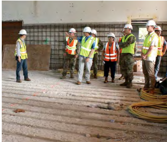
USACE Pacific Ocean Division Commander Col. Thomas J. Tickner (fourth from right, green vest) reviews renovations at Schofield Barracks' historic Bldg. 449, Quad D, in October 2017. PHOTO COURTESY DINO W. BUCHANAN, USCAE-HONOLULU DISTRICT
