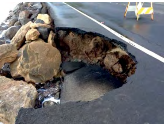
Damaged shoulder area in Kaaawa PHOTO COURTESY HAWAII DEPARTMENT OF TRANSPORTATION
