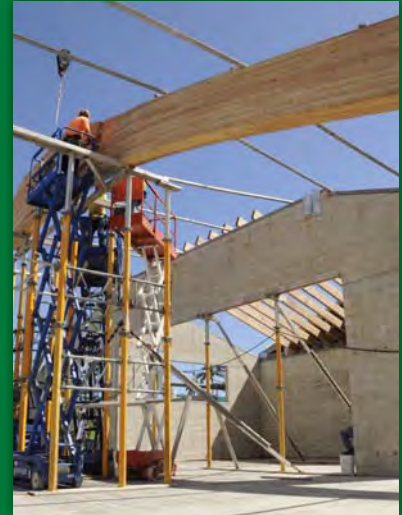
GLULAMS @ KEAUKAHA ELEMENTARY SCHOOL
