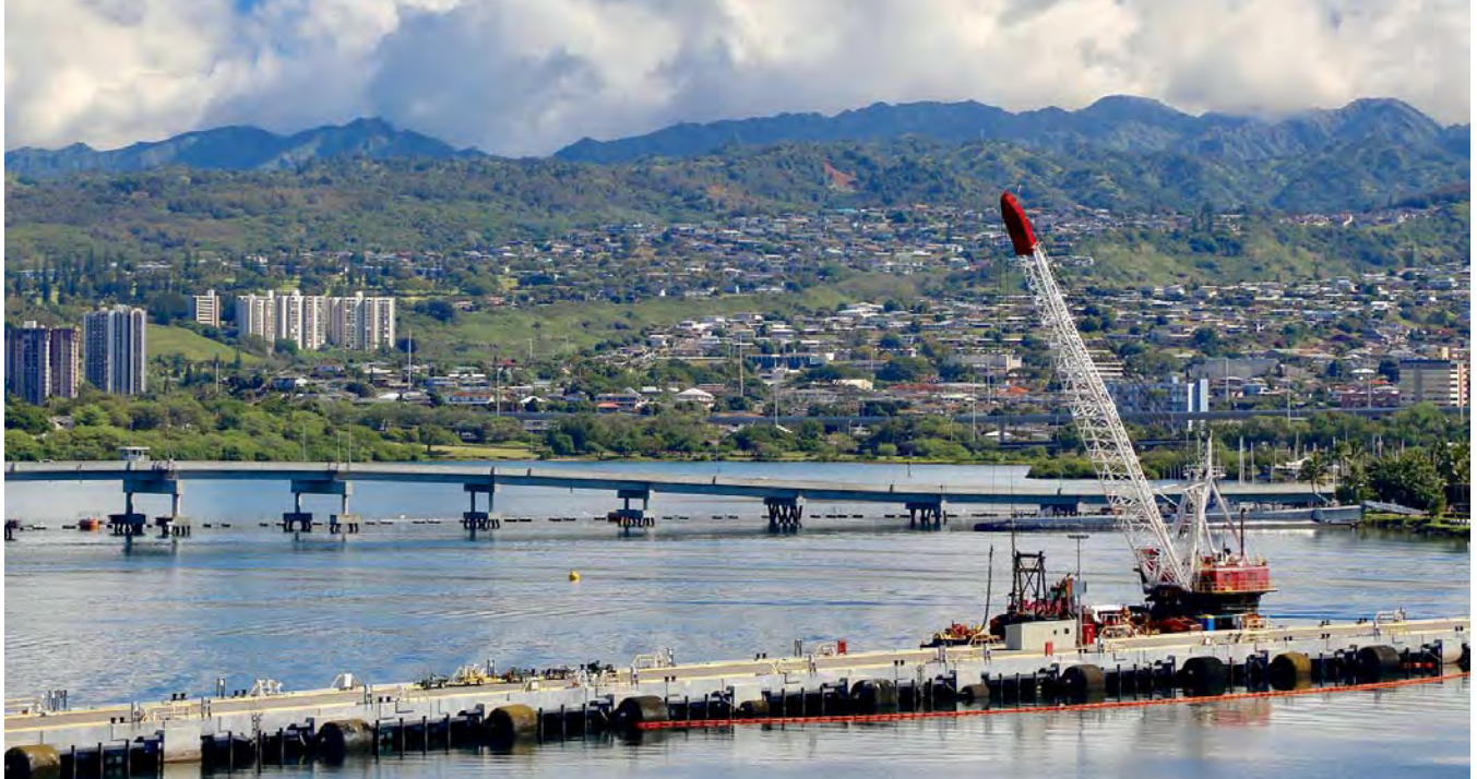
Hotel Pier at JBPHH is the first of several piers that will be dredged to its original design depth. PHOTO COURTESY SHANNON HANEY/NAVFAC HAWAII PUBLIC AFFAIRS
