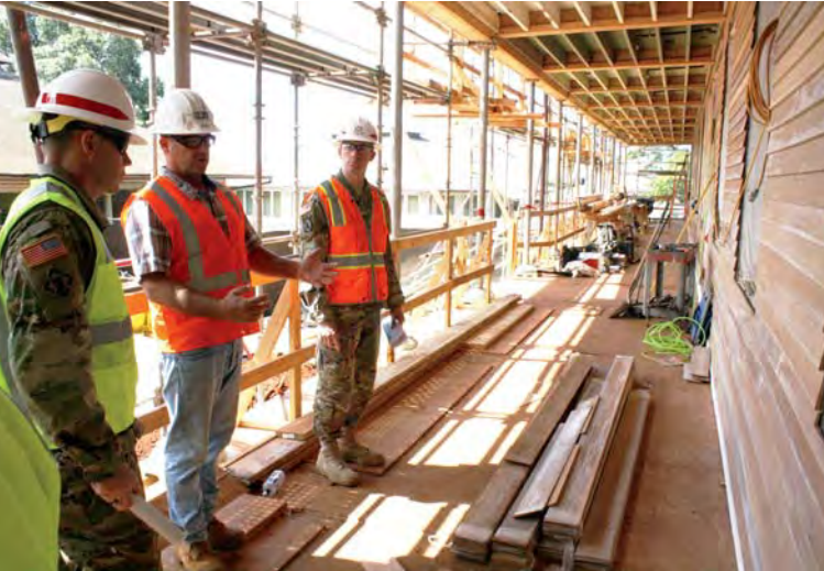
The USACE recently completed renovations to Palm Circle’s historic Bldg. 112 at Fort Shafter.
