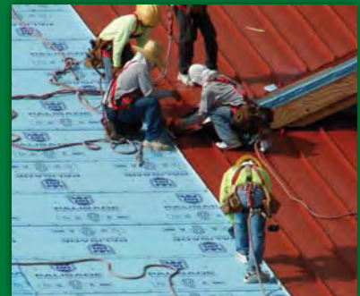
CUSTOM METAL ROOFING
