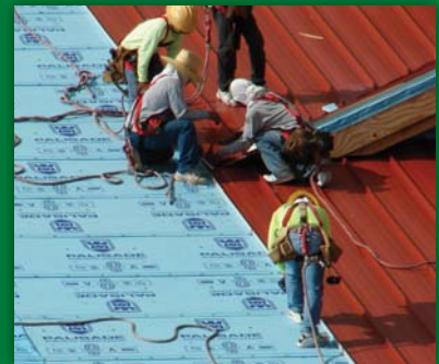
CUSTOM METAL ROOFING
