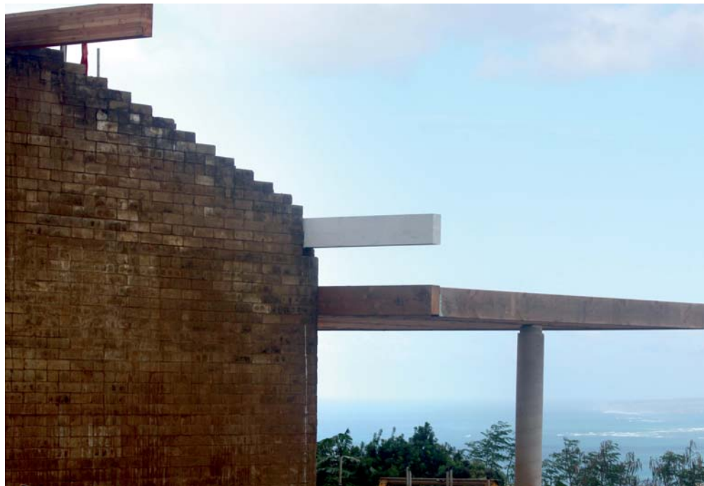
The builders needed to make 40,000 bricks out of the Maui mud for the walls of the house.
