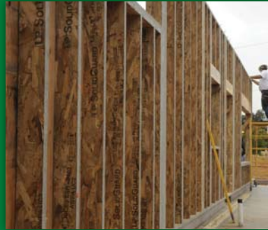
LSL WALL PANELS @ HOSPICE, KAMUELA
