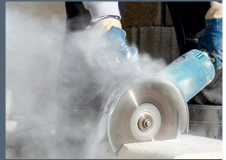
Construction companies are required to protect employees from exposure to the dangers of silica dust.
