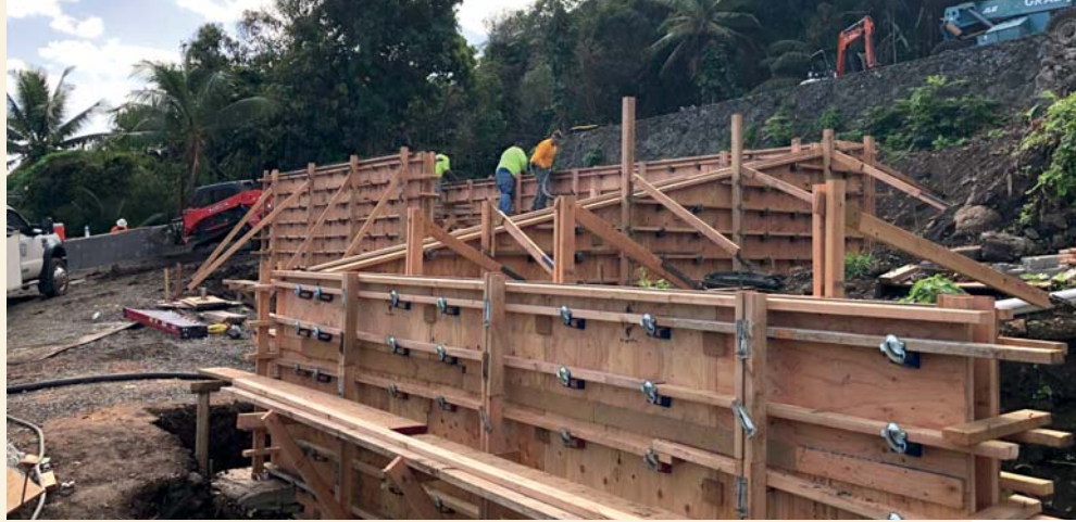
Complete Construction Services’ jobs include a remodel project in Nuuuanu.
