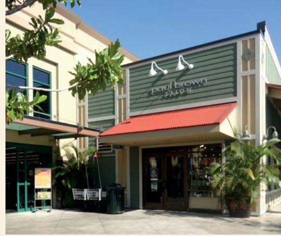
Complete Construction Services handled a commercial tenant improvement project in Kailua.
