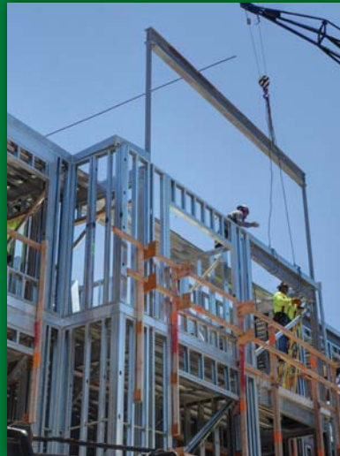
STEEL FRAMING @ KA MALANAI, KAILUA
