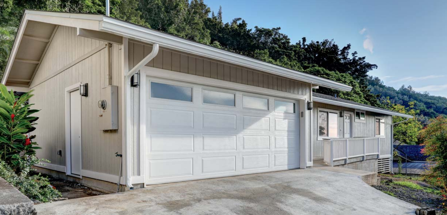
A Pauoa home rebuilt by Graham Builders
