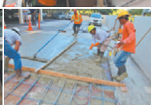
PARKING DECK & PT CABLE REPAIRS
