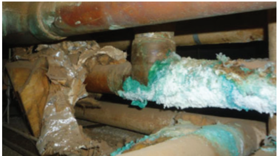
Domestic Water Supply Corrosion Conditions
