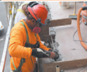
HIGH-RISE SPALL REPAIR
