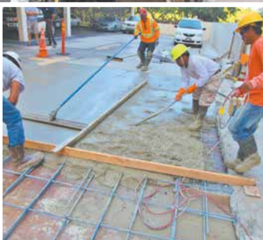
PARKING DECK & PT CABLE REPAIRS
