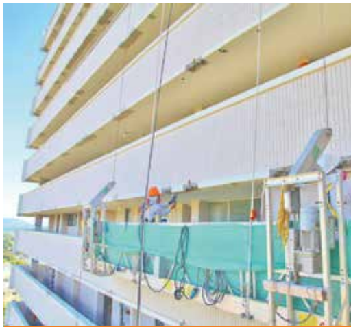
HIGH-RISE SPALL REPAIR
