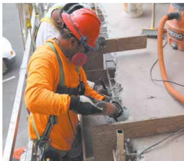
HIGH-RISE SPALL REPAIR
