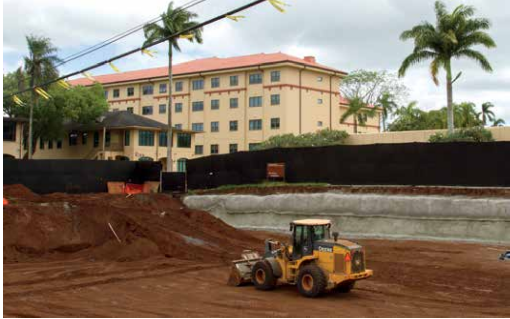
Swinerton Builders is working with the U.S. Army on a new parking structure at Schofield Barracks. PHOTO COURTESY U.S. ARMY
