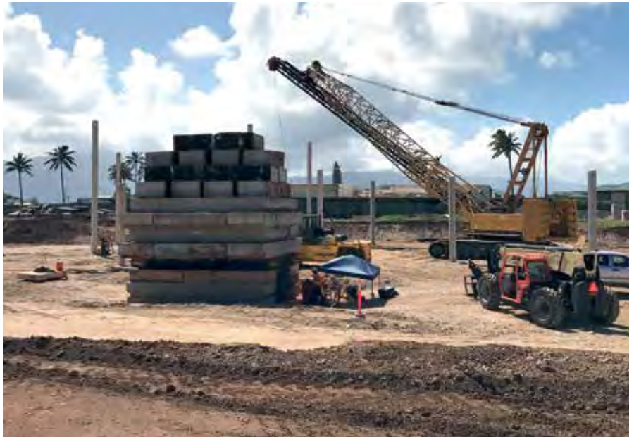
Caddell-Nan Joint Venture load-tests the concrete pile foundation for the new Marine Corps Base Hawaii Medical/Dental Clinic.
