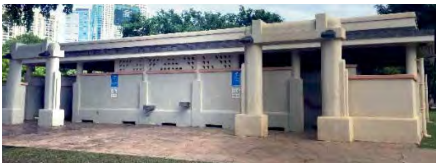
The Diamond Head bathhouse is being renovated by Amethyst Builders Inc.
