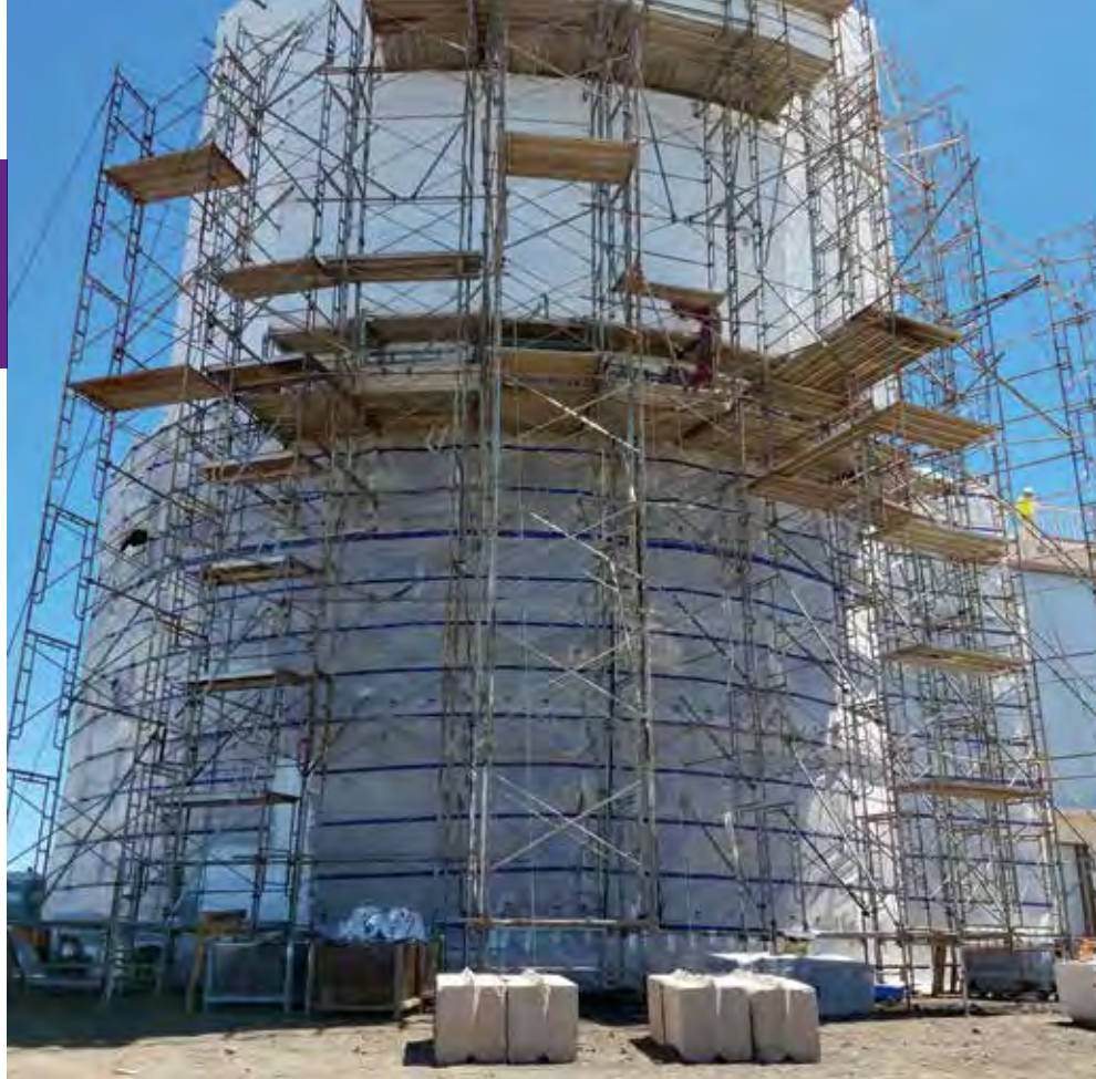
Lead paint mitigation on a Mauna Kea telescope requires specialized equipment and allowances for the high altitude.
