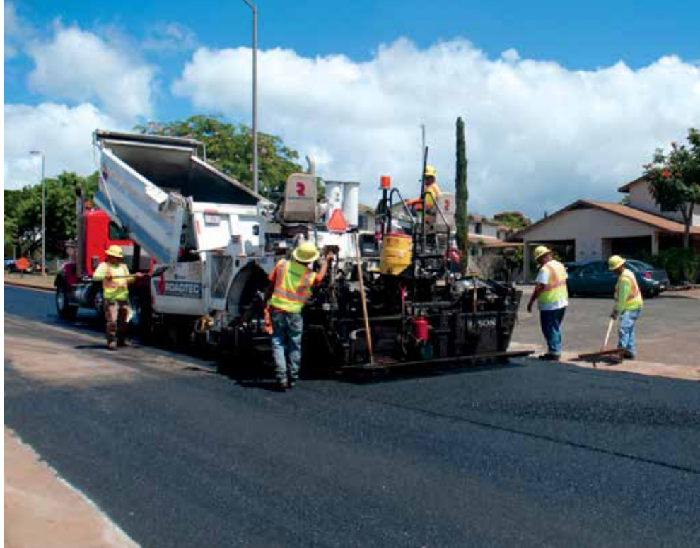
Crews from Grace Pacific LLC repaving Lauhala Road near the Wili Wili neighborhood at Wheeler Army Airfield.
