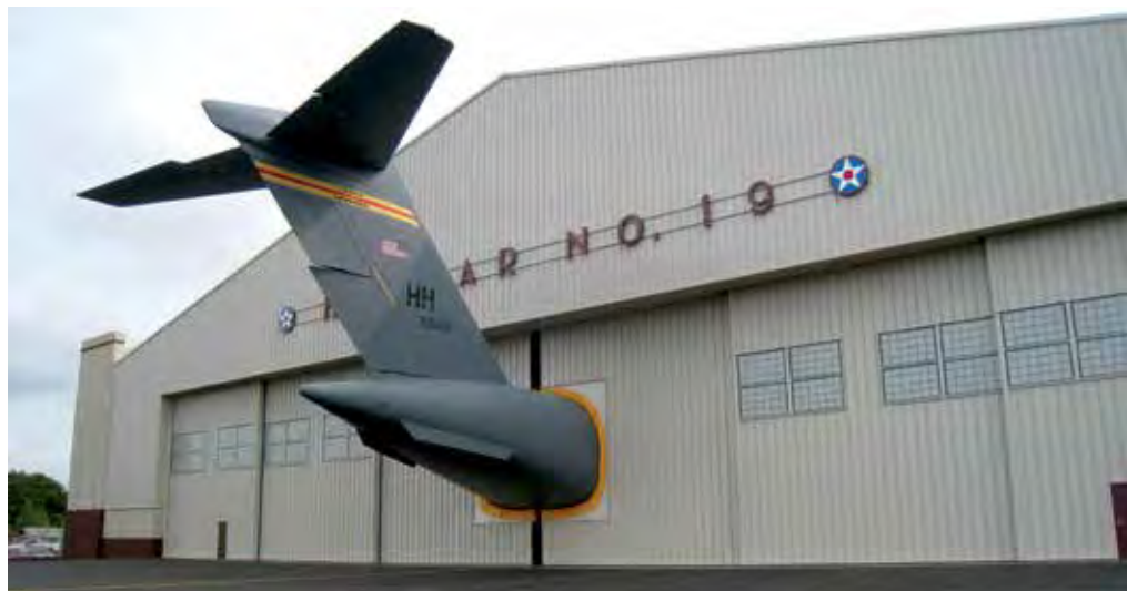
The tail section of a C-17 sticks out of Hangar 19 at Hickam while its nose fuel cell receives maintenance.
