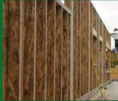
LSL WALL PANELS @ HOSPICE, KAMUELA
