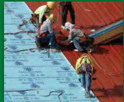
CUSTOM METAL ROOFING
