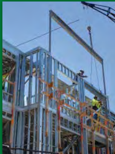
STEEL FRAMING @ KA MALANAI, KAILUA
