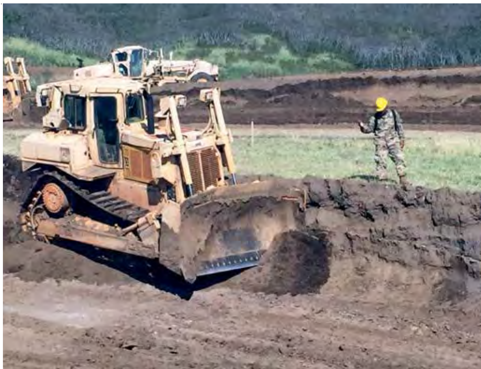
Soldiers from the U.S. Army Corps of Engineers work on the Range 5 Trench Construction Project on Marine Corps Base Hawaii. The recently completed live-fire trench warfare system facility will provide increased readiness for land forces across Hawaii.
