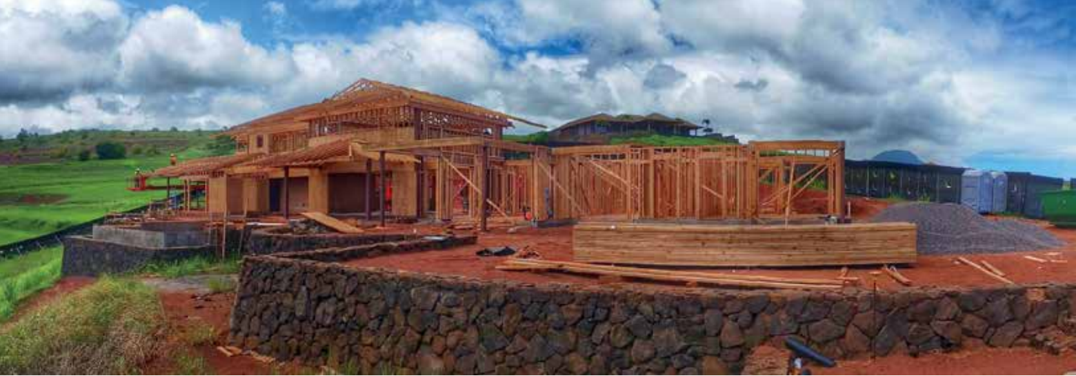
Lava rock walls surrounding monolithic slab and frame
