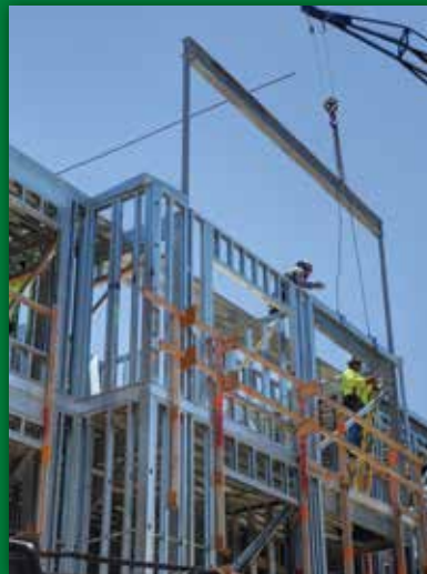
STEEL FRAMING @ KA MALANAI, KAILUA
