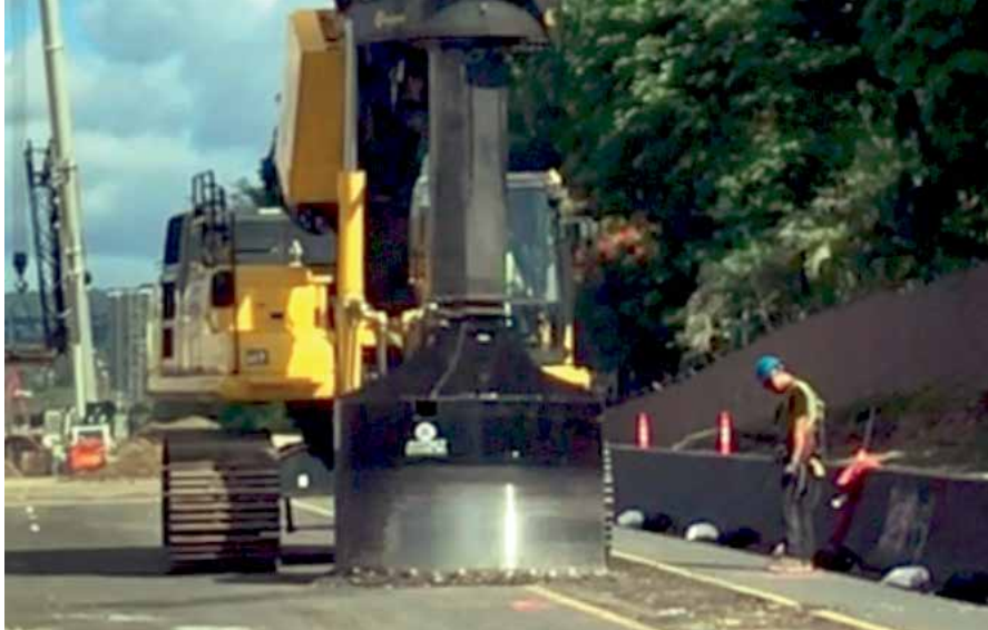
Crews from Shimmick/Traylor/Granite JV prepare Kamehameha Highway near Aloha Stadium for pouring the foundations for the rail guideway. PHOTO COURTESY HART
