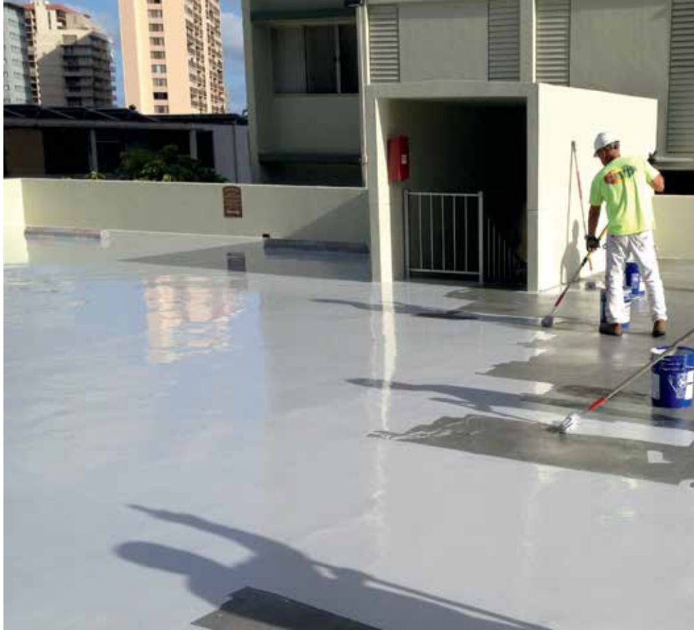
Crews from Ford Painting Professionals waterproofing at the Crown Thurston PHOTO COURTESY FORD PAINTING PROFESSIONALS
