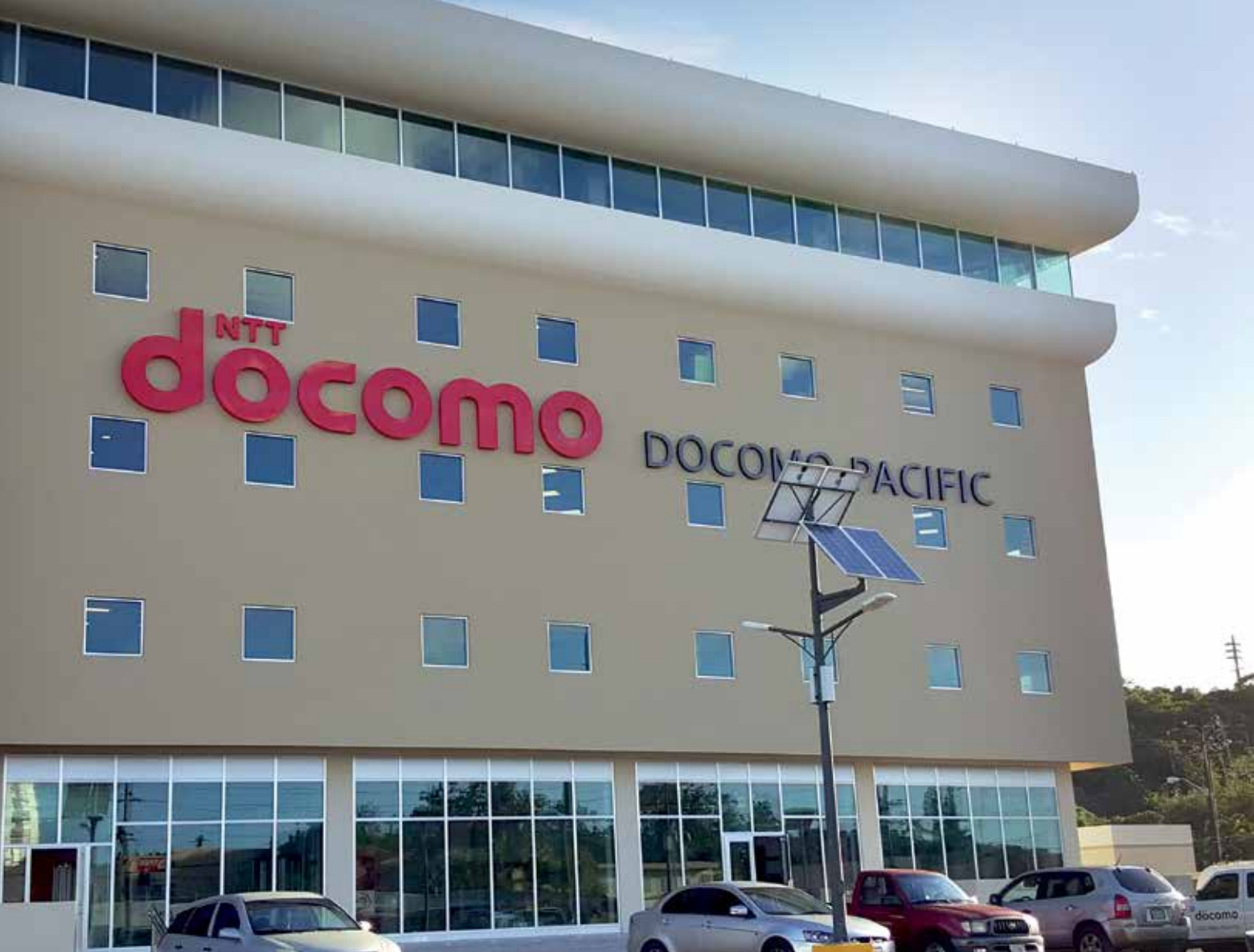
Docomo Pacific's new headquarters
