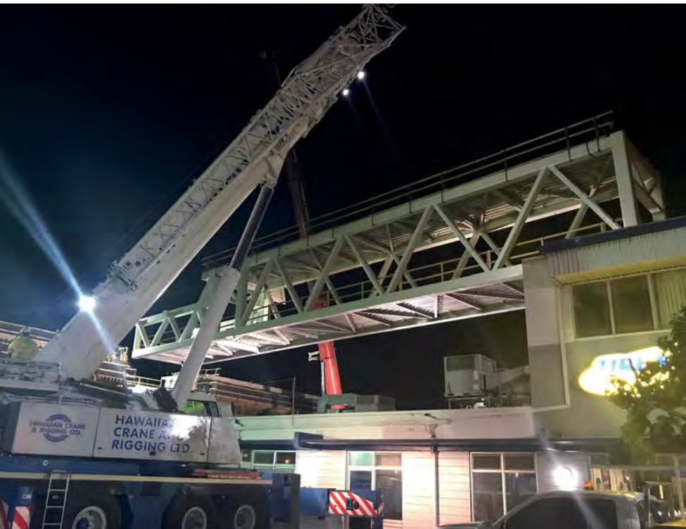
Hawaiian Crane & Rigging installing HART pedestrian bridge PHOTO COURTESY HAWAIIAN CRANE & RIGGING LTD.
