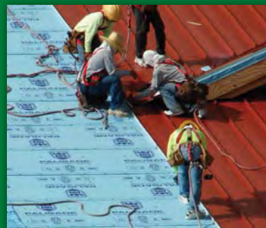
CUSTOM METAL ROOFING
