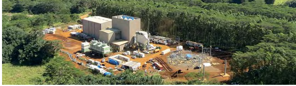
A biomass-to-energy facility on Kauai
