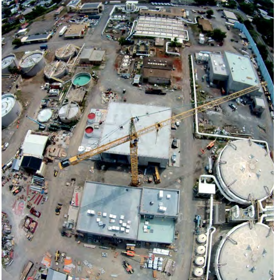
Hensel Phelps is using AR to manage the Kailua-Kaneohe Gravity Sewer Tunnel TIPS project. PHOTO COURTESY BOWERS + KUBOTA/TONY JONES
