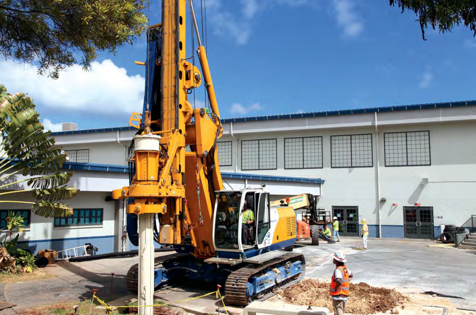
Kelikai Inc.'s BG15H drill rig installs 5-foot diameter caissons/drilled shafts at Ewa Makai Middle School.
