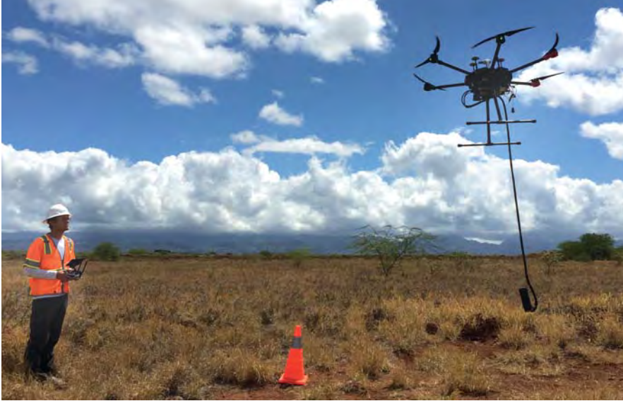
A HECO employee used a drone to survey the future site of a solar facility at Joint Base Pearl Harbor-Hickam West Loch Annex. PHOTO COURTESY HAWAII ELECTRIC
