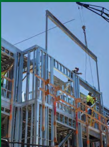
STEEL FRAMING @ KA MALANAI, KAILUA
