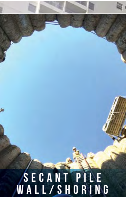
AUGERCAST PILES
