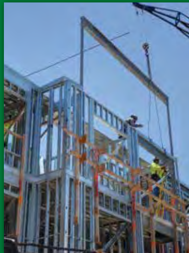
STEEL FRAMING @ KA MALANAI, KAILUA
