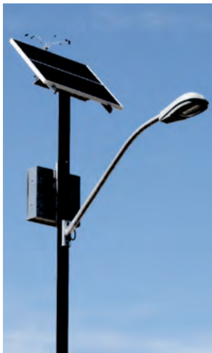
Newer distributed solar lighting fixture with high-performance LEDs for high lumen levels, but heavier loads and larger foundations.
