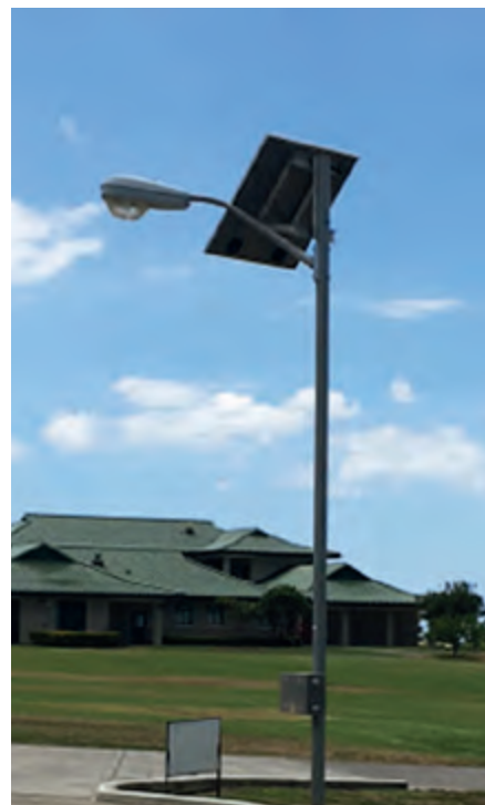
Older distributed solar lighting fixture with outdated cobra head, large solar panel and battery box at the base.
