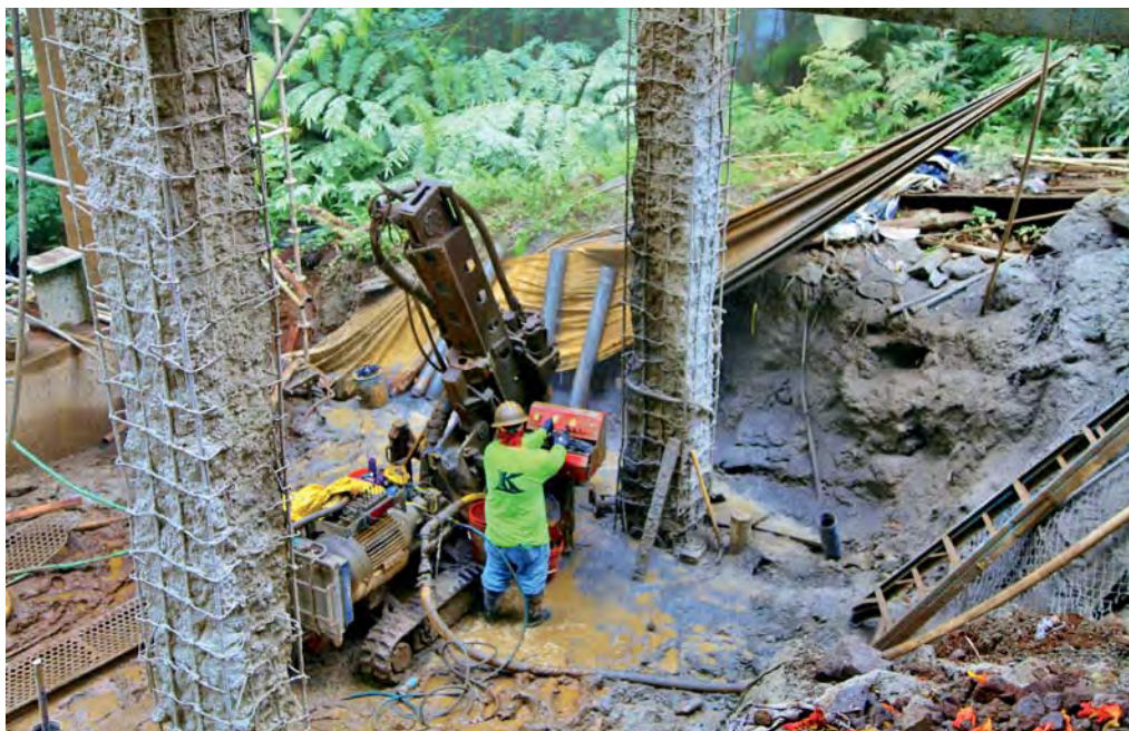
Kelikai Inc. workers add reinforcing bars to the pillars.
