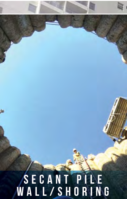
AUGERCAST PILES
