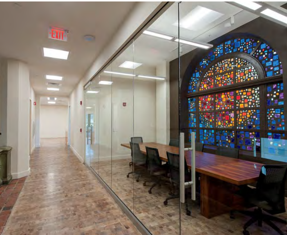
Second-floor conference room and Blox-On-End corridor flooring © 2017, DAVID FRANZEN
