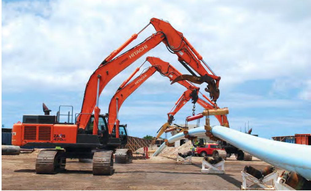
Healy Tibbitts installs fusible PVC pipe into new underwater steel casing. PHOTO COURTESY HEALY TIBBITTS BUILDERS INC.
