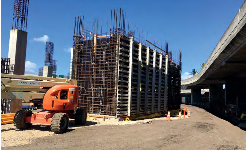
Watts Constructors is using auger cast piles at Honolulu’s new CONRAC. PHOTO COURTESY WATTS CONSTRUCTORS LLC
