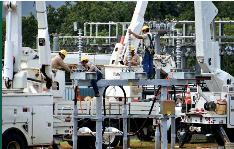
Worker from KIUC begin connecting the Kapaia Power Station to the Tesla solar farm, the first utility-scale dispatchable solar project in the world. PHOTO COURTESY KIUC
