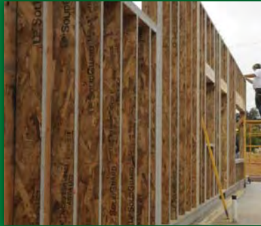
LSL WALL PANELS @ HOSPICE, KAMUELA
