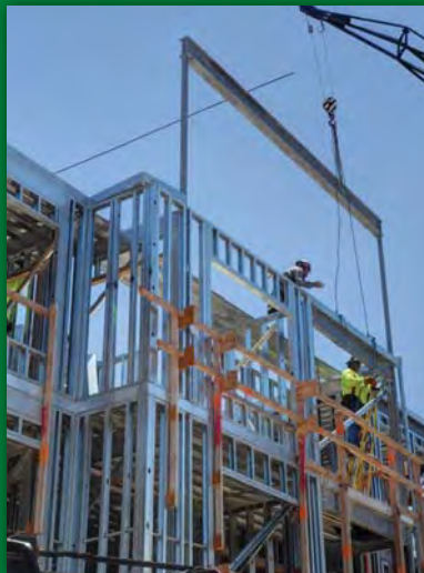
STEEL FRAMING @ KA MALANAI, KAILUA
