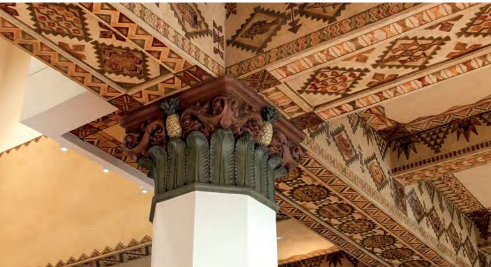
Restored column capital and faux painted beams
