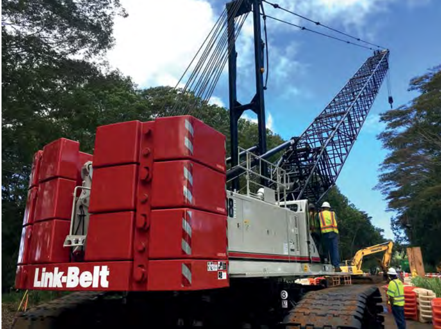
W.W. Clyde & Company puts Doc Bailey's 238 HSL 150-ton lattice tele crawler crane to work on the Bridge 7E replacement project on Kauai.
