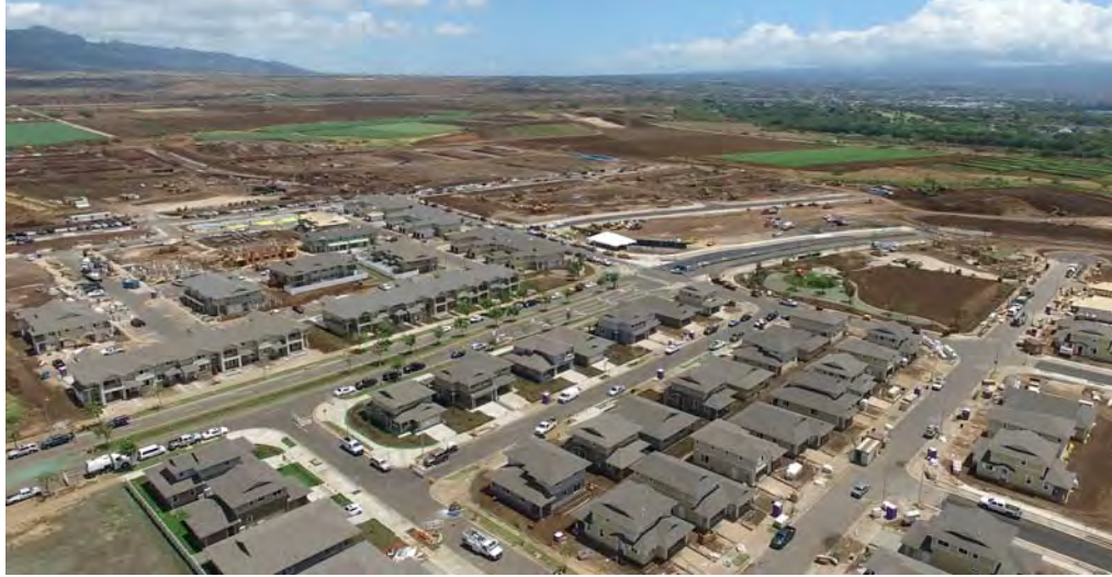
Royal Contracting is prepping 100 acres for Hoopili Phases 1 and 3. PHOTO COURTESY ROYAL CONTRACTING CO. LTD.
