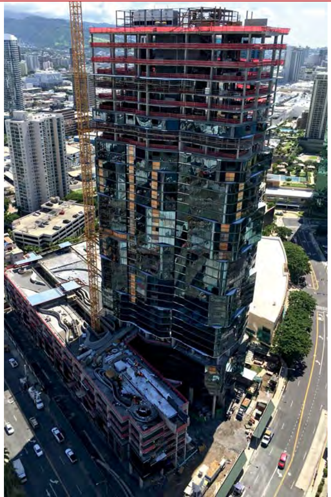
ACK recently wrapped work on Anaha, the latest addition to Ward Village. PHOTO COURTESY ALBERT C. KOBAYASHI INC.
