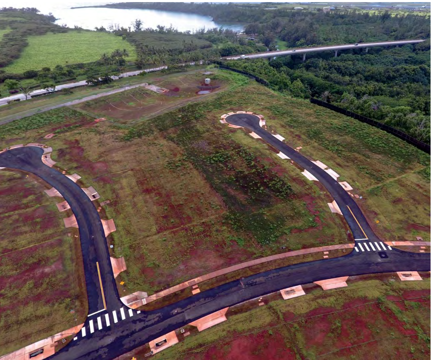
Among the projects Earthworks Pacific recently worked on was the 109-lot residential project Hooluana at Koheo Loa. PHOTOS COURTESY EARTHWORKS PACIFIC INC.
