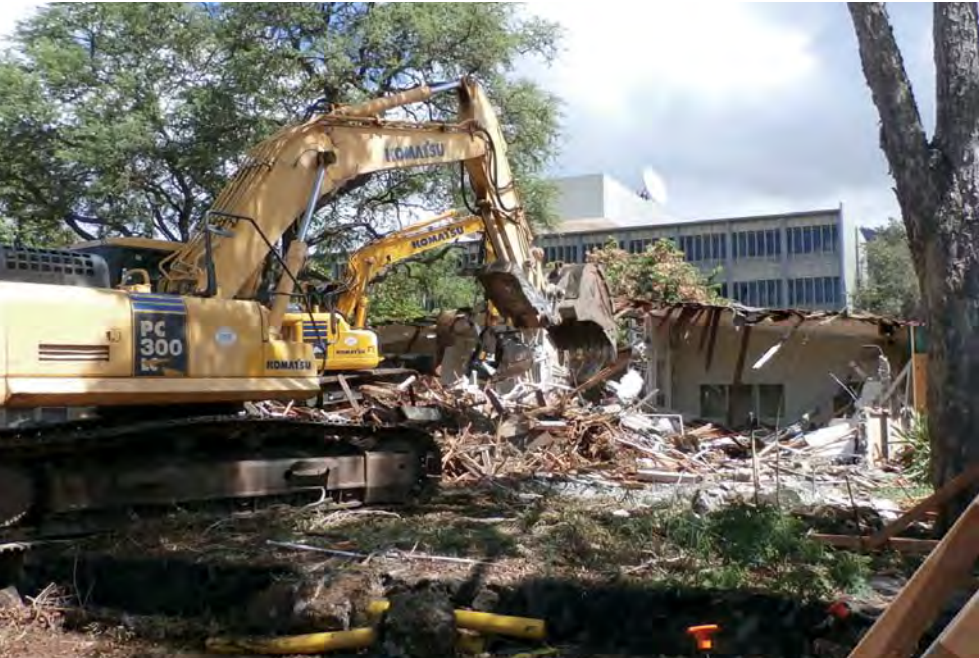
Layton is clearing the site for its build-out of the new University of Hawaii Life Sciences Building. PHOTO COURTESY LAYTON CONSTRUCTION CO. LLC
