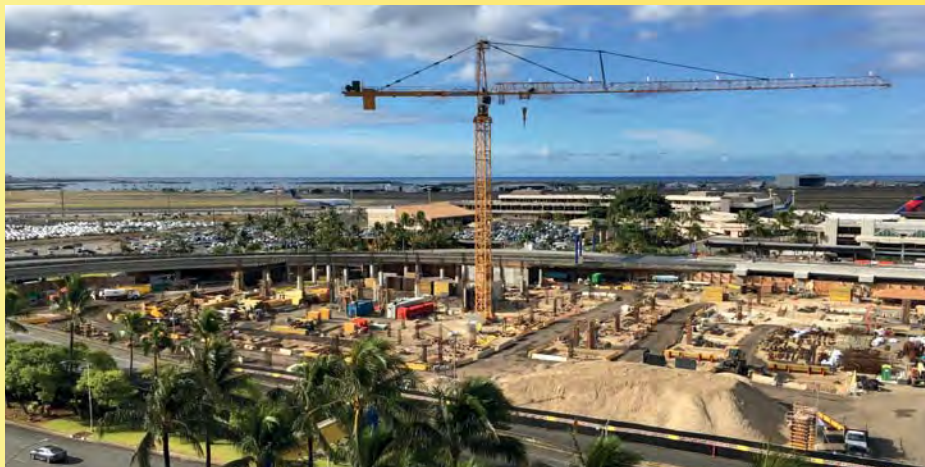
The Daniel K. Inouye International Airport CONRAC is under way by Watts Constructors PHOTO COURTESY WATTS CONSTRUCTORS LLC
