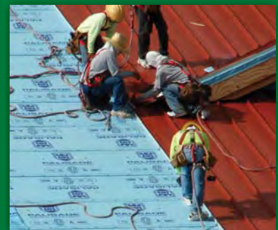
CUSTOM METAL ROOFING
