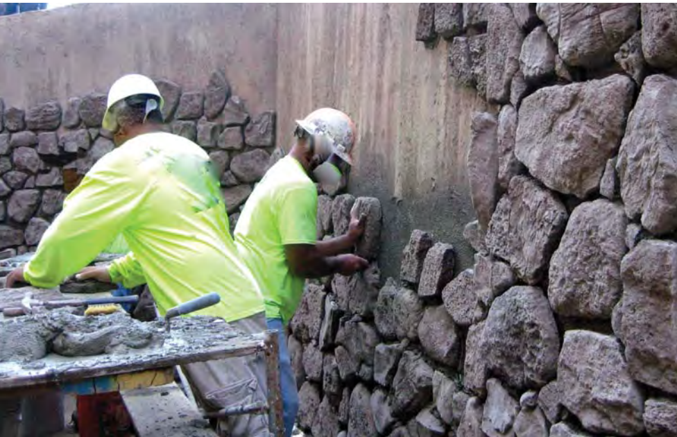
A Big Rock Manufacturing crew adds decorative veneer to a new wall.
