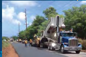
Hansen Road Pavement Reconstruction
