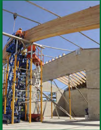
GLULAMS @ KEAUKAHA ELEMENTARY SCHOOL
