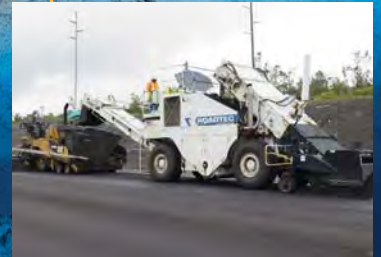
Saddle Road Reconstruction
