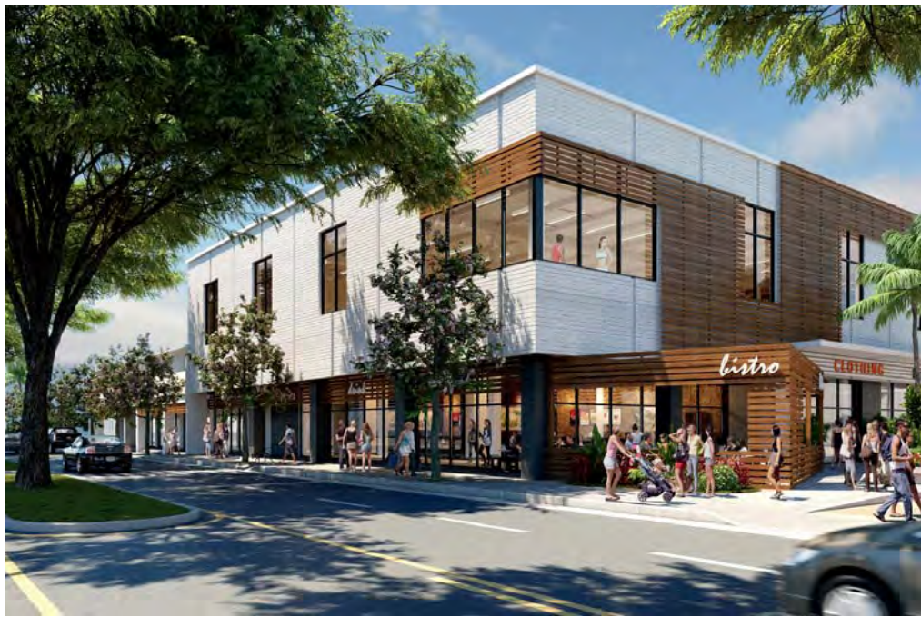
The renovated Lau Hala Shops in Kailua RENDERING COURTESY AHL AND ALEXANDER & BALDWIN
