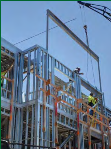
STEEL FRAMING @ KA MALANAI, KAILUA
