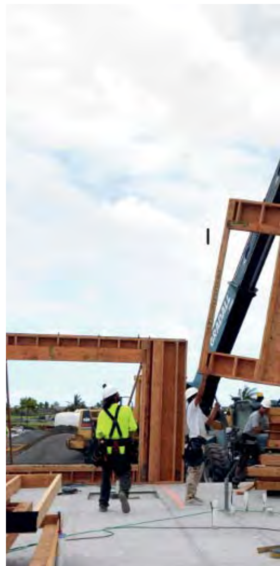
The Kohaniki Hale Project features HPM’s wall panels. PHOTO COURTESY HPM BUILDING SUPPLY
