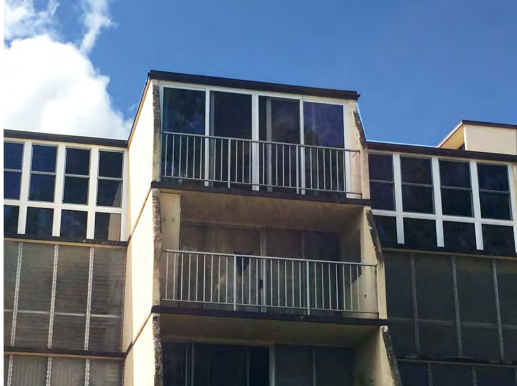
Coastal Windows and Doors is replacing all doors and windows in Mililani's 132-unit Ridgecrest condominium complex.
