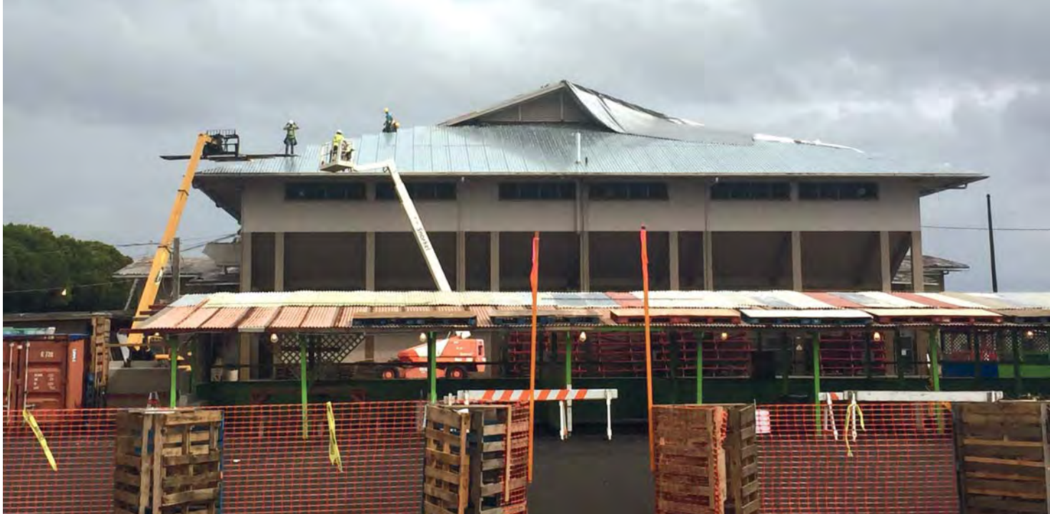
Sterling Pacific Construction recently completed work on the Afook-Chinen Hilo Civic Auditorium. PHOTO COURTESY STERLING PACIFIC CONSTRUCTION
