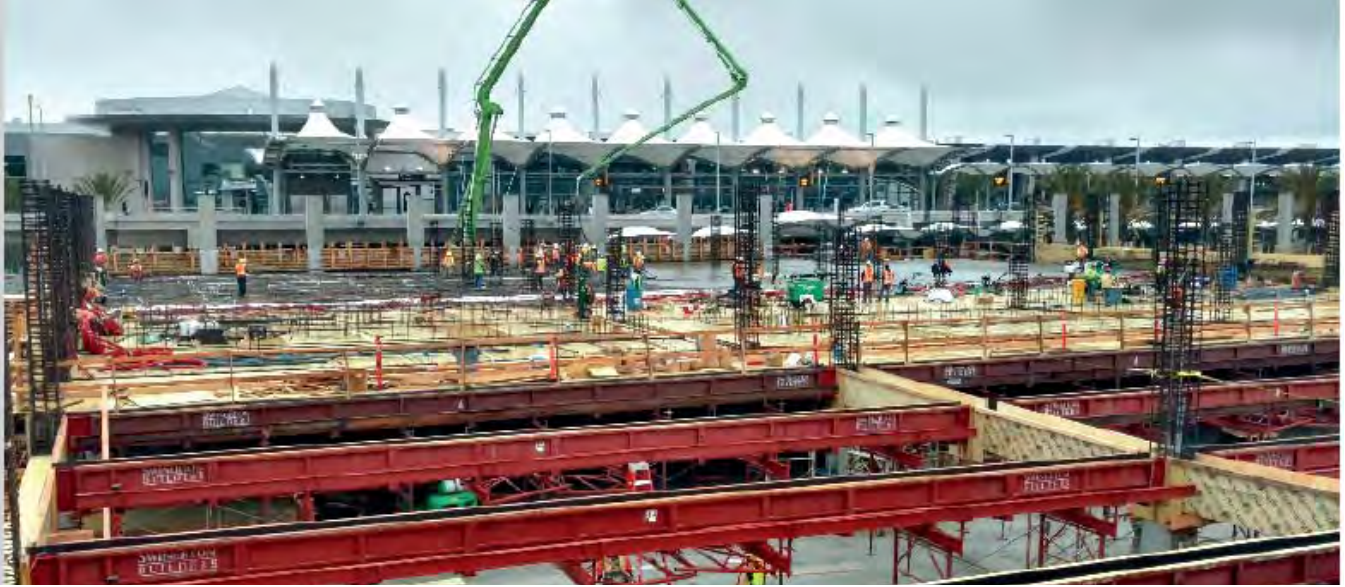
The San Diego Parking Plaza required a three-day compressive strength mix of 2,750 psi. PHOTO COURTESY VAPOR LOCK/SPECIALTY PRODUCTS GROUP
