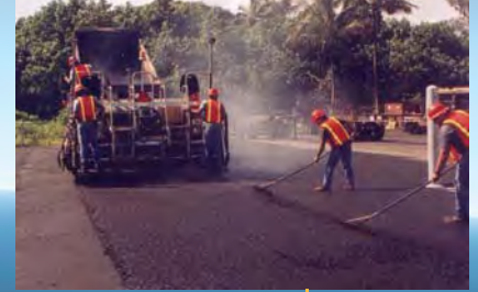
Hilo Harbor Improvements
