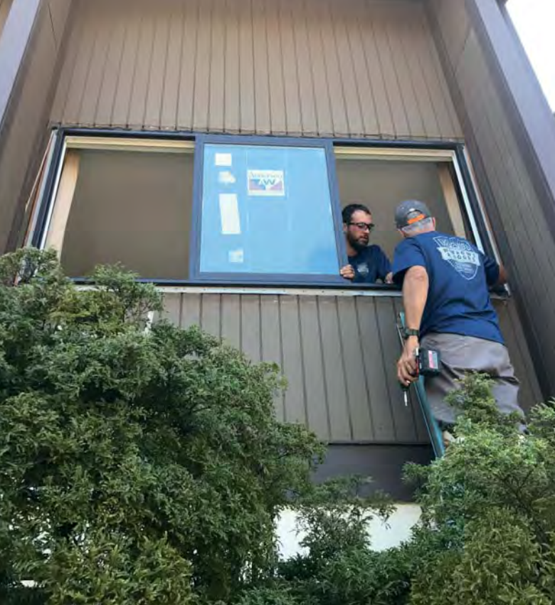
Crews from Maui Windows and Doors install Andersen windows.
