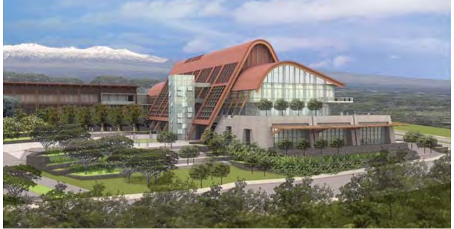
A major project for Isemoto Contracting is work on the University of Hawaii at Hilo’s Daniel K. Inouye College of Pharmacy.
