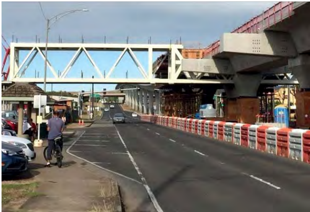
A Hawaiian Dredging Construction Co. crew recently lifted the 197,000-pound pedestrian bridge into position at the site of the rail’s West Loch Station.
