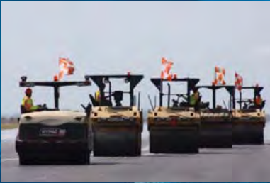
Reef Runway Pavement Improvements
