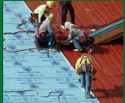
CUSTOM METAL ROOFING
