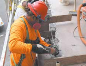
HIGH-RISE SPALL REPAIR
