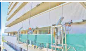
HIGH-RISE SPALL REPAIR
