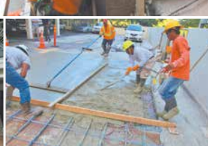
PARKING DECK & PT CABLE REPAIRS
