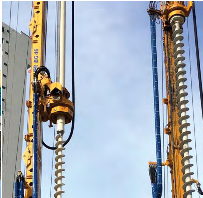
AUGERCAST PILES
