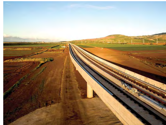
(Top and above) Two views of the rail system using drones. PHOTOS COURTESY KENJI CROMAN PHOTOGRAPHY
