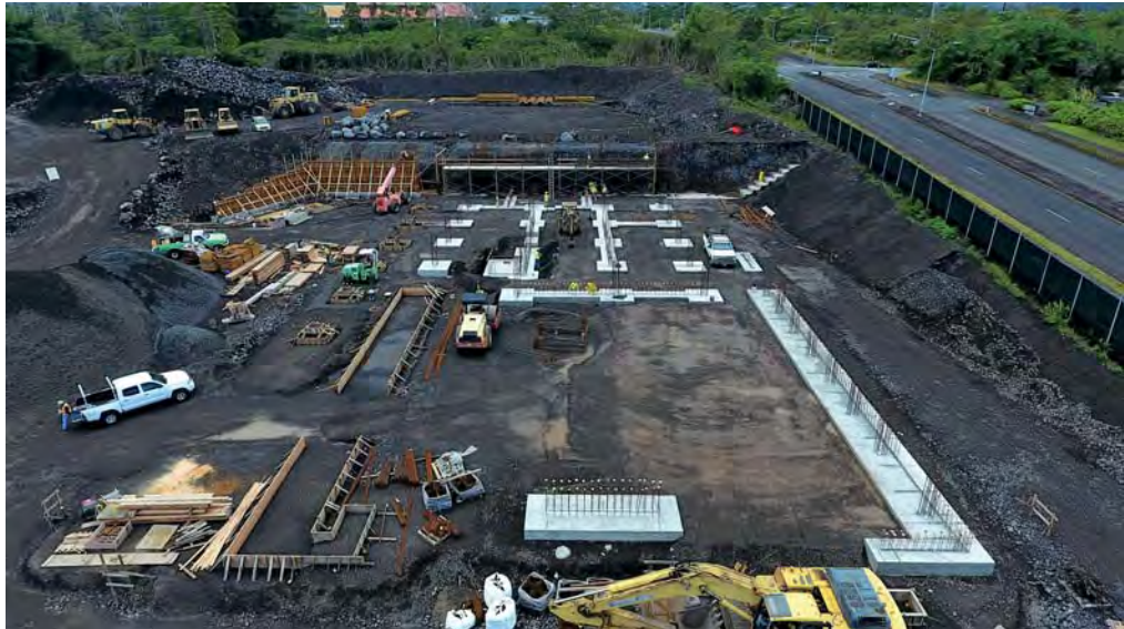
Isemoto Contracting's work continues on the College of Pharmacy building at the University of Hawaii-Hilo.
