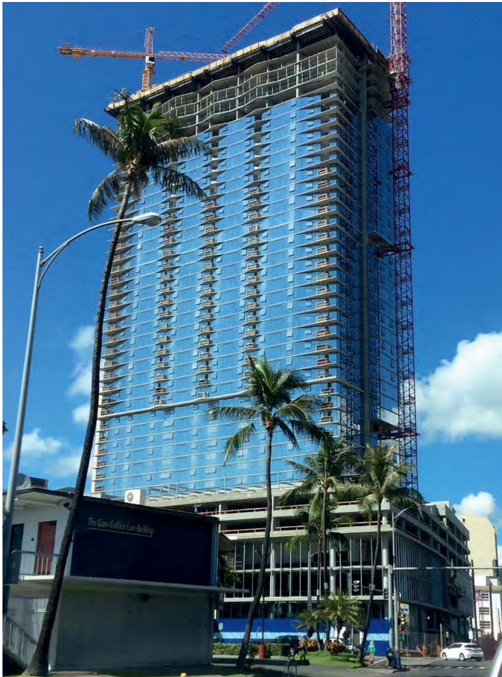
Dorvin D. Leis Inc, completed its work on OM Symphony Honolulu last year.
