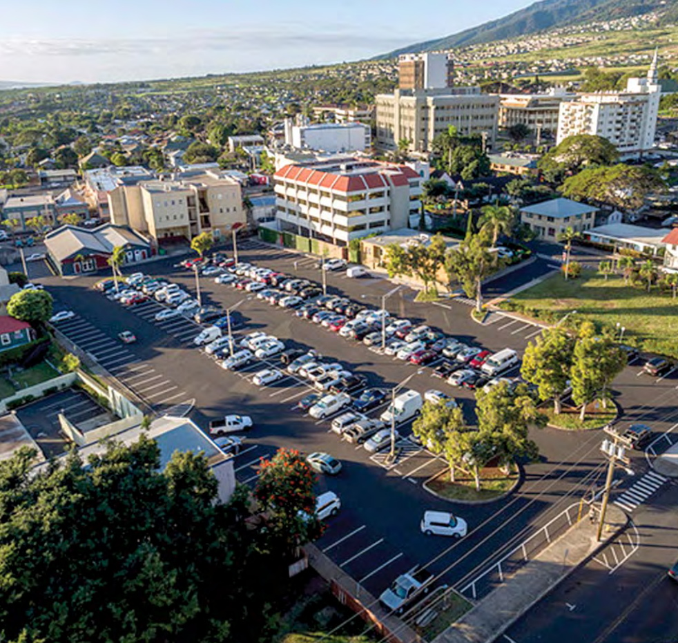
A drone view of a proposed parking structure in Wailuku, Maui PHOTO COURTESY ANDREA BRIZZI PHOTOGRAPHY LLC
