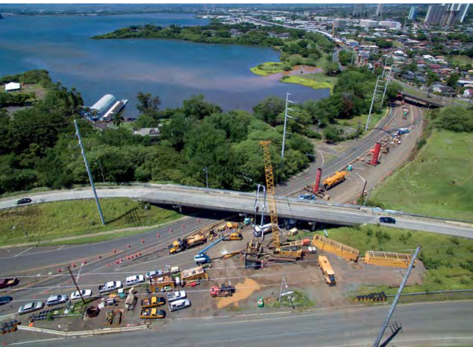
Kiewit completes the final shaft pour at the guideway along Kamehameha Highway.
