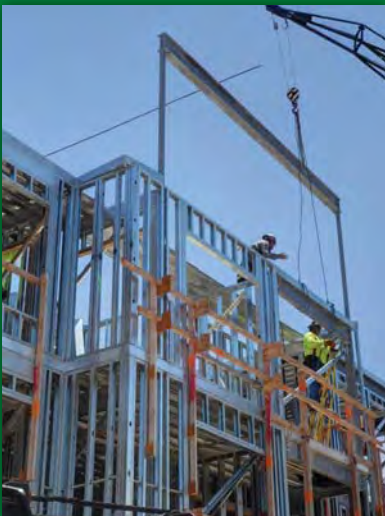
STEEL FRAMING @ KA MALANAI, KAILUA
