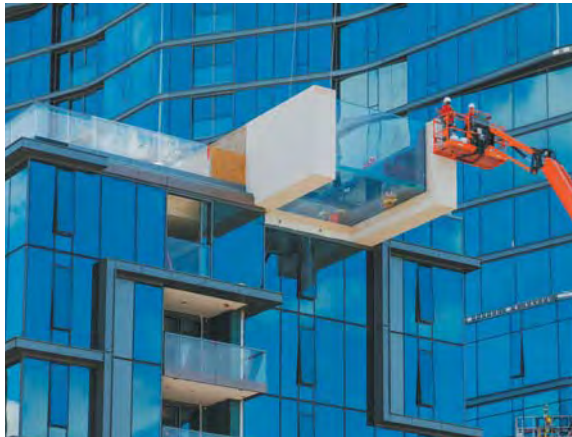
A glass-bottomed pool at Anaha juts out 16 feet from the building. The pool is being built Pacific Aquascapes. PHOTO COURTESY THE HOWARD HUGHES CORPORATION
