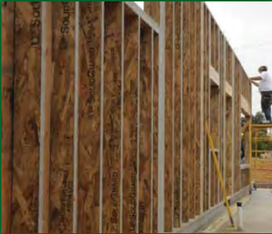
LSL WALL PANELS @ HOSPICE, KAMUELA
