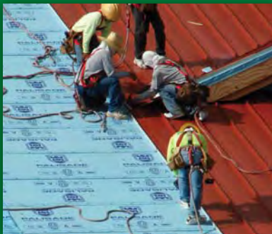
CUSTOM METAL ROOFING
