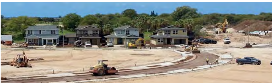
Paradigm Construction wrapped up work at Ewa By Gentry Area 17 last year.
