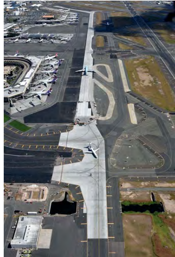
Kiewit projects last year included Taxiway Z at Honolulu International Airport.
