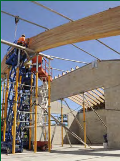
GLULAMS @ KEAUKAHA ELEMENTARY SCHOOL
