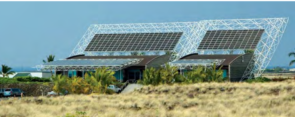
Hawaii Gateway Energy Center
