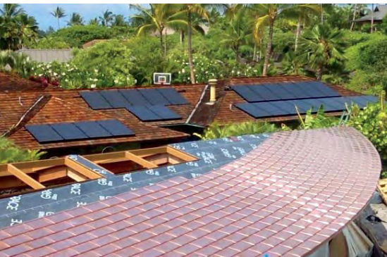
Kokua Roofing installed a copper shingle roof on a custom home in Kukio, Kailua-Kona.
