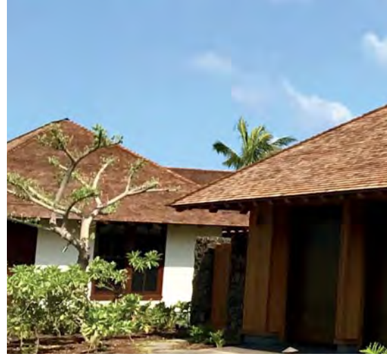
Cedar shake shingles, Kohanaiki, Kailua-Kona. PHOTO COURTESY OF KOKUA ROOFING
