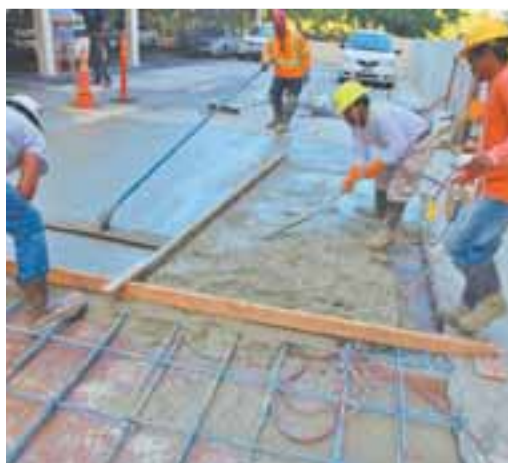
PARKING DECK & PT CABLE REPAIRS
