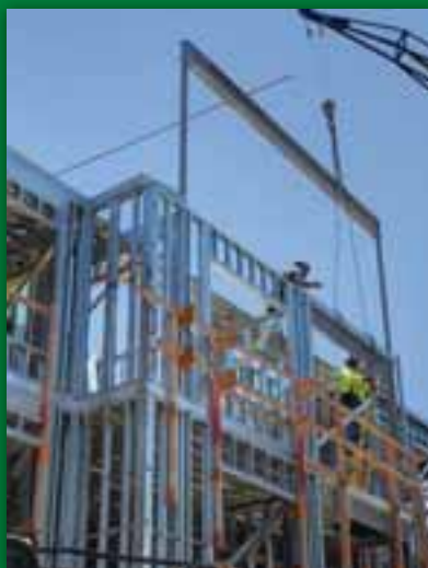
STEEL FRAMING @ KA MALANAI, KAILUA
