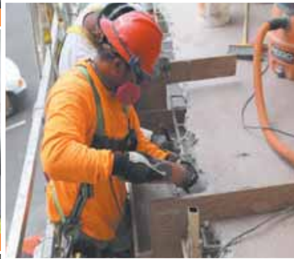
HIGH-RISE SPALL REPAIR
