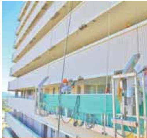
HIGH-RISE SPALL REPAIR
