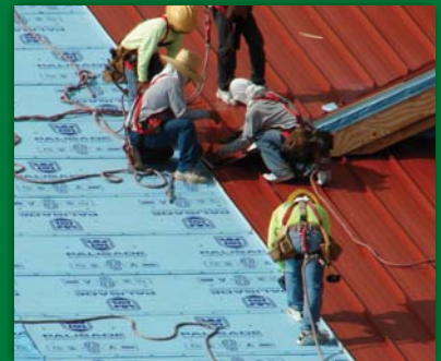
CUSTOM METAL ROOFING
