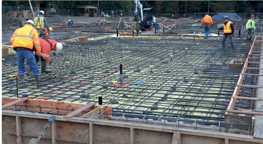
Stego's Beast Screed System being used at a construction project.
