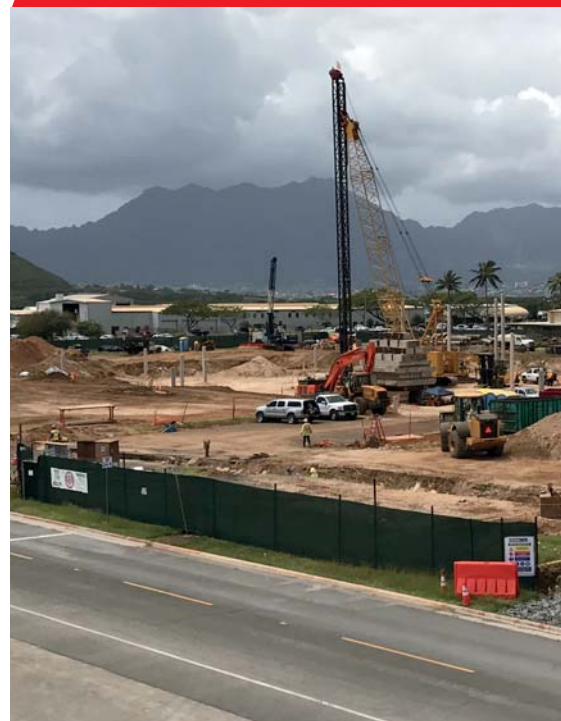
After foundation load test, Caddell-Nan JV executes pile driving operations at the new MCBH Medical/Dental Clinic in March.
