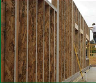
LSL WALL PANELS @ HOSPICE, KAMUELA
