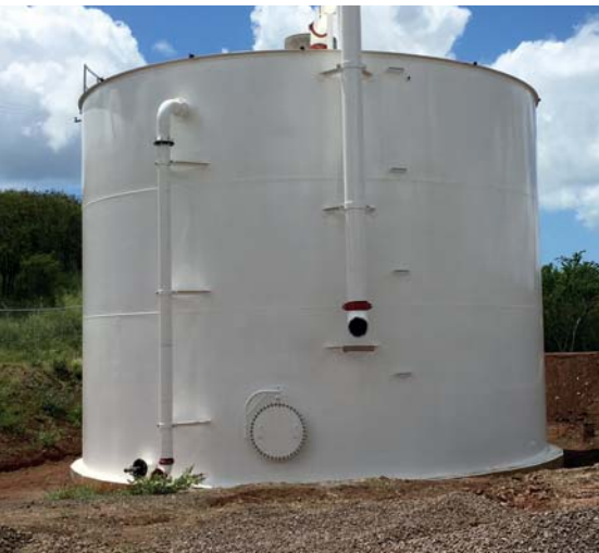
Hensel Phelps completed a 125,000-gallon retention tank for the collection and disposal of Aqueous Film Forming Foam (AFFF) at the Navy Red Hill Fuel Tank Facility. PHOTO COURTESY ANTHONY KLUTZ/HENSEL PHELPS
