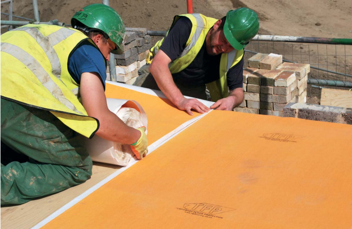
Workers installing a Skudo Tack-Mat.
