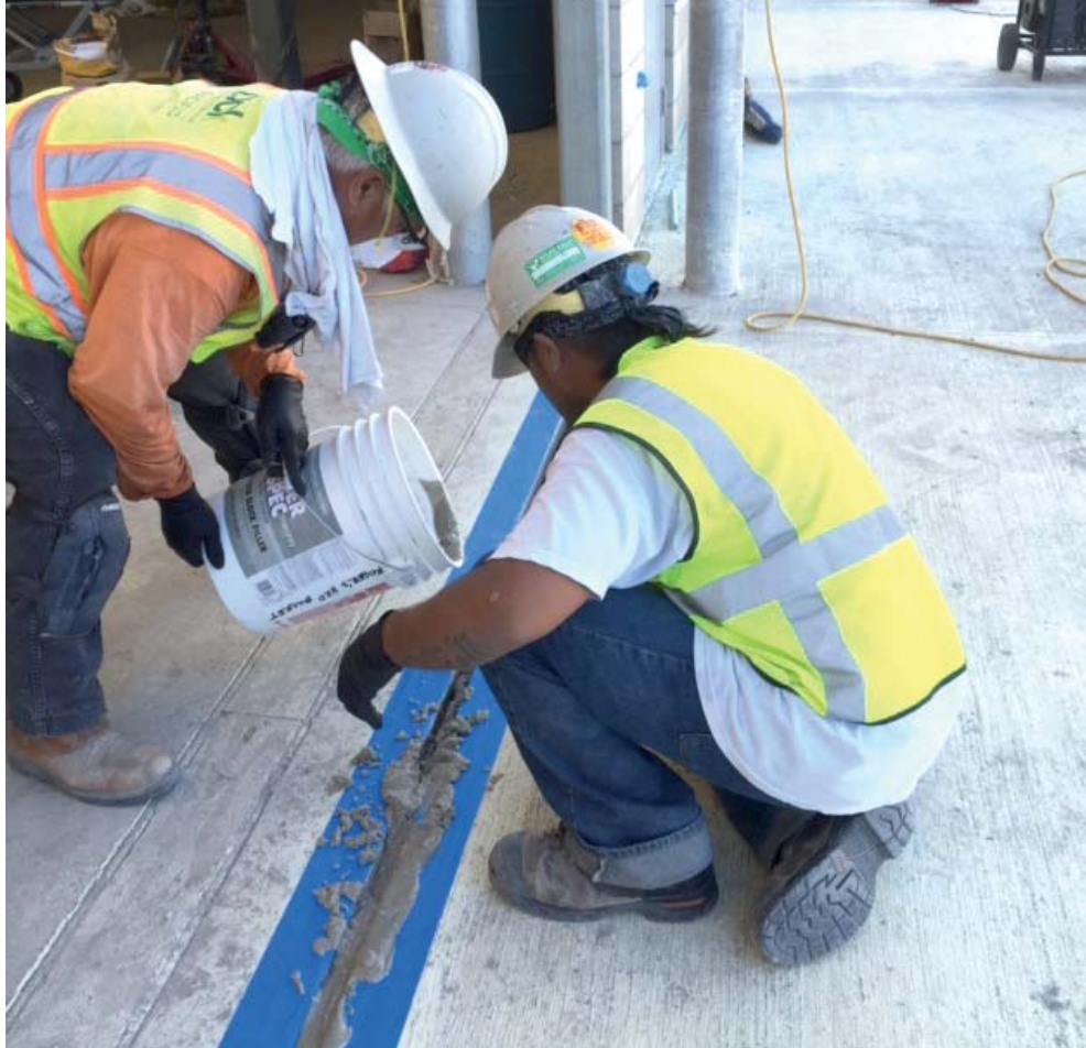
Workers apply material to bond concrete slabs together.
