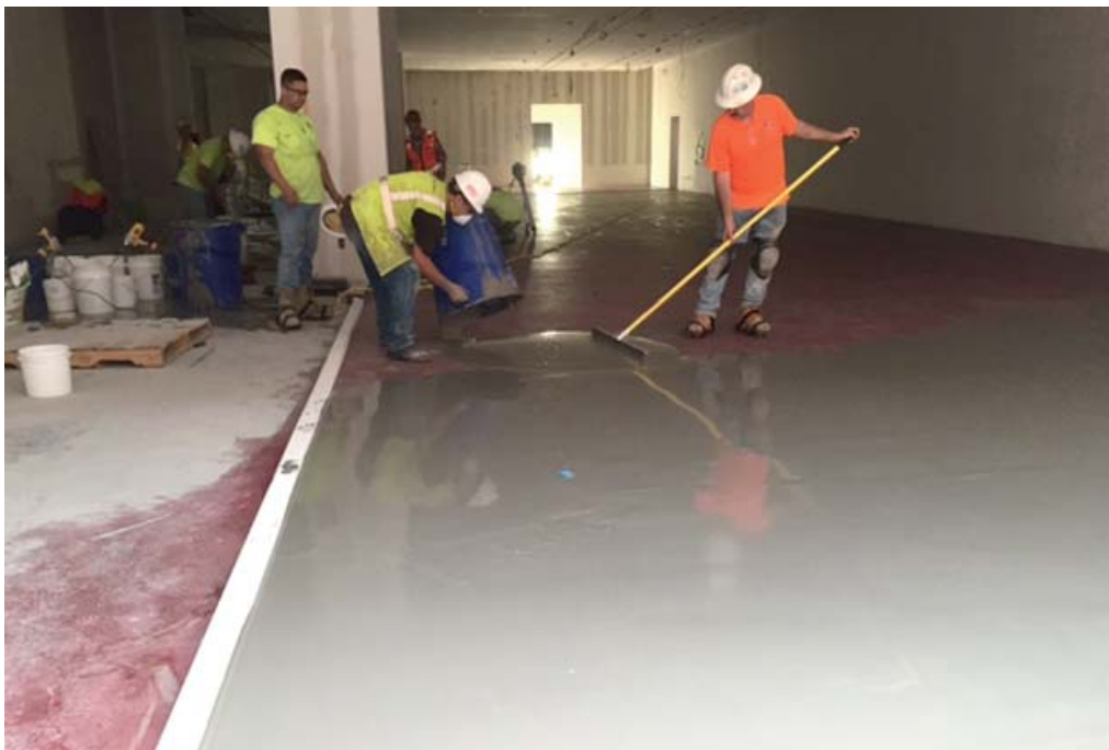
A surface protection is applied to a concrete slab flooring.
