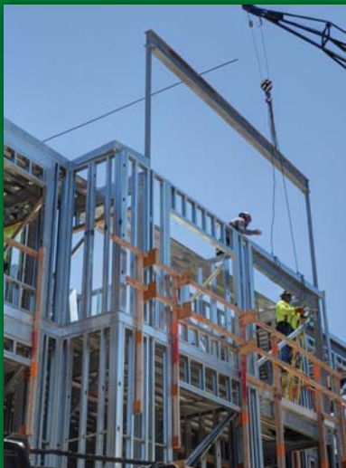
STEEL FRAMING @ KA MALANAI, KAILUA
