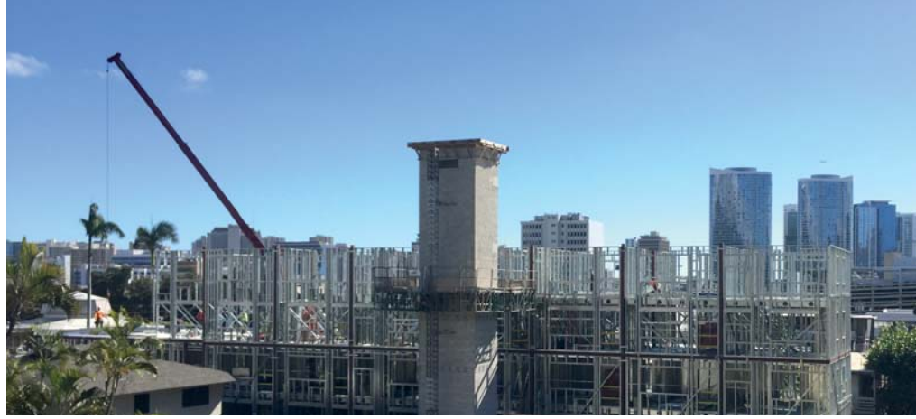
The Residence at Makiki: five-story light gauge metal framing with red iron post and distribution members
