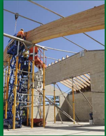
GLULAMS @ KEAUKAHA ELEMENTARY SCHOOL
