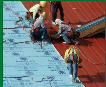
CUSTOM METAL ROOFING
