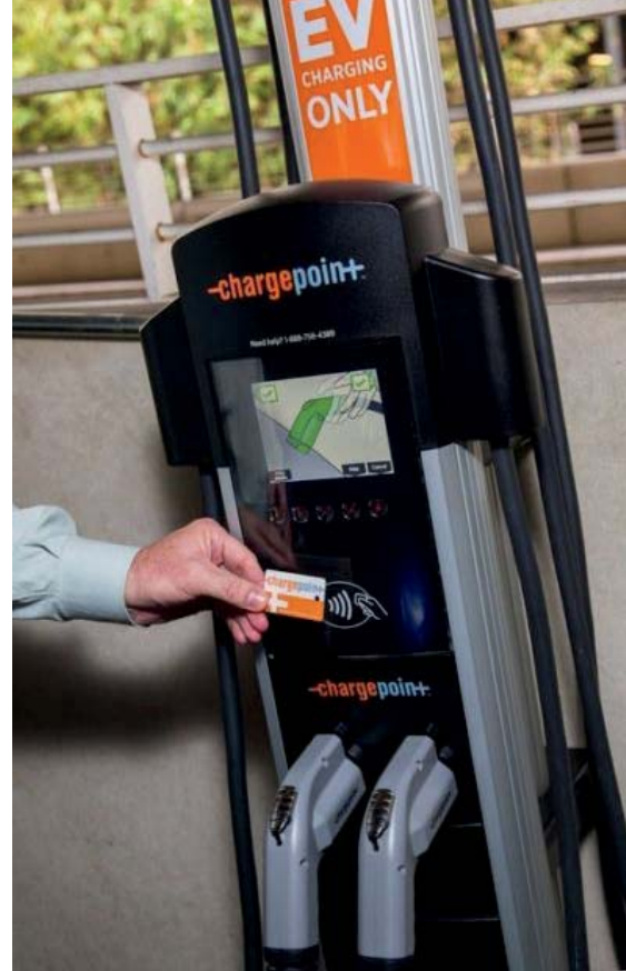
A customer uses a Charge Point EV charging station.
