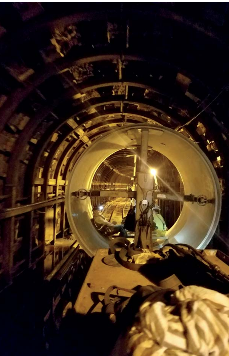
A tunnel pipe being transported as part of the KK Tunnel Project
