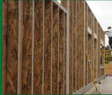
LSL WALL PANELS @ HOSPICE, KAMUELA
