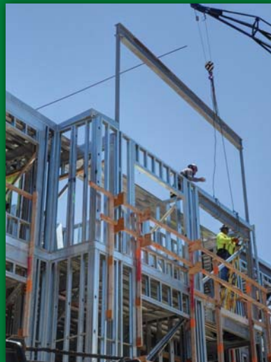
STEEL FRAMING @ KA MALANAI, KAILUA
