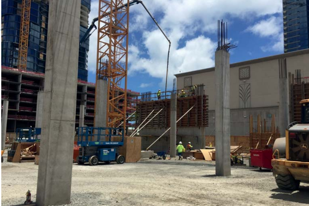
At the Aeo tower with Layton Construction as GC, W.W. Clyde is placing concrete from the footings to the top (42nd) floor.
