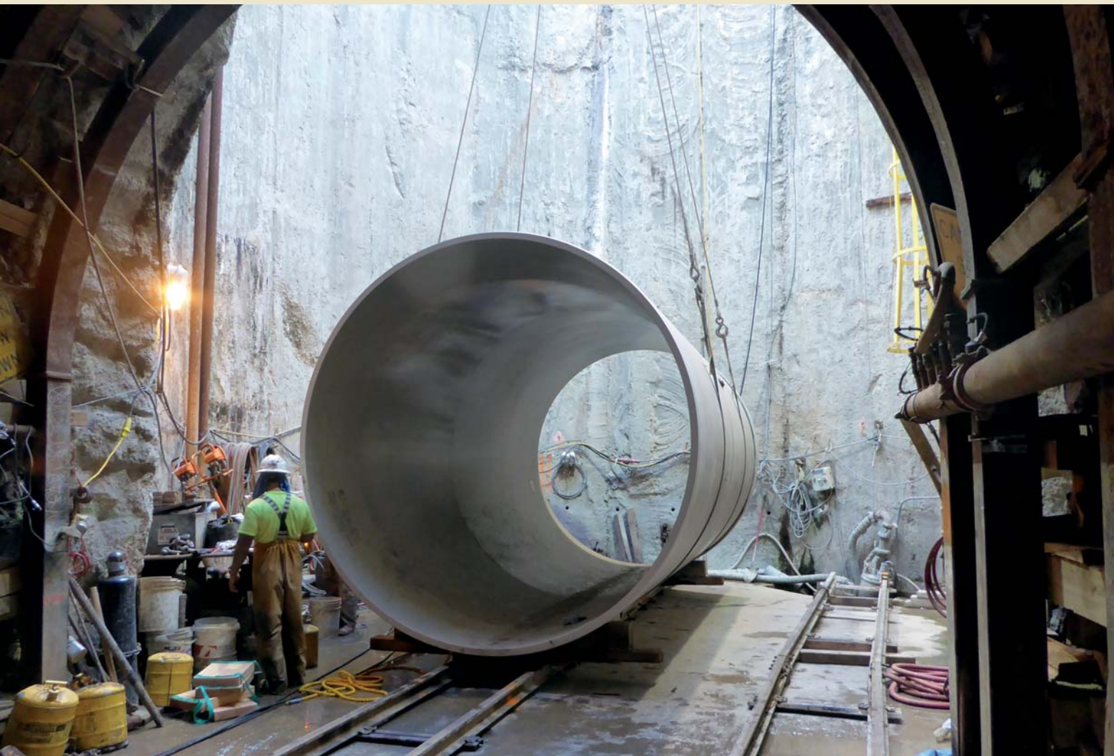
A 20-foot staging pipe, part of the KK Tunnel Project
