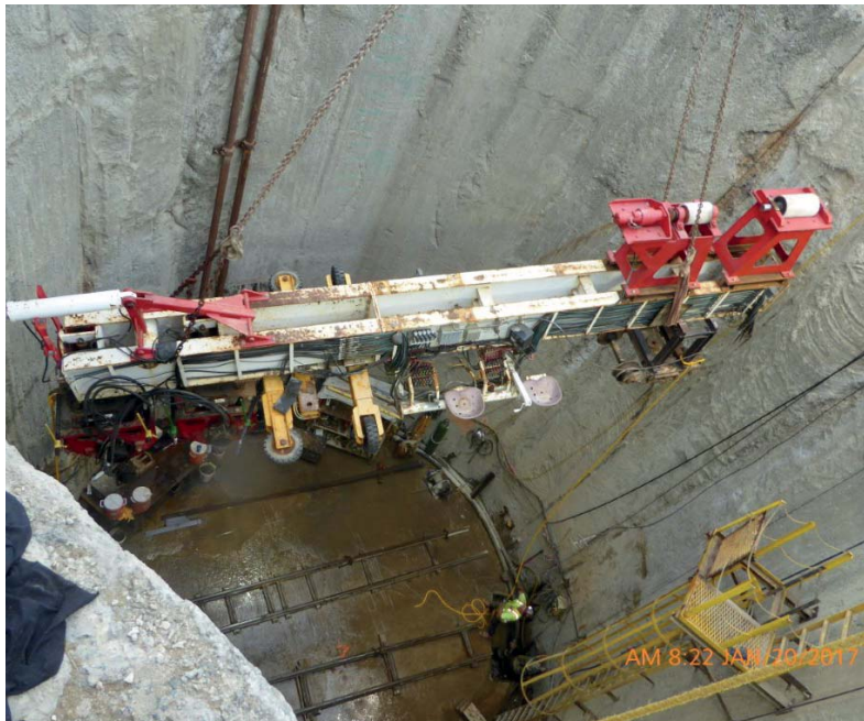
A pipe is lowered into the shaft of the KK Tunnel Project.
