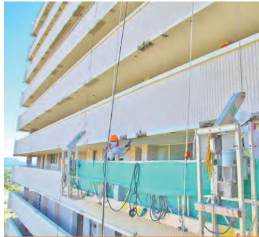
HIGH-RISE SPALL REPAIR
