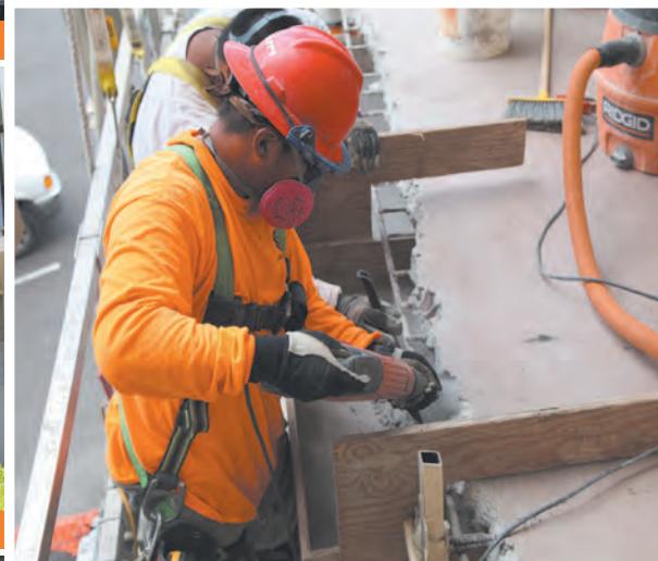
HIGH-RISE SPALL REPAIR
