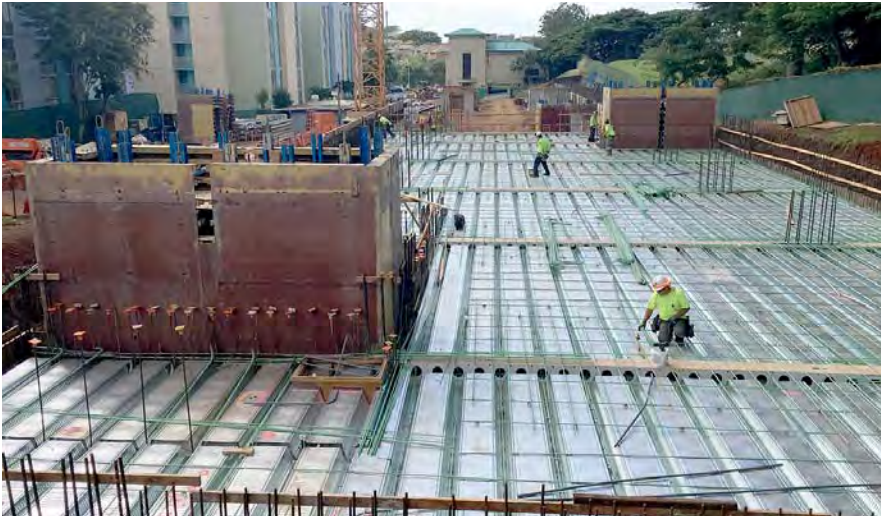
Work continues at Moanalua Hillside Apartments
