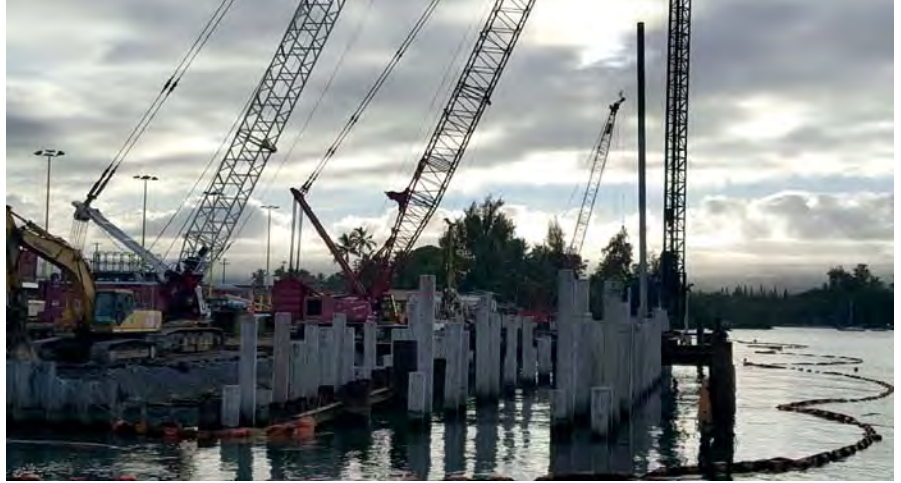
Healy Tibbitts job at Pier 4 requires the use of multiple crane booms, piles and pile leads.
