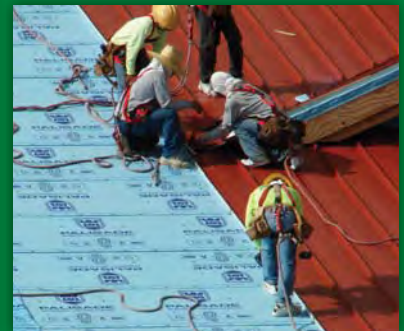
CUSTOM METAL ROOFING
