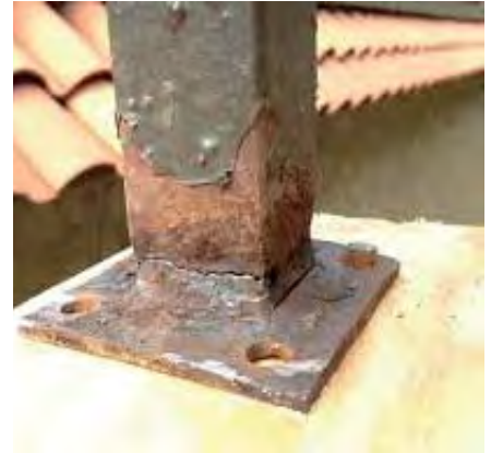
Metal also must be waterproofed.
