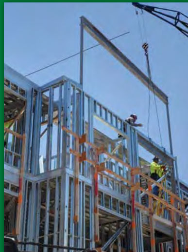
STEEL FRAMING @ KA MALANAI, KAILUA
