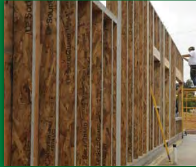
LSL WALL PANELS @ HOSPICE, KAMUELA
