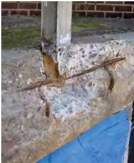
Spalling in concrete must be repaired
