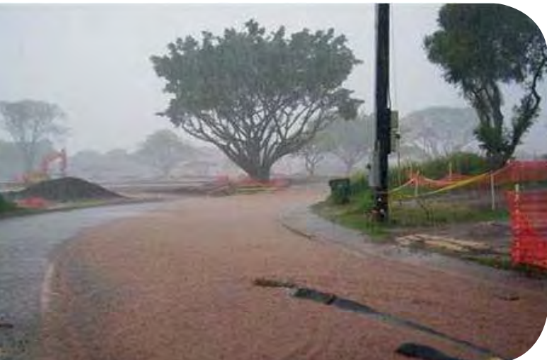
Large graded areas during a downpour. PHOTO COURTESY RUSSELL LEONG
