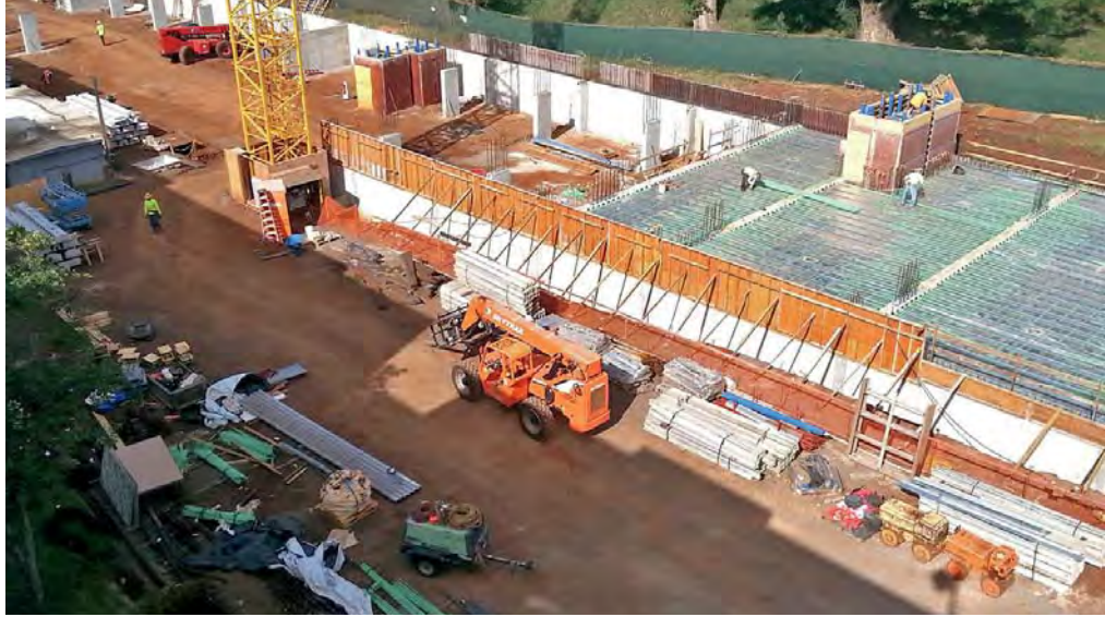
King & Neel Inc. is providing surety services for the ongoing Moanalua Hillside Apartments. Unlimited Construction Services Inc. is the general contractor.
