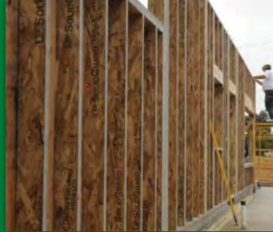
LSL WALL PANELS @ HOSPICE, KAMUELA
