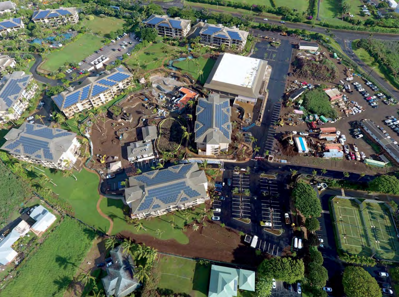
Layton Construction's Koloa Landing Phase III on Poipu Beach PHOTO COURTESY LAYTON CONSTRUCTION CO. LLC
