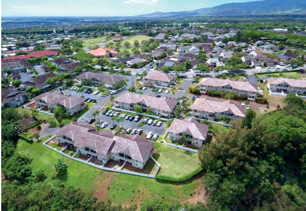
Commercial Roofing & Waterproofing installed shake roofs at Cliffside Villages.
