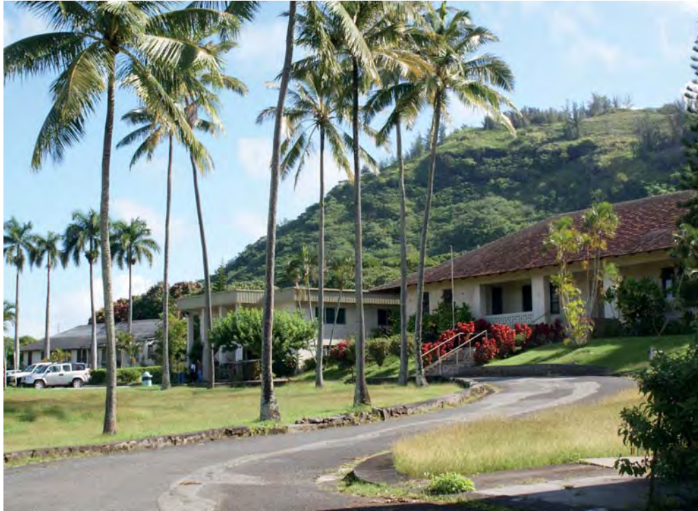
Former convalescent home to be renovated for 32 female adolescent residents.
