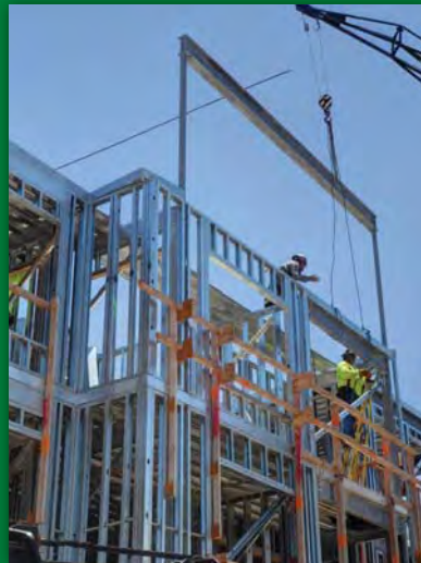
STEEL FRAMING @ KA MALANAI, KAILUA
