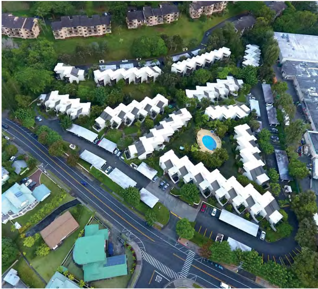
Commercial Roofing & Waterproofing installed roofing at Puu Alii II condominiums.
