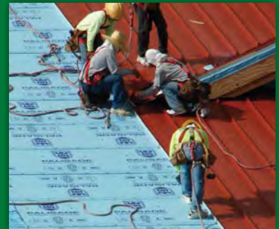
CUSTOM METAL ROOFING
