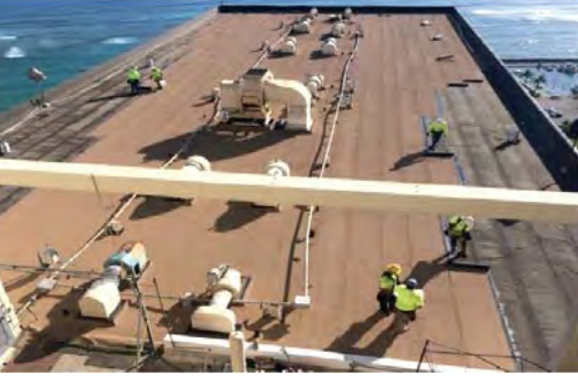
Honolulu Roofing won a first-place RCAH Award for its work at Hilton Hawaiian Village.
