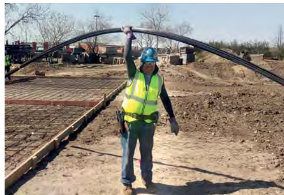
GatorBar is seven times lighter than steel, according to Neuvokas Corp.
