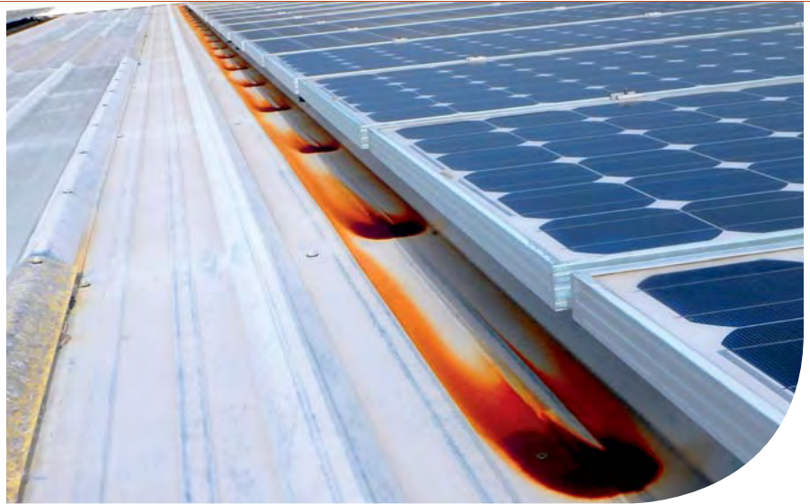
Cleaning away rust and corrosion can restore the PV system to full power.
