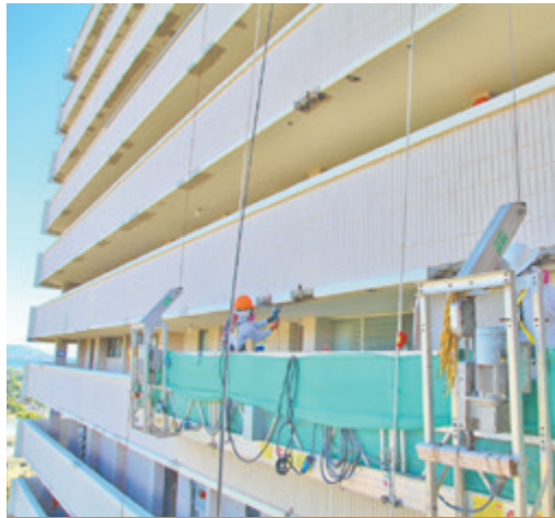
HIGH-RISE SPALL REPAIR
