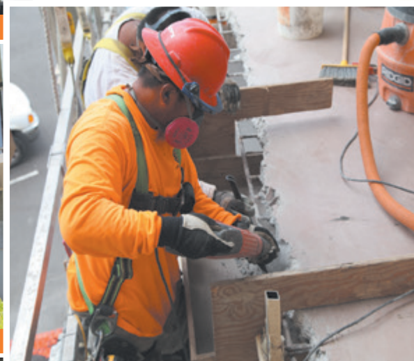
HIGH-RISE SPALL REPAIR
