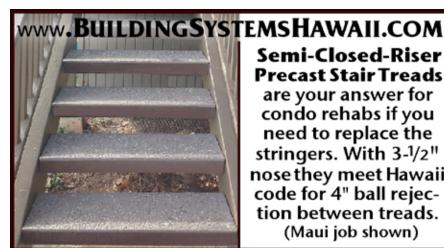
Semi-Closed-Riser Precast Stair Treads are your answer for condo rehabs if you need to replace the stringers. With 3-1/2" nose they meet Hawaii code for 4" ball rejection between treads. (Maui job shown)
