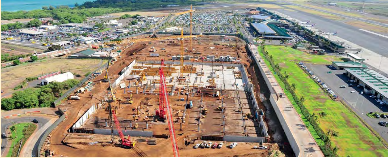
Hawaiian Dredging is GC on the Kahului Airport ConRAC. PHOTO COURTESY HAWAIIAN DREDGING
