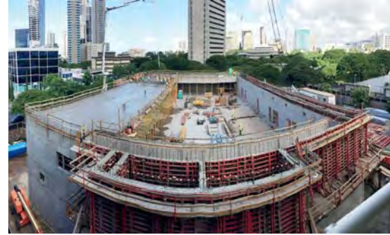
Joint Traffic Management Center PHOTO COURTESY OF WATTS CONSTRUCTORS
