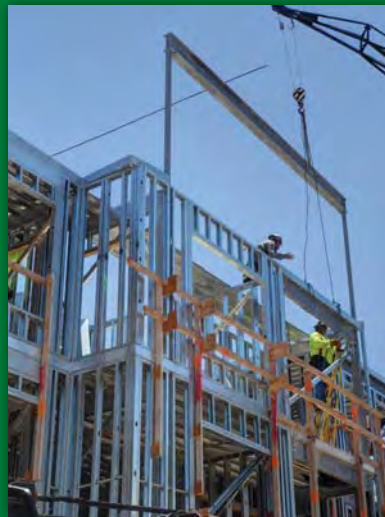
STEEL FRAMING @ KA MALANAI, KAILUA
