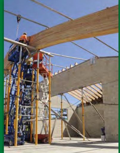
GLULAMS @ KEAUKAHA ELEMENTARY SCHOOL
