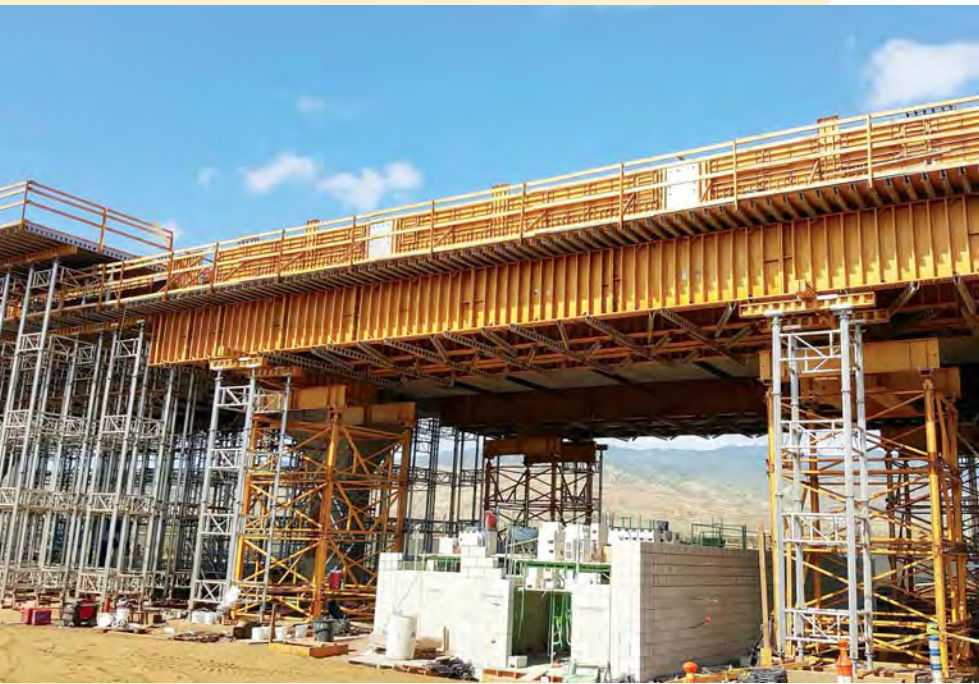
HART Hoopili station TCCR building with shoring PHOTO COURTESY JUSTIN BARFIELD/NAN INC.
