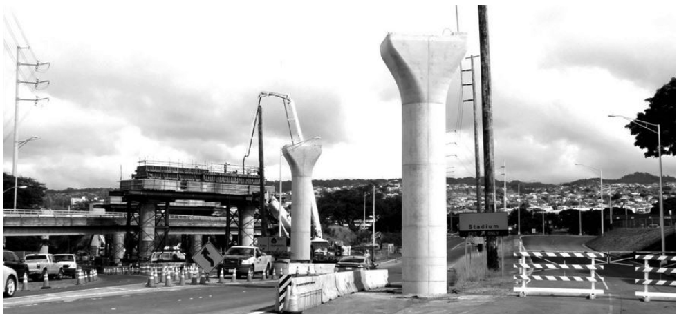
Kiewit crews work on the guideway over Kamehameha Highway. The final column of the first 10 miles of the 20-mile guideway is between the westbound Kamehameha Highway ramp to Moanalua Freeway and the Aloha Stadium entrance ramp.
