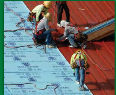
CUSTOM METAL ROOFING
