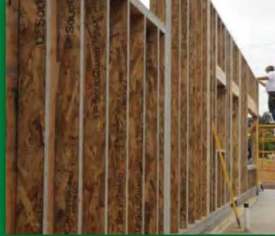
LSL WALL PANELS @ HOSPICE, KAMUELA
