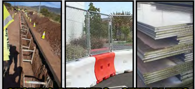
SHORING, BARRIERS & STEEL PLATES
