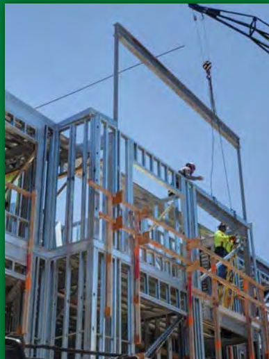
STEEL FRAMING @ KA MALANAI, KAILUA
