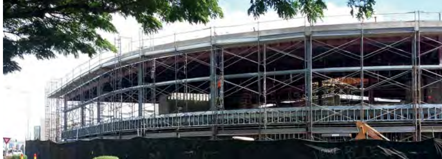
Steel superstructure encasing the original concrete shell PHOTO COURTESY ALLIED BUILDERS SYSTEM
