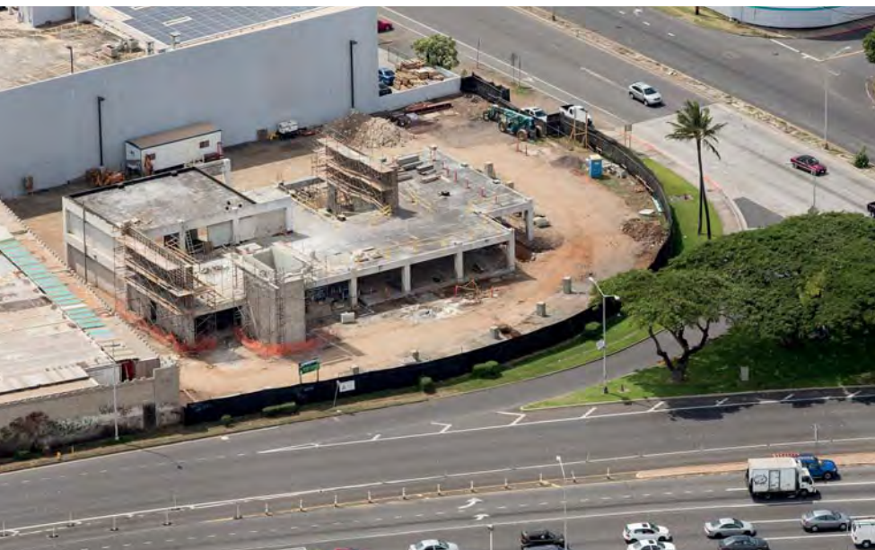
Jobsite on Nimitz Highway and Sand Island Access Road PHOTO COURTESY PBS HAWAII
