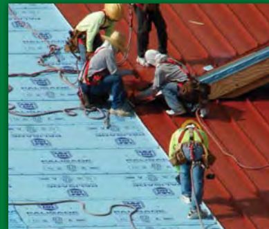
CUSTOM METAL ROOFING
