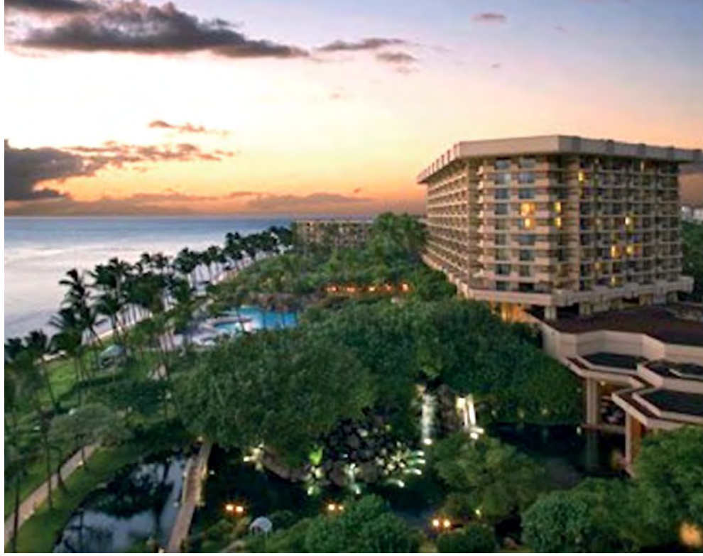
Hyatt Regency Maui Resort & Spa with Swinerton Builders as general contractor
