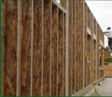
LSL WALL PANELS @ HOSPICE, KAMUELA
