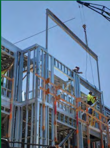
STEEL FRAMING @ KA MALANAI, KAILUA
