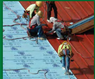
CUSTOM METAL ROOFING
