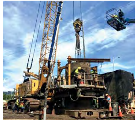
Closing up the cantilever over the H-1 (top) and pouring concrete for the Aloha Stadium drilled shafts. PHOTOS COURTESY HART
