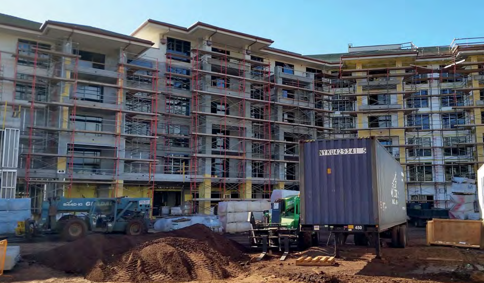
Dorvin D. Leis Co. Inc. provides full mechanical services working with general contractor Hawaiian Dredging on the Kaanapali Ocean Resort, Lot 3. PHOTO COURTESY DORVIN D. LEIS CO. INC.
