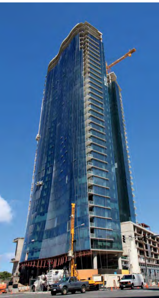
Nordic PCL raises Waiea's curving glass curtain wall.
