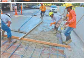
PARKING DECK & PT CABLE REPAIRS
