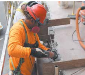
HIGH-RISE SPALL REPAIR
