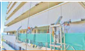
HIGH-RISE SPALL REPAIR
