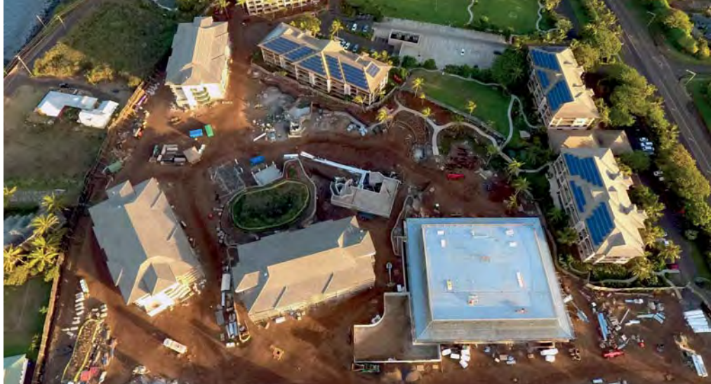
Koloa Landing Phase Three by Layton Construction Co. PHOTO COURTESY LAYTON CONSTRUCTION CO.
