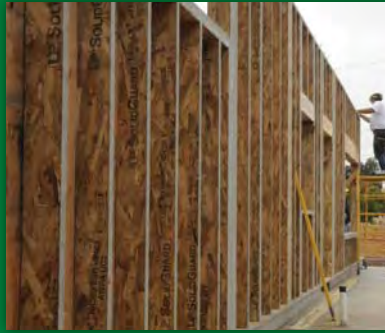
ISL WALL PANELS @ HOSPICE, KAMUELA
