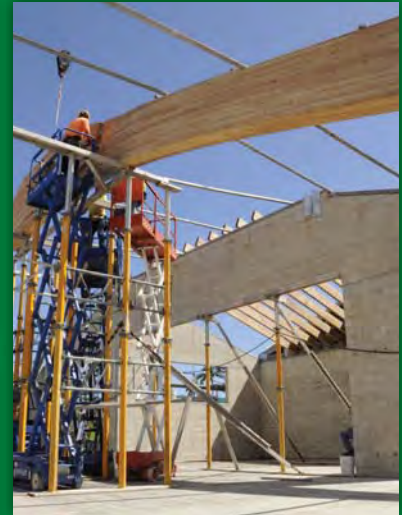
GLULAMS @ KEAUKAHA ELEMENTARY SCHOOL
