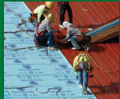
CUSTOM METAL ROOFING
