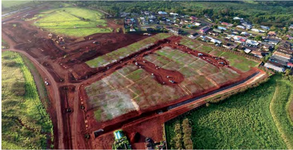
Earthworks Pacific Inc. grades the site of D.R. Horton-Hawaii Division's Hooluana at Kohea Loa neighborhood. PHOTO COURTESY EARTHWORKS PACIFIC INC.
