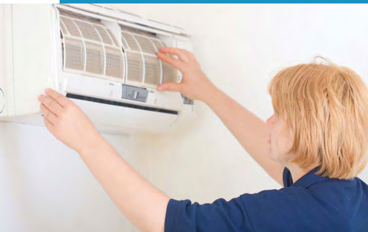
An air conditioner's filters and coils accumulate dust and dirt that affect its efficiency. PHOTO COURTESY ENERGY.GOV
