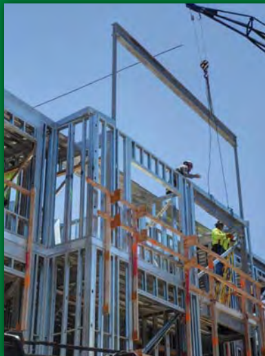
STEEL FRAMING @ KA MALANAI, KAILUA
