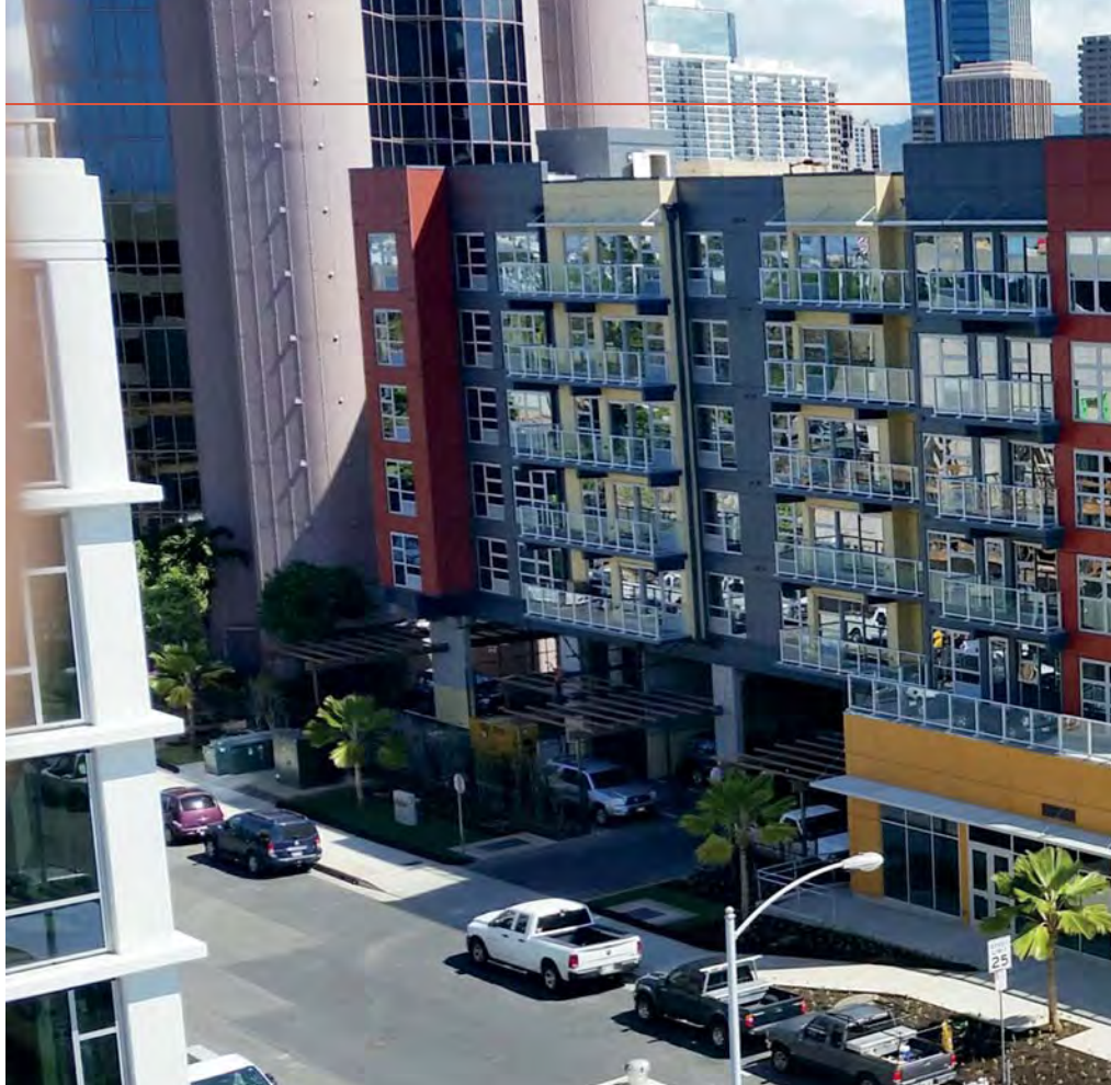
Exterior view of Hawaiian Dredging's 400 Keawe St. project
