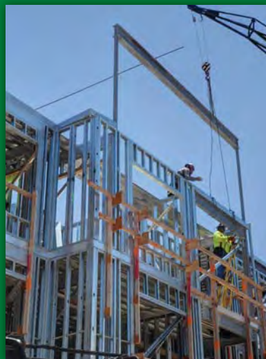
STEEL FRAMING @ KA MALANAI, KAILUA
