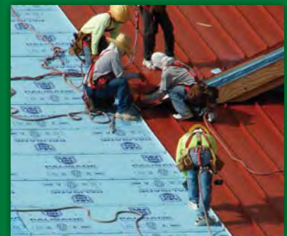
CUSTOM METAL ROOFING
