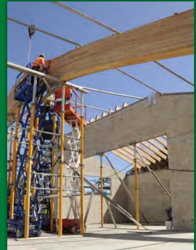
GLULAMS @ KEAUKAHA ELEMENTARY SCHOOL
