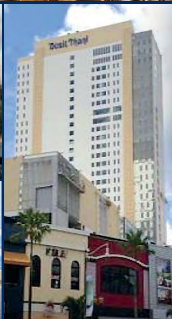
Waikiki Trade Center Renovations
