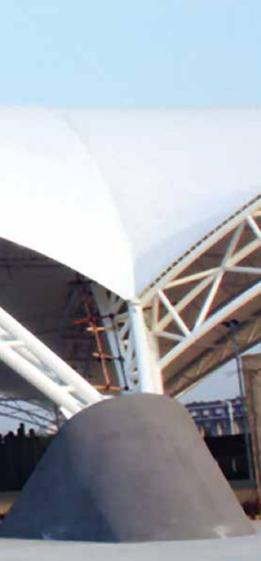
Tensile membrane structures can cover large areas while providing an attractive appearance.
