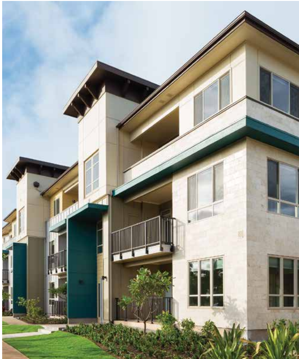
The Kapolei Lofts community, designed by KTG Architecture + Planning, is a four-block series of three-story walk-up apartment buildings and neighborhood gathering places.
