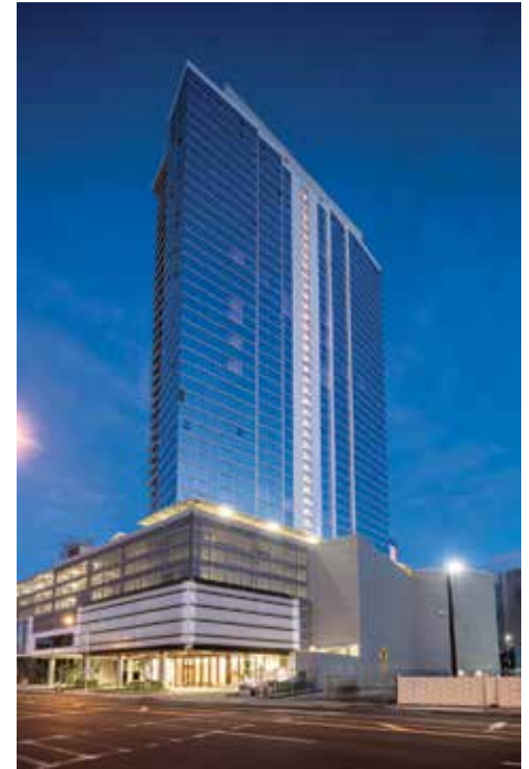
Symphony Honolulu is a beautiful new high-rise building, home to 388 private condominium residences with sweeping mountain and ocean views.
