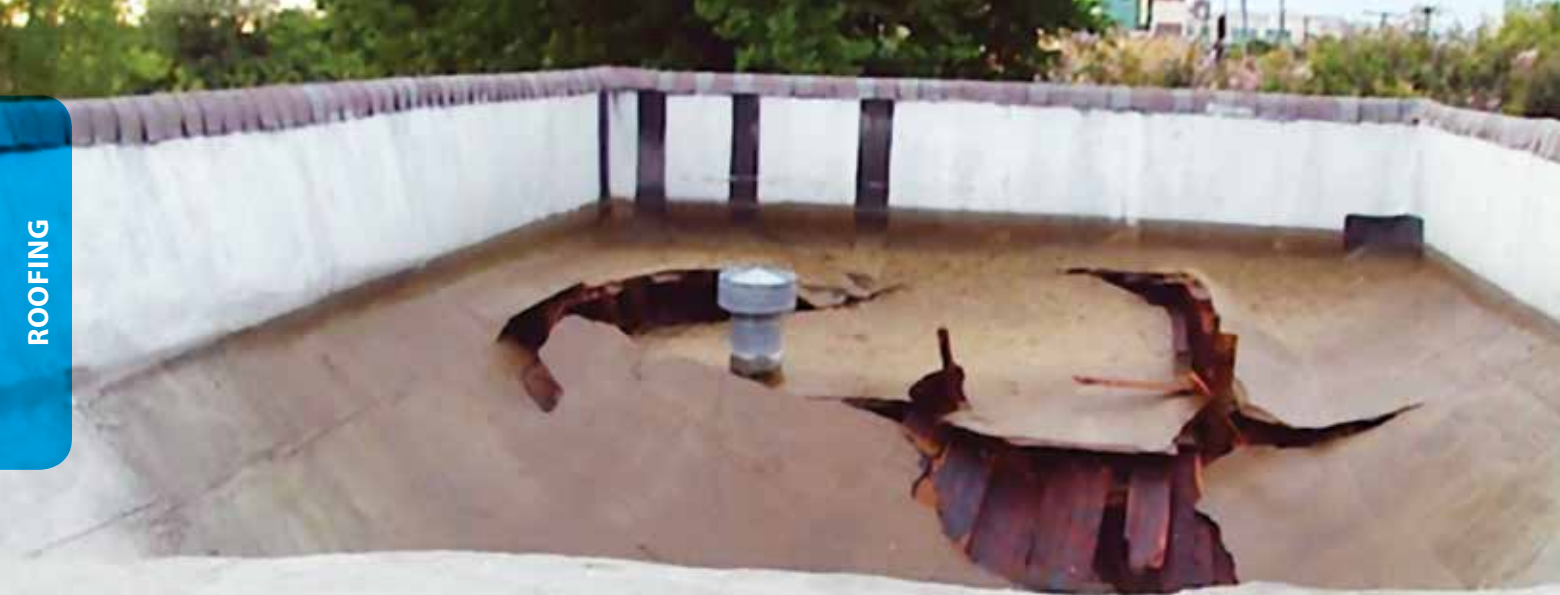
A collapsed roof due to water weight.
